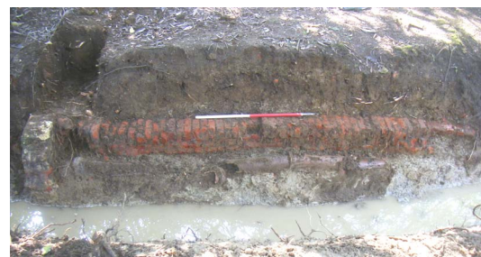
Culvert and headwall in Area 29. Scale 1m
