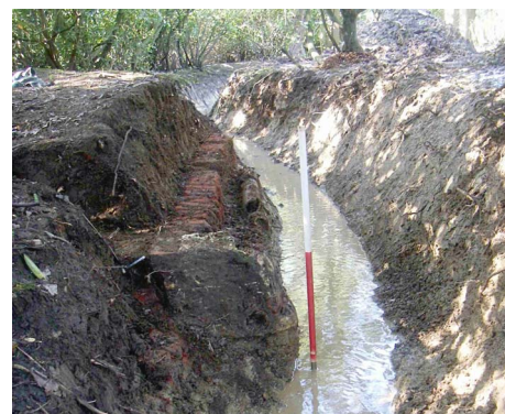
Culvert and headwall in Area 29. Scale 1m
