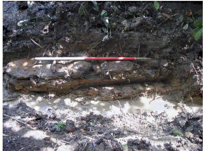
Culvert 2052 in Area 31. Scale 1m
