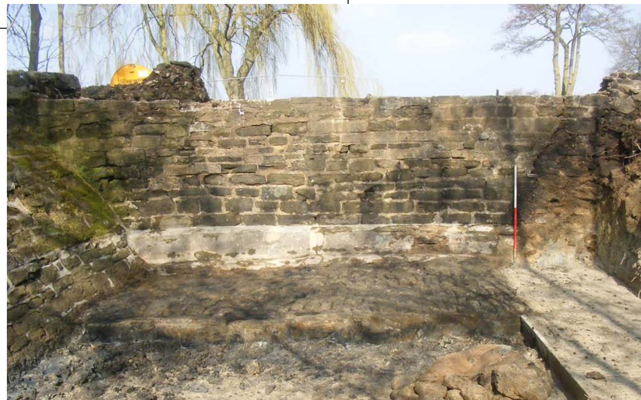
Stones at base of weir. Looking north. Scale 1m
