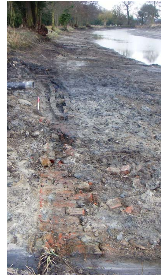
Culvert (1081), looking south. Scale 1m
