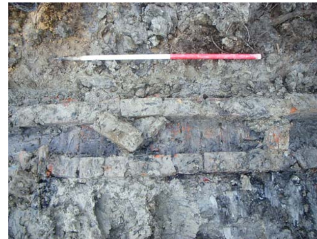
Middle part of culvert (1081), looking east. Scale 1m
