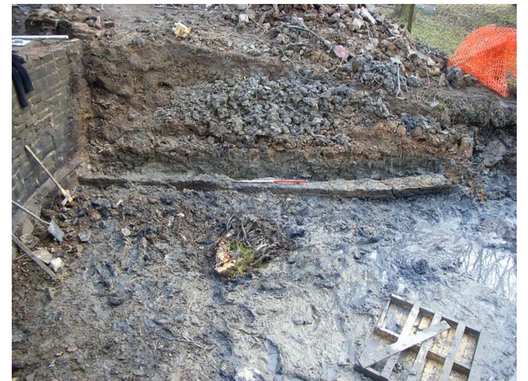
Foundations revealed after removal of east wing wall Scale 1m
