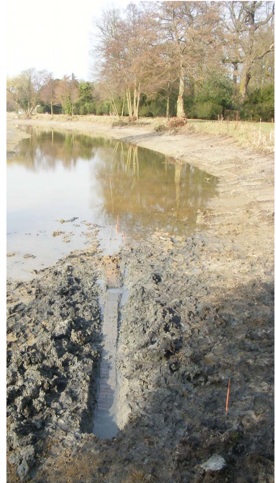
Culvert, looking north east.
