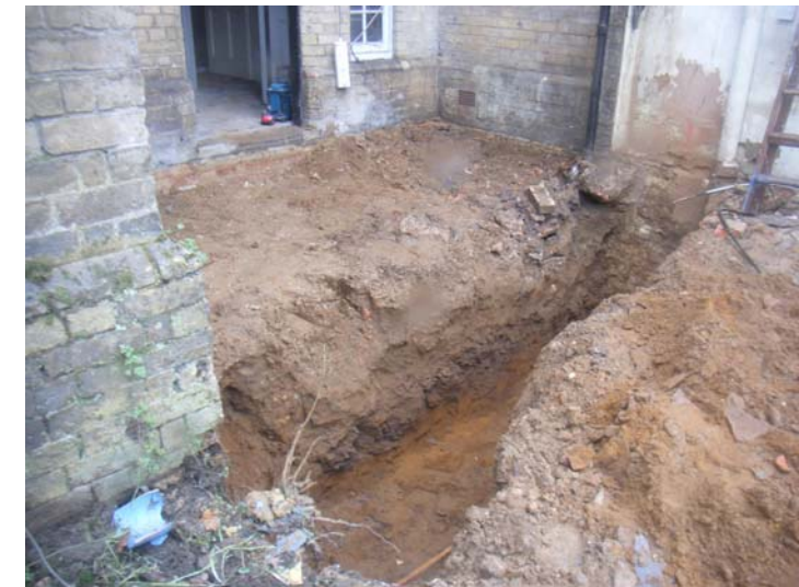
Footing trench excavated on the west side of Silsoe House Facing SE.
