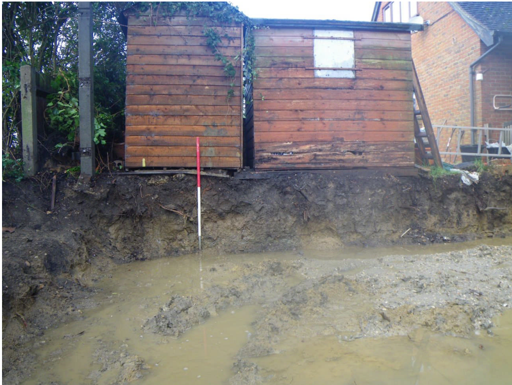
Figure 3: Soil profile in western part of site after ground reduction
