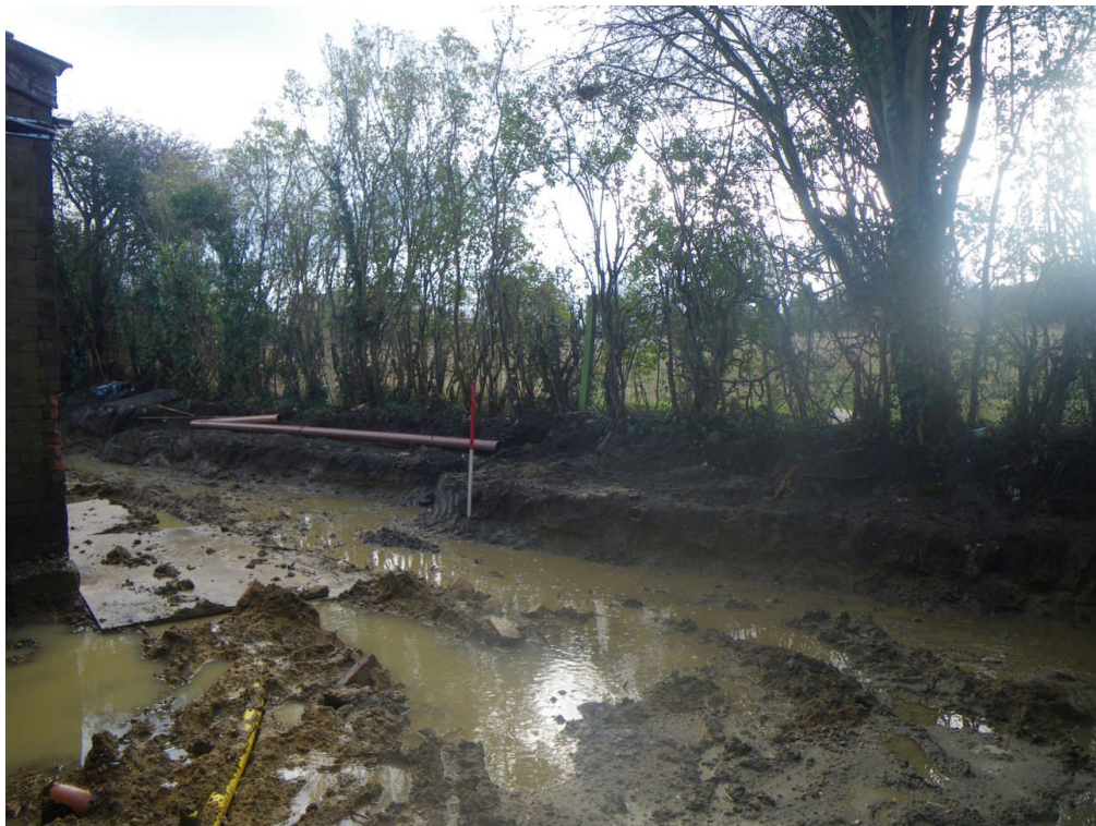
Figure 4: Soil profile in southern part of site after ground reduction
