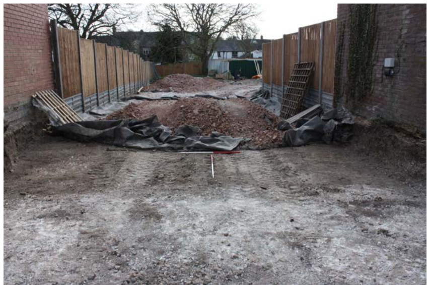
Unexcavated side of ditch [11] taken from NE (scales 1m)
