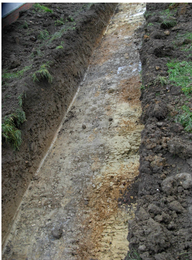
Image 3: General pre-excitation view of the northern part of Trench 5, showing ditch [504]/[506] and [512] aligned roughly N-S and curving to the SW in the south.
