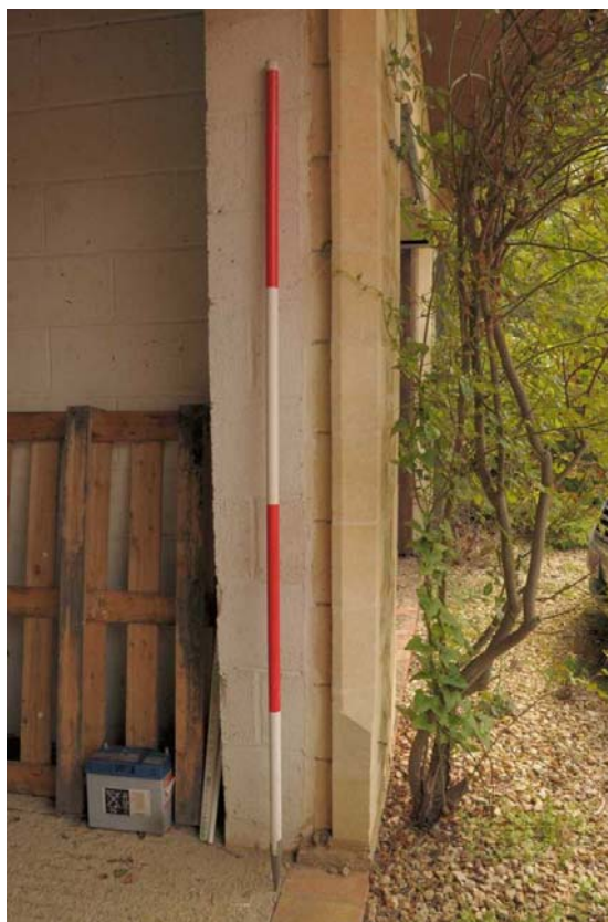
Figure 9: Breeze block and stone-clad construction of garage complex
