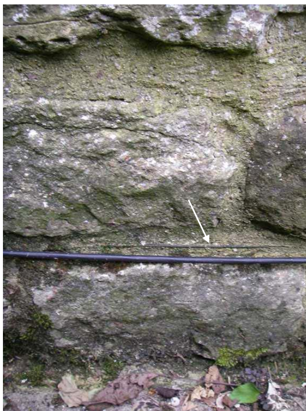
Figure 10: Damp course at base of building
