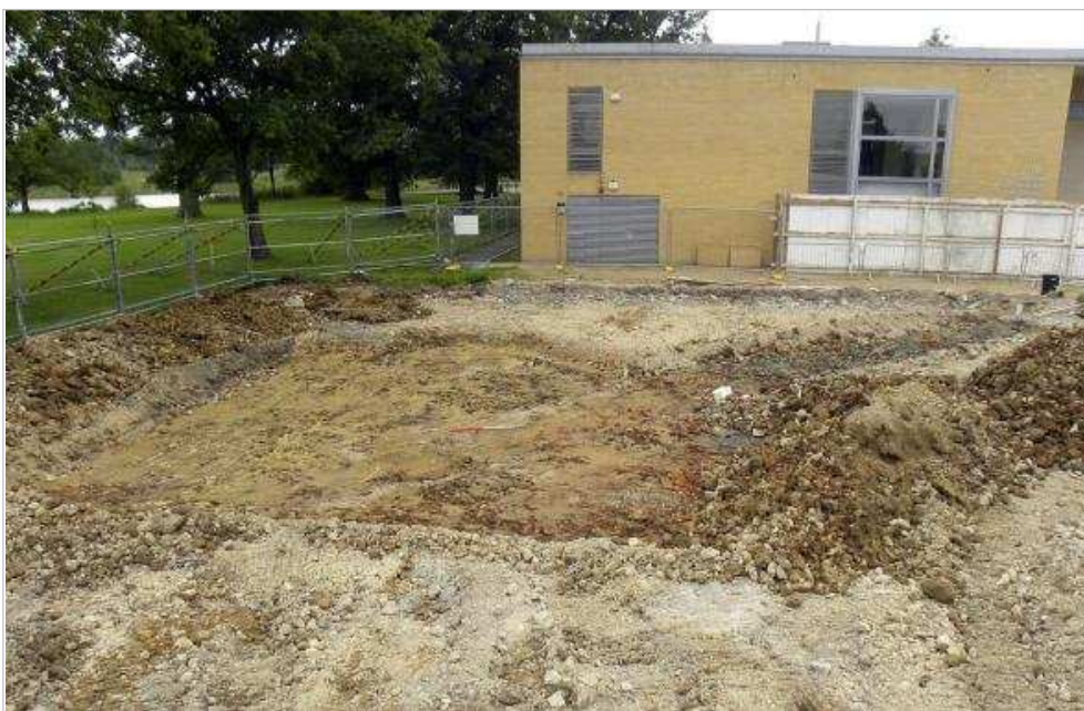
Stripped area at east end of Trench 3, viewed from north-west
