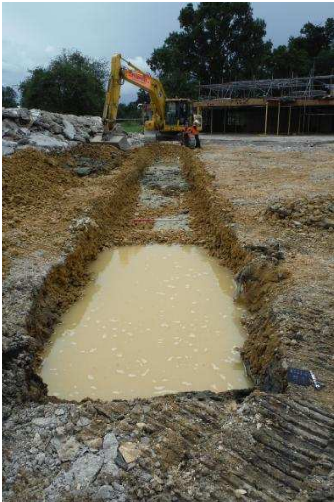
Trench 2 viewed from north-west end
