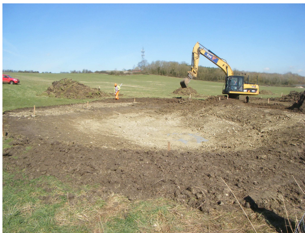
Pond B – stripped and formed to the pre-determined shape.
