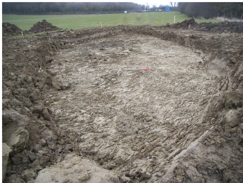
Pond D – stripped to the undisturbed geological horizon within the ‘cut’ area.
