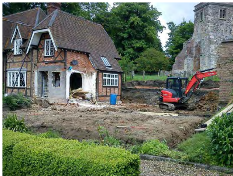
View of ground reduction to the south-east of the house (1m scale)
