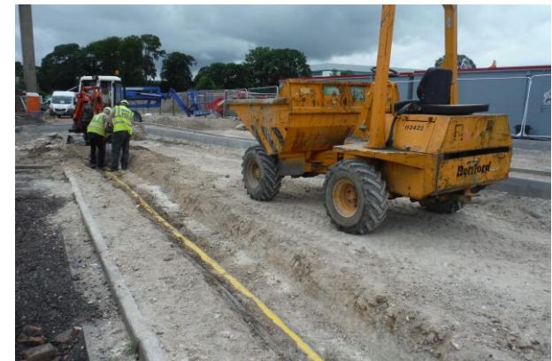
Area E: service trench, looking north
