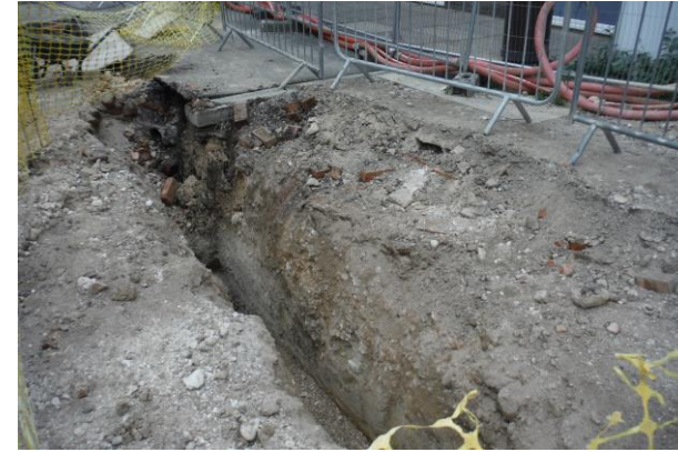
Area C: pipe trench, looking south
