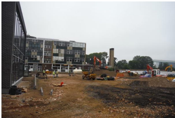
Area D: shallow stripped area, looking north
