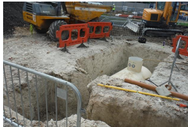
Area E: water-tank trench, looking SE
