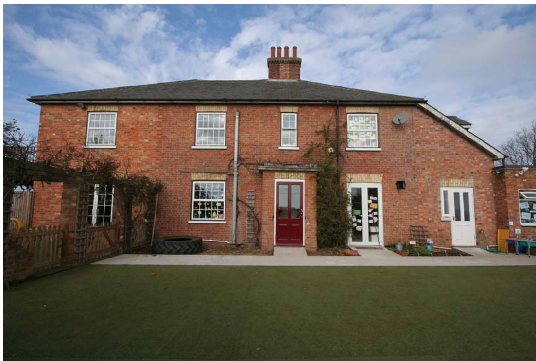
Plate 1: East elevation of building
