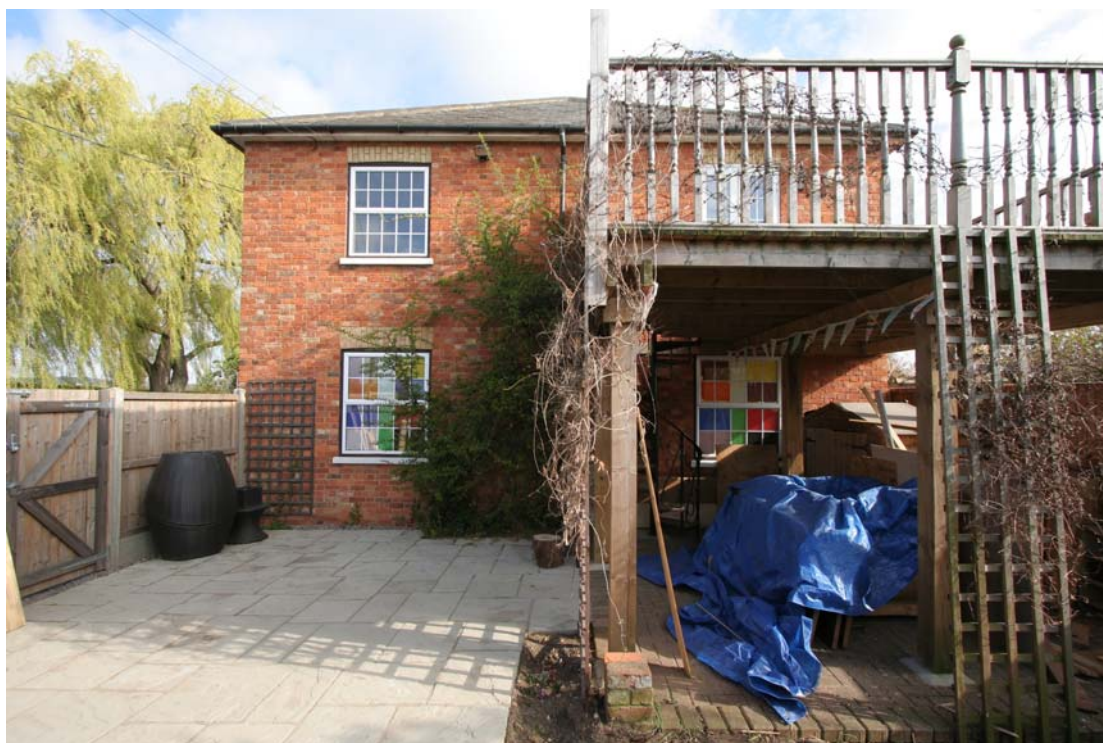
Plate 3: South end of building
