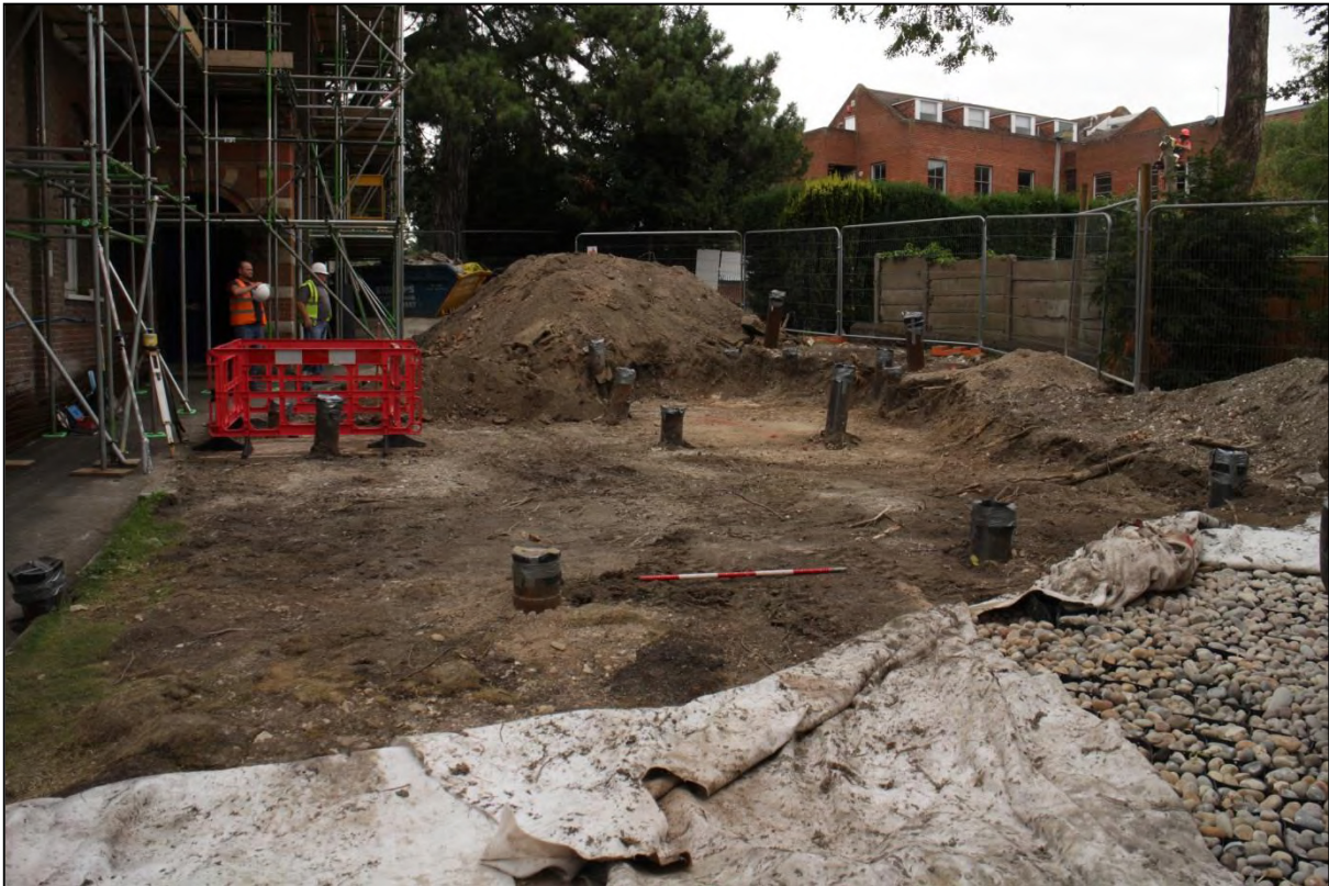
Image 1: General view of groundworks, looking west
