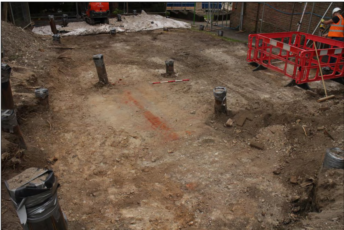
Image 2: General view of groundworks looking east
