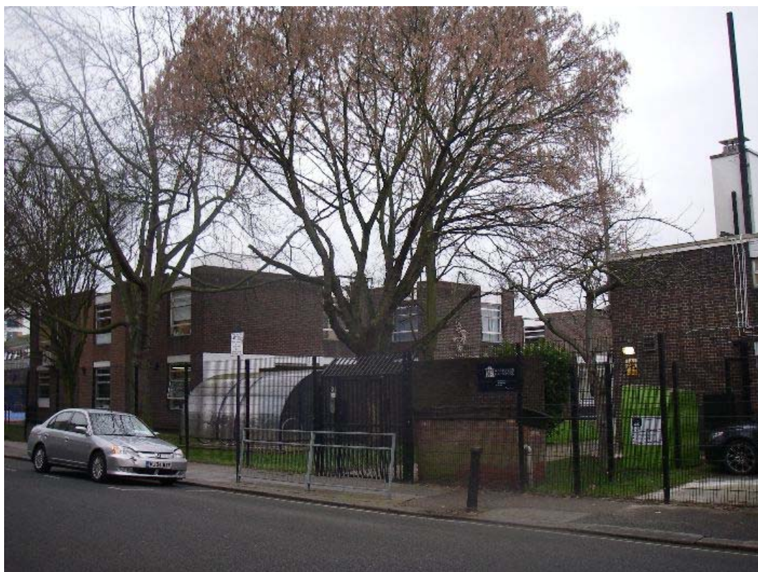
Figure 4: West London Free School in 2013, looking south-west from Cambridge Grove
