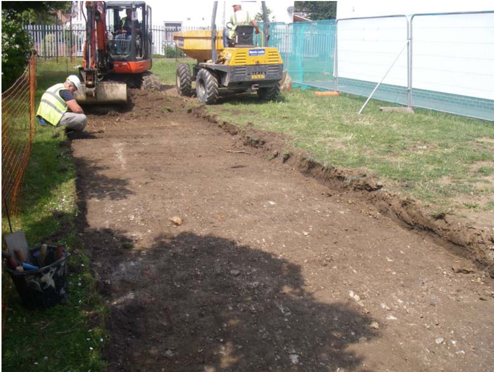
Trench 1 – excavated area for new pedestrian path
