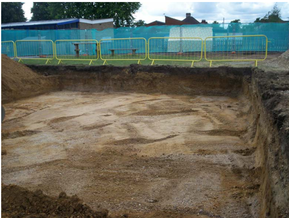
Trench 2 – excavated area for the two-classroom connect block (looking west)
