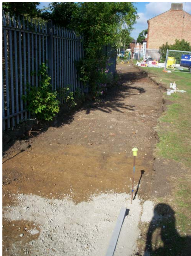
Trench 4 – excavated area for new pedestrian path
