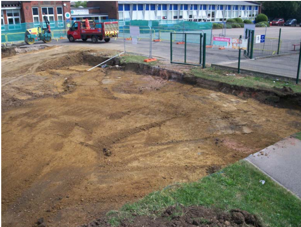
Trench 3 – excavated area for the eight-classroom connect block (looking north-east)
