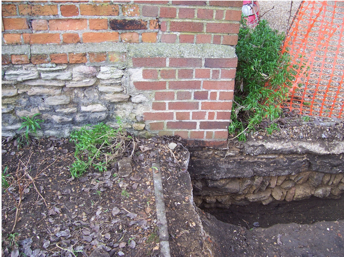
Figure 8: Foundation of wall in Trench 5 in context with upstanding wall
