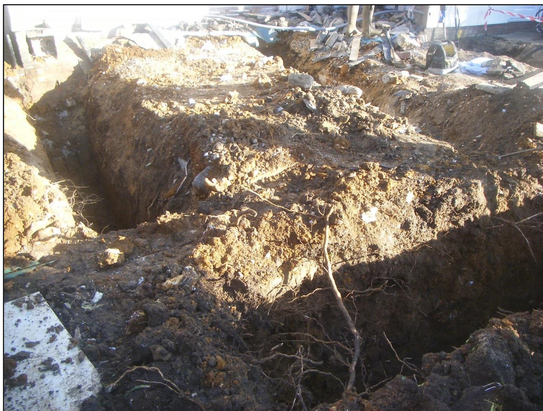
Figure 3: General view of footings looking south-east
