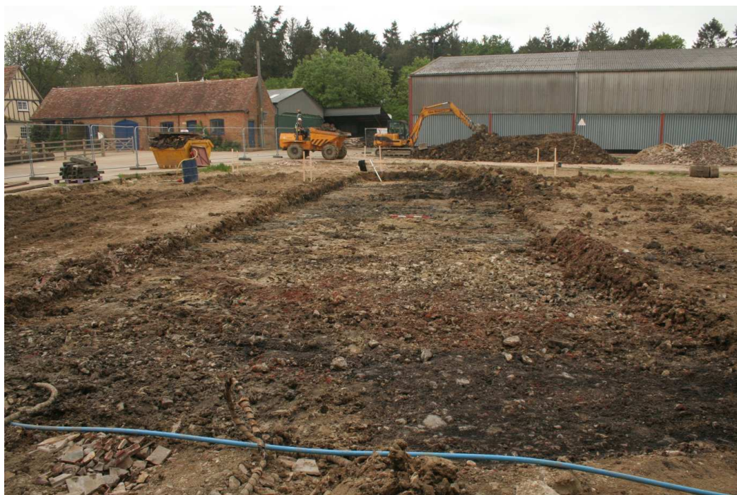
Image 4: Zone E during the construction phase
