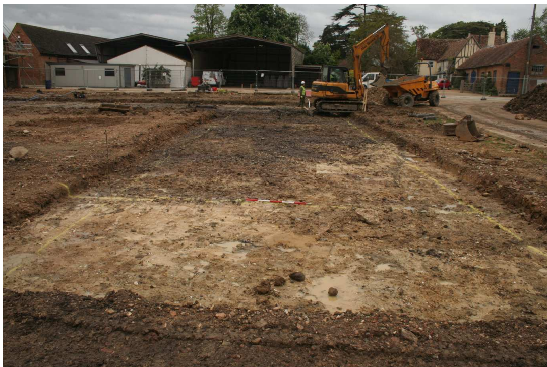
Image 5: Zone E during the construction phase
