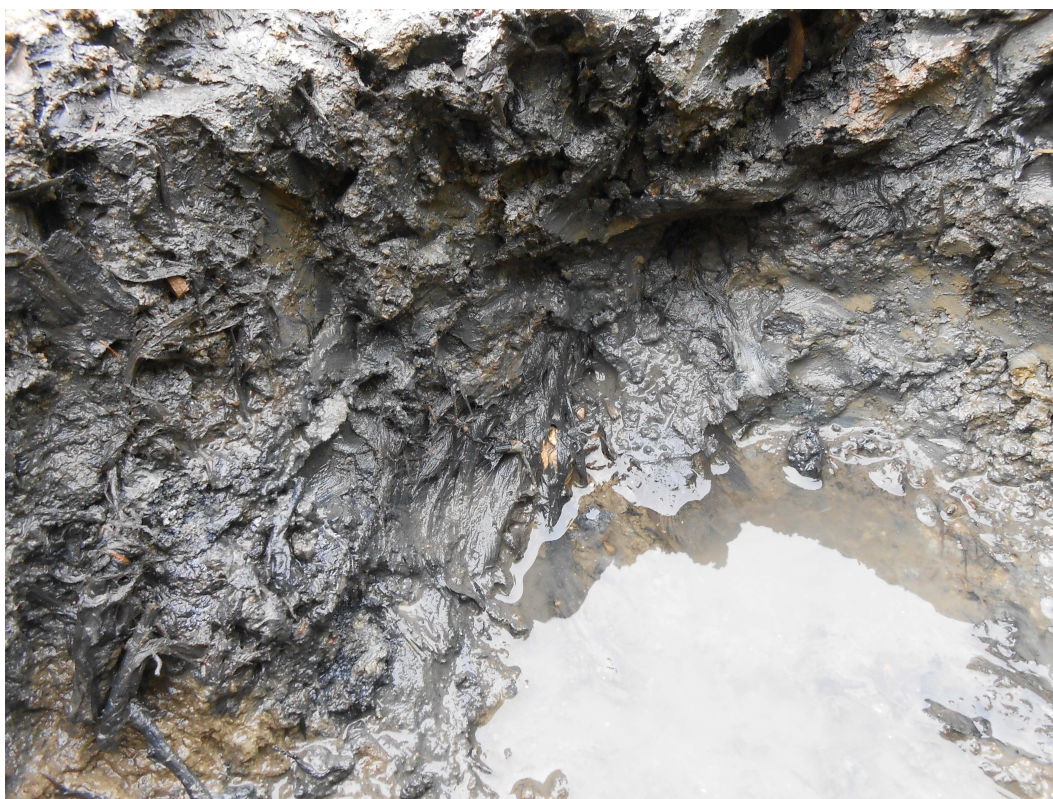
Image 8: Investigation of the wattle-lined pit during the recent mitigation works, showing the considerable deterioration in the wood.
