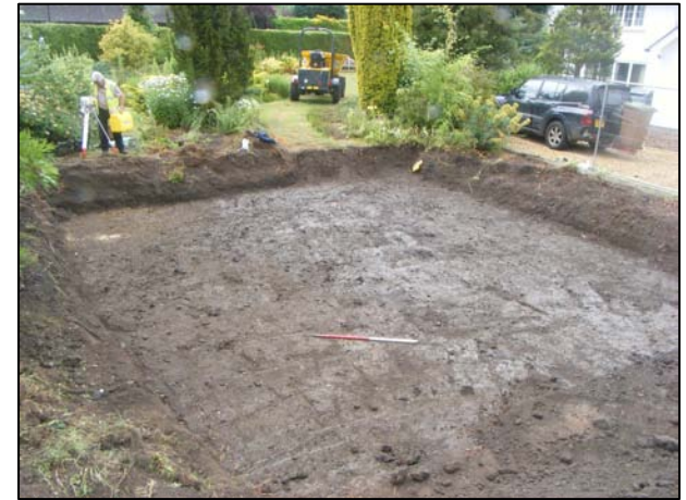
Area 1 – looking northwest (1m scale)
