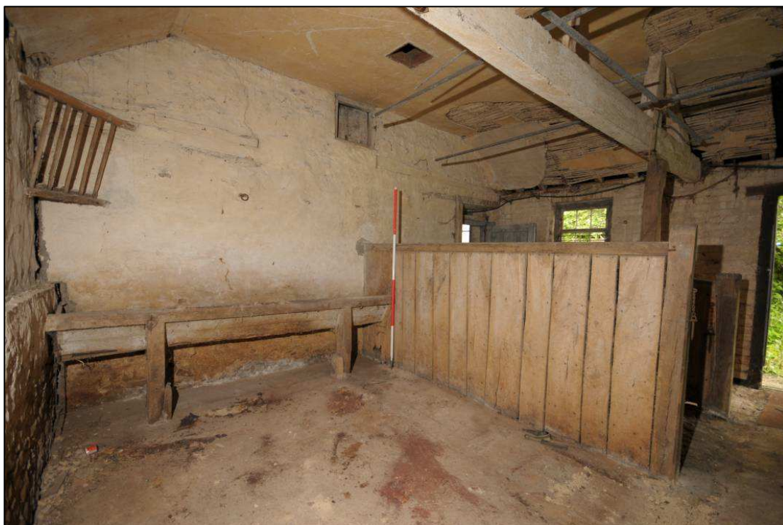
Image 11: West range: Interior of stable looking north-east (Loose box with feed trough and hay rack)
