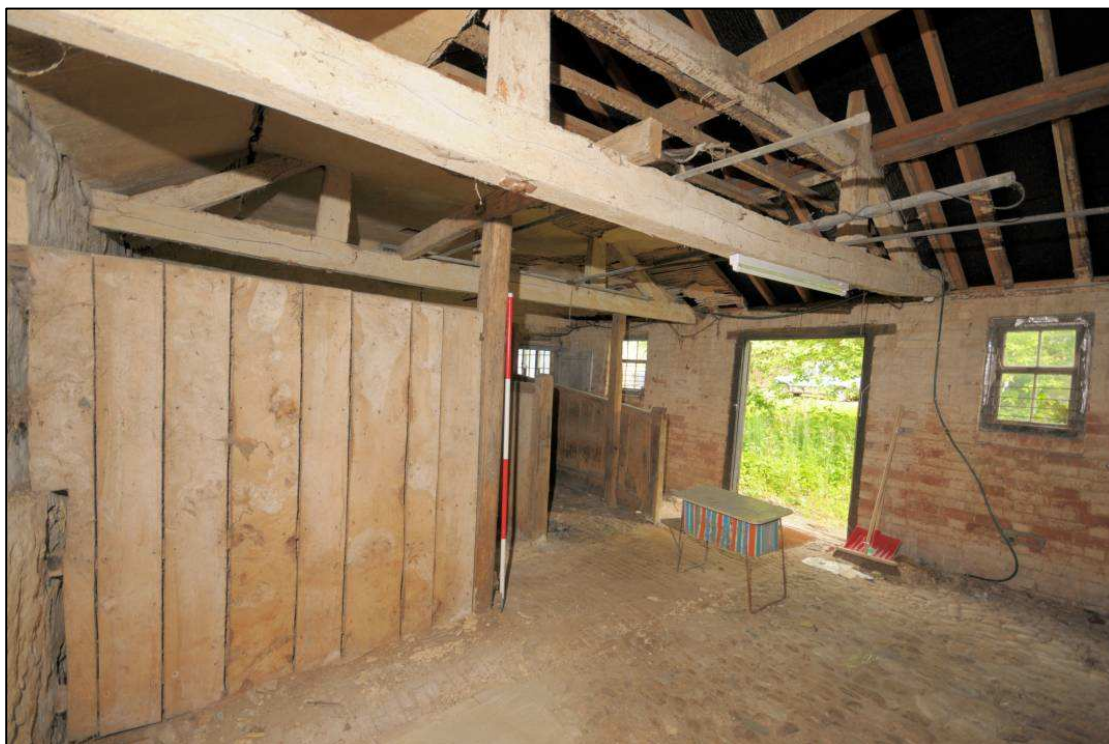
Image 9: West range: Interior of stable looking north-east
