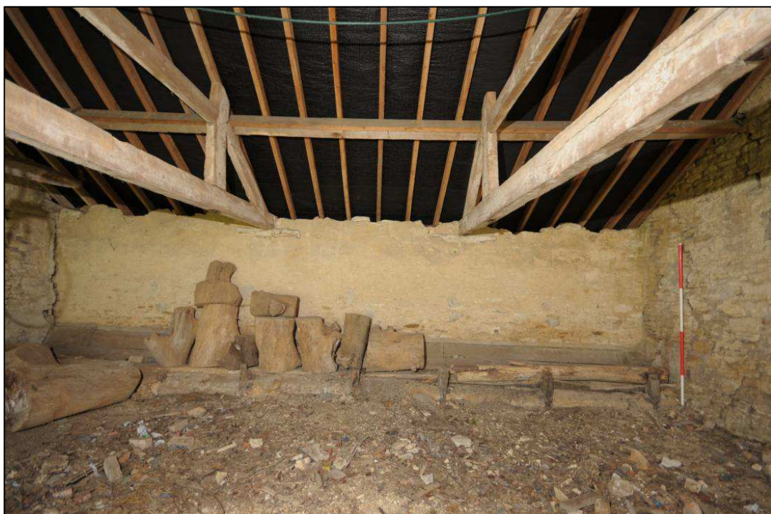
Image 22: West range: Shelter shed, west wall
