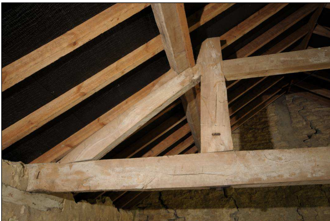
Image 26: West range: Shelter shed, detail of queen post roof truss
