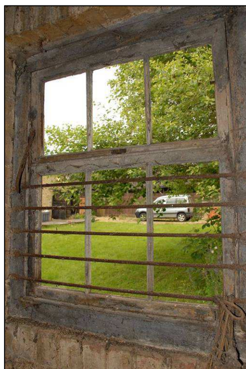
Image 12: West range: Details of stable window
