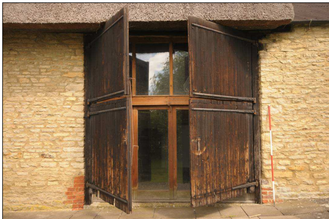
Image 34: North range: Barn, detail of double doors
