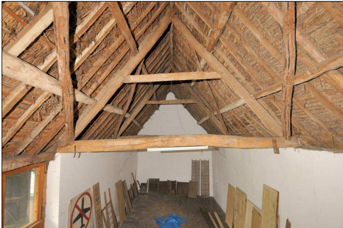
Image 32: North range: Barn, detail of roof over western section
