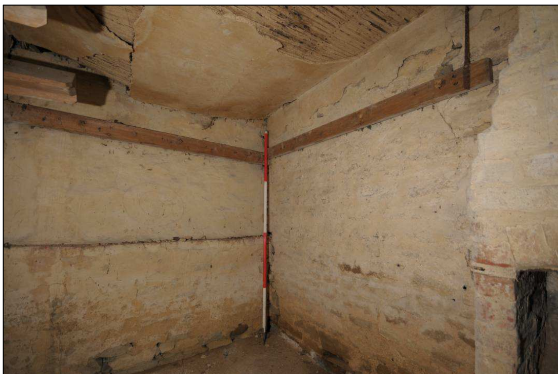
Image 16: West range: Tack room showing north-west corner
