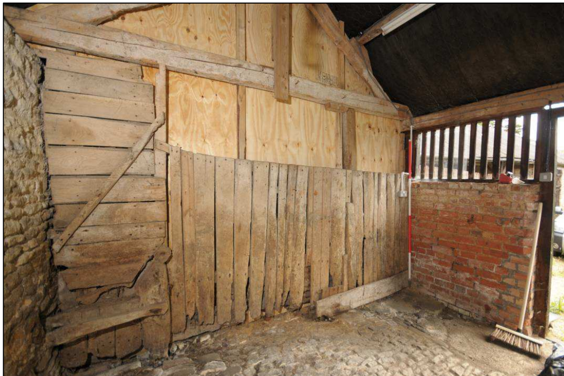
Image 36: North range: Stable, looking south-east
