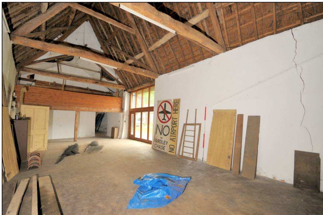
Image 28: North range: Barn, western section, looking south-east
