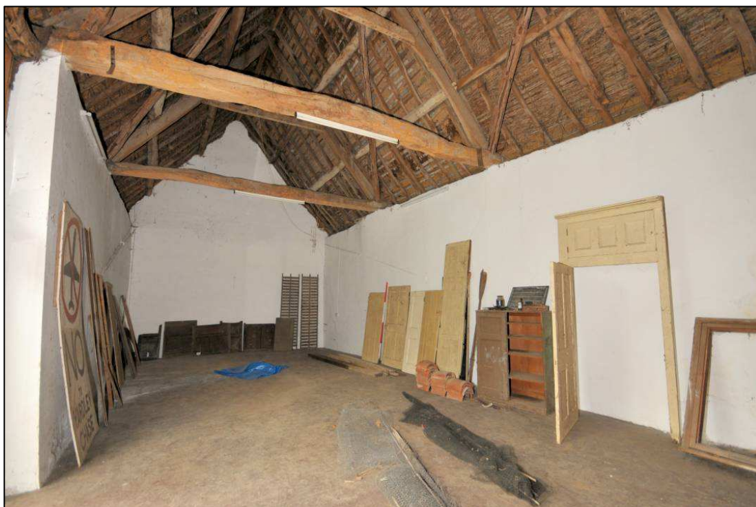
Image 27: North range: Barn, western section looking north-west
