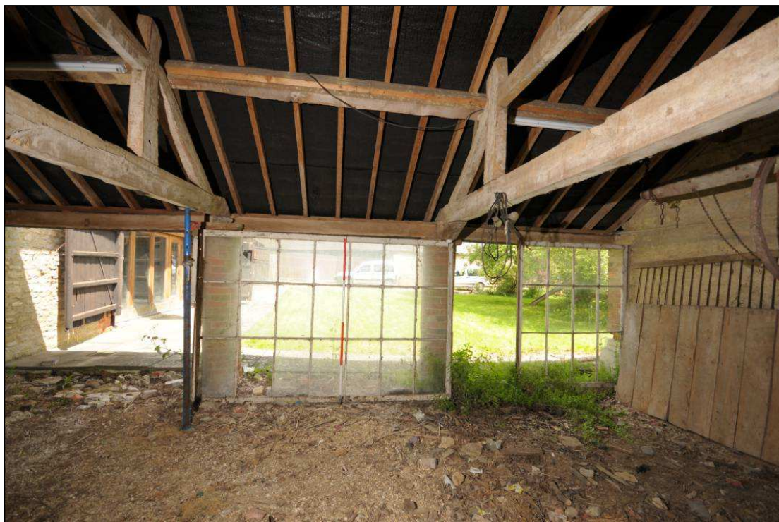
Image 25: West range: Shelter shed, east side
