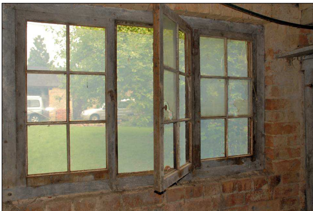
Image 18: West range: Tack room window
