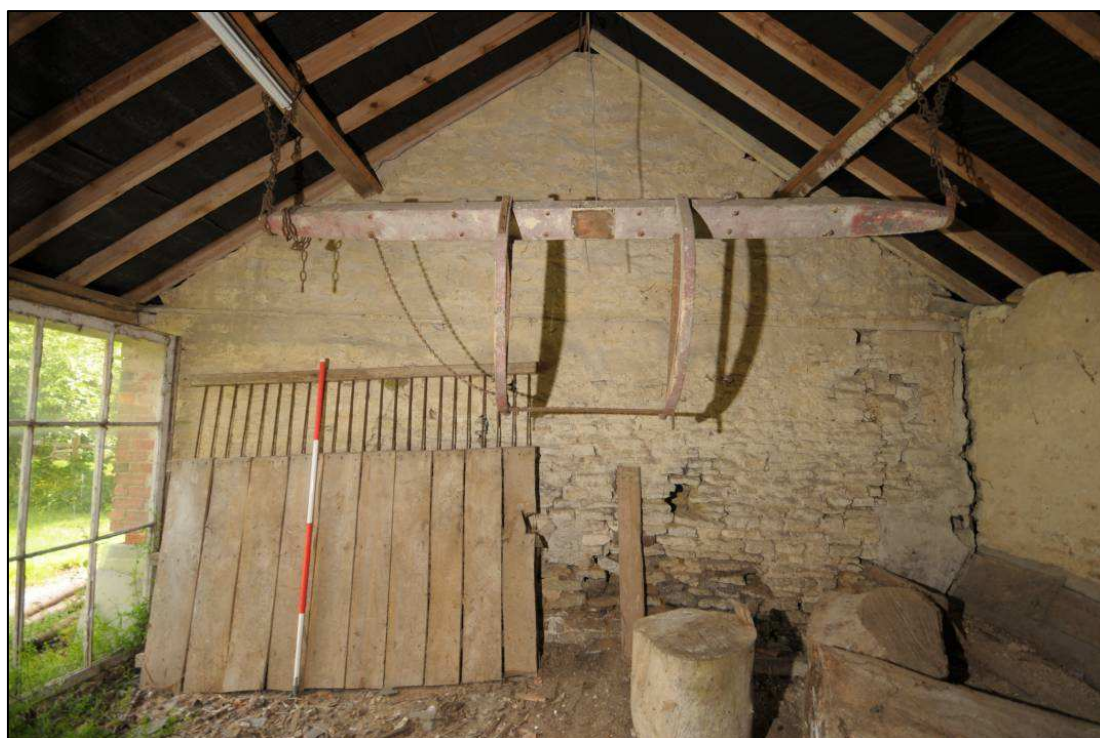
Image 24: West range: Shelter shed, south wall
