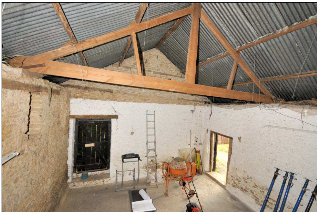
Image 33: North range: Barn, detail of roof over eastern section
