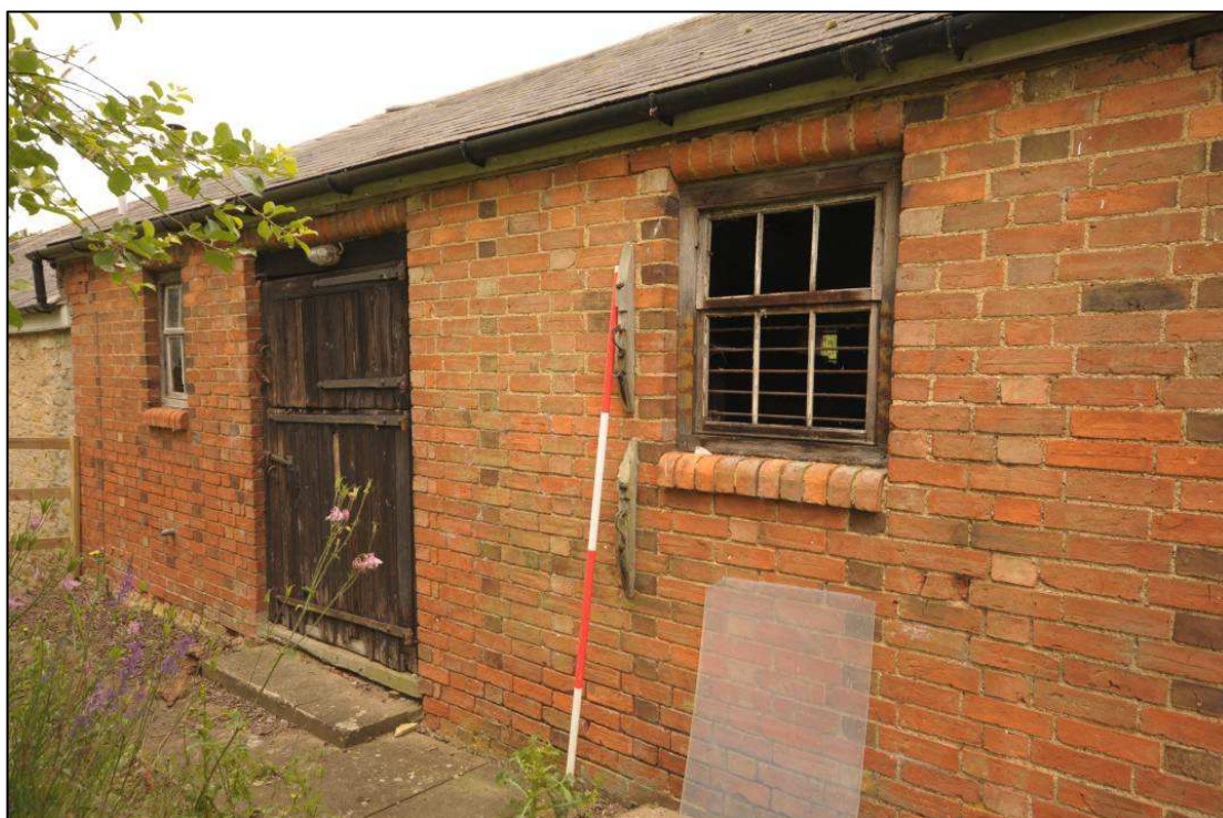
Image 6: West range: showing east wall of stable
