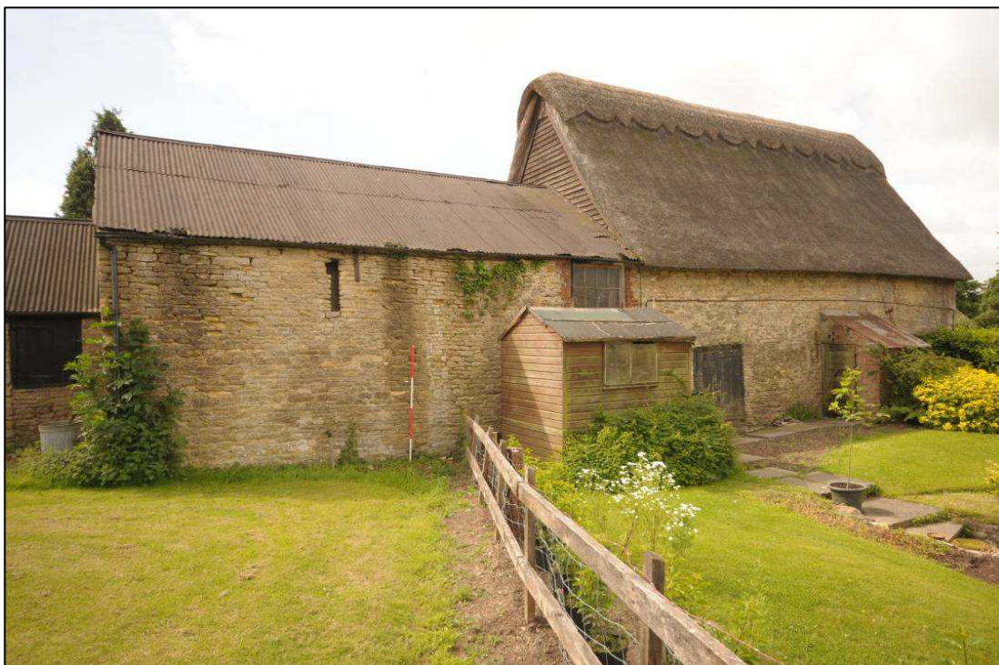
Image 4: North range, view looking south
