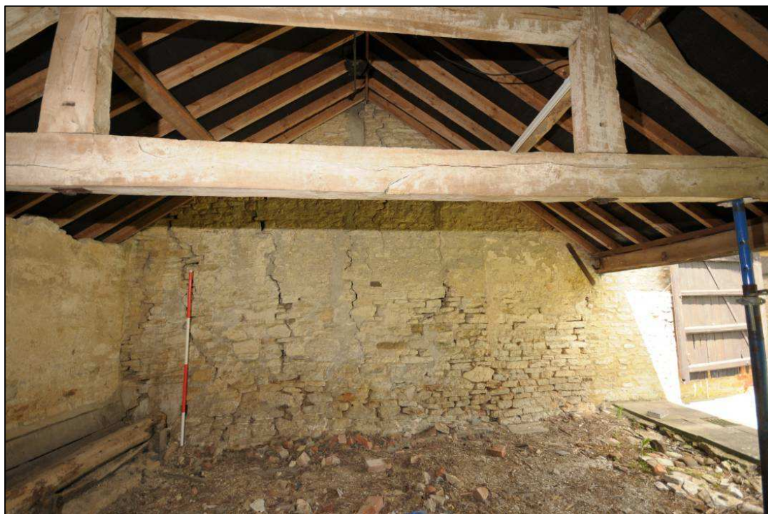
Image 23: West range: Shelter shed, north wall
