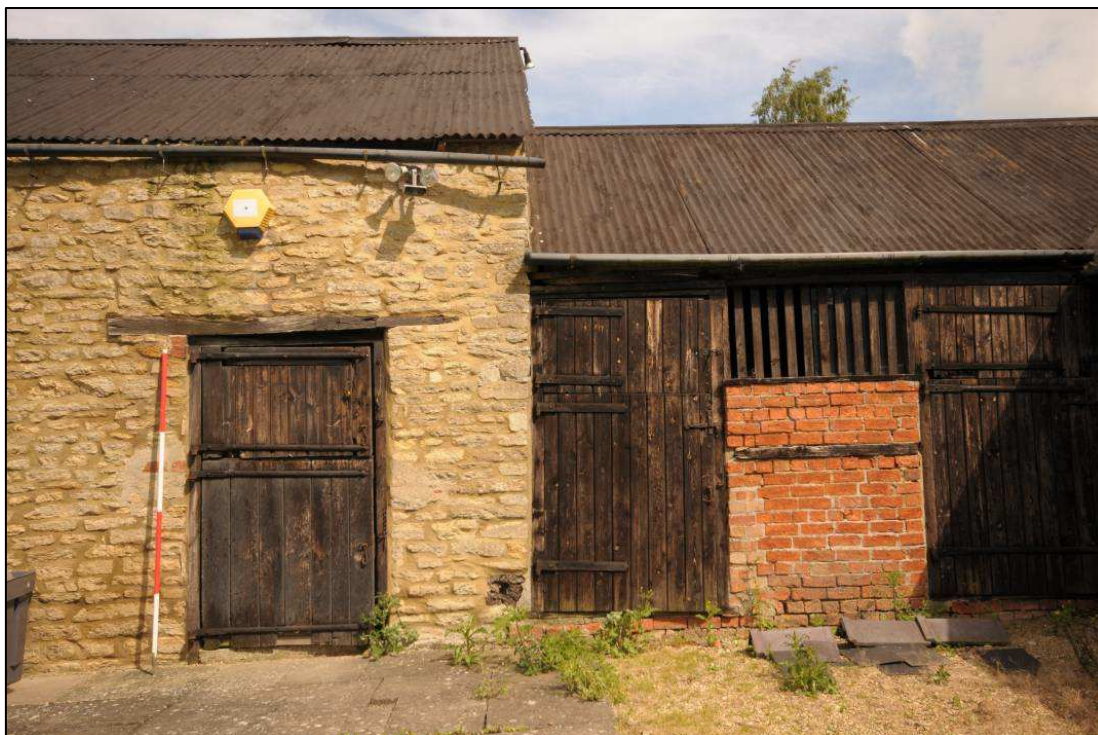
Image 35: North range: detail of doors in barn and adjacent stable
