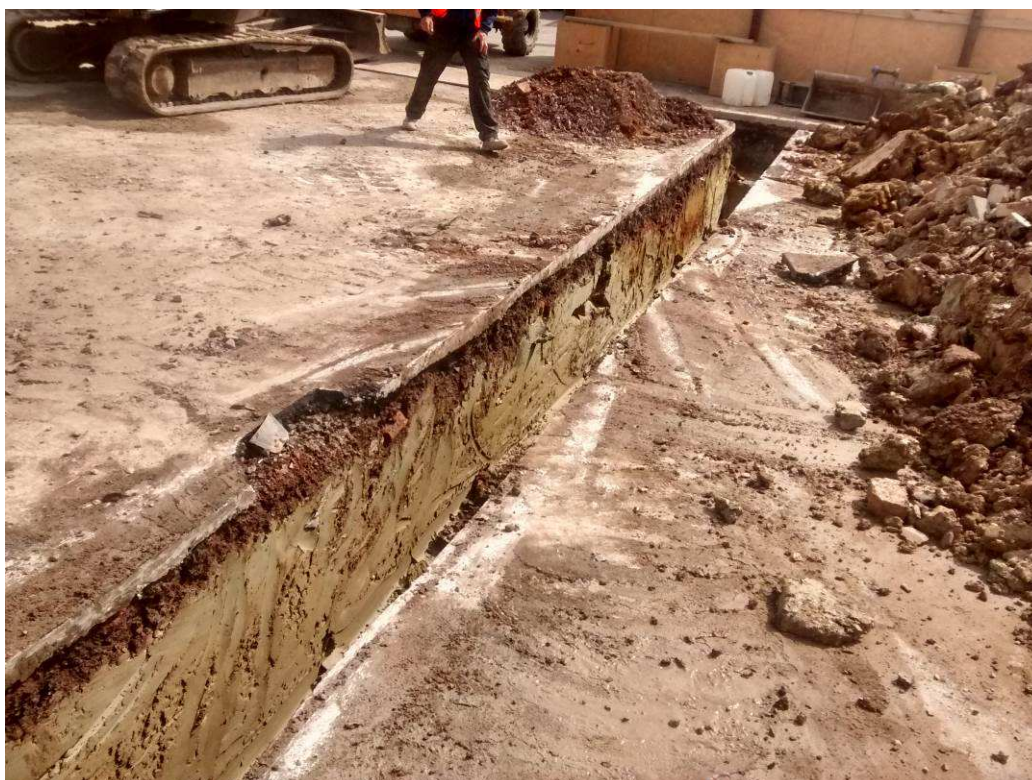
Figure 3: Typical trench section to south (looking SE)
