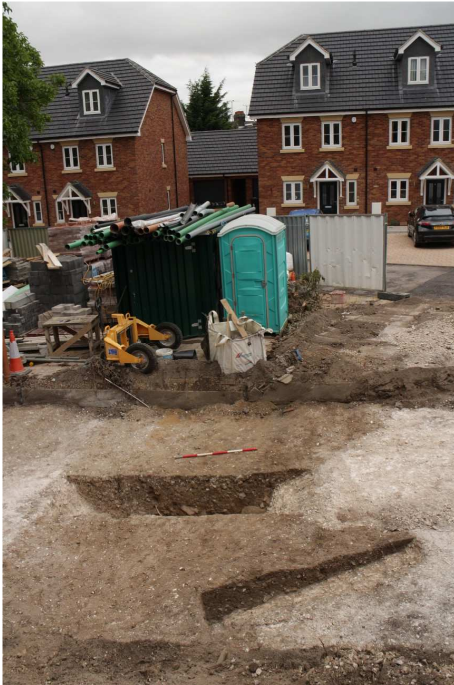
Image 1: View of site looking north-west
