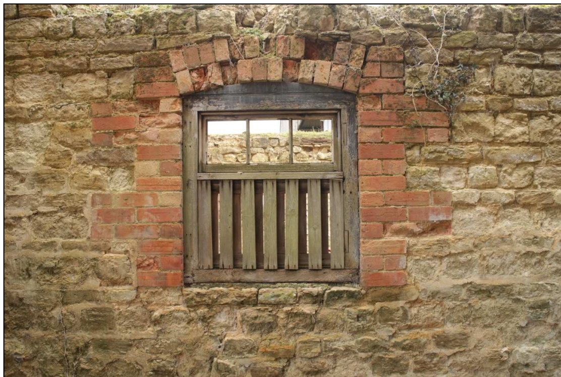
Image 15: North range: C6: Exterior window detail: north wall Shows slatted section in lower part and horizontal hinged light above
