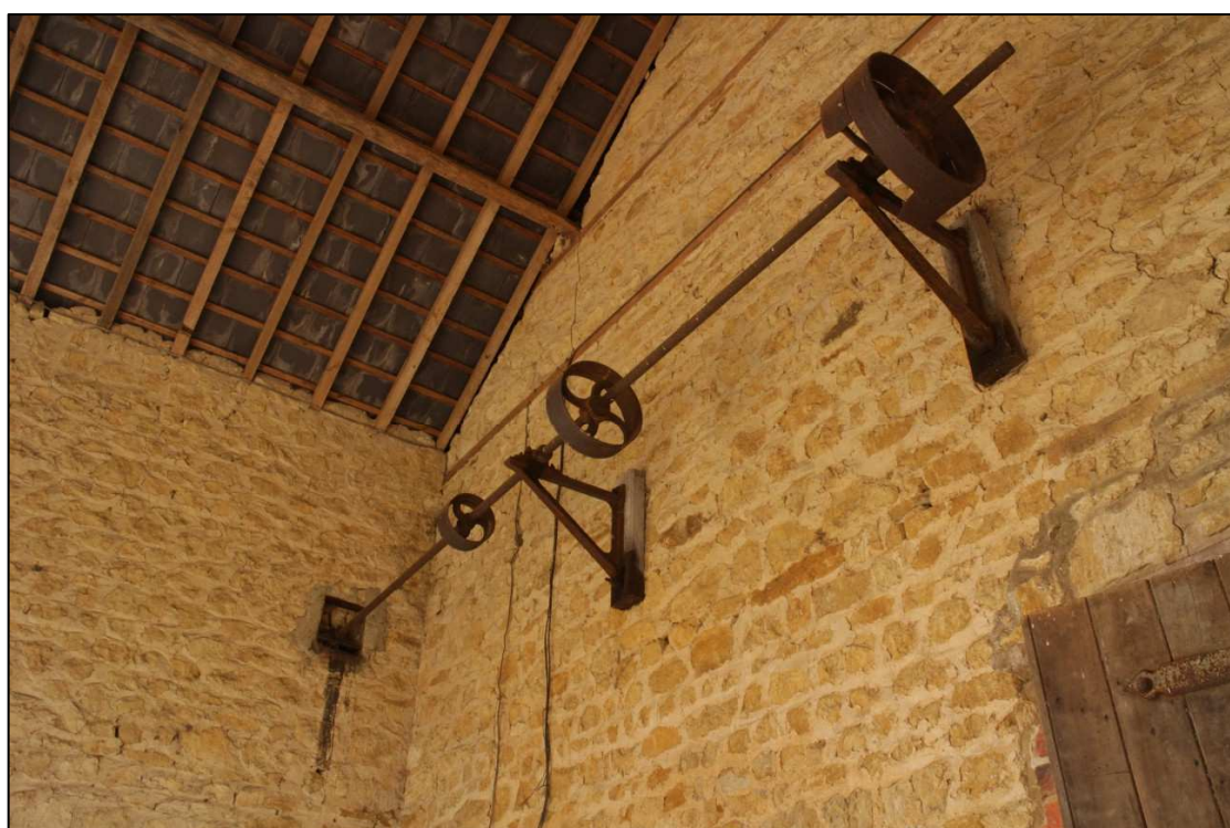
Image 24: North range: C7 Barn: Interior detail showing line shafting
