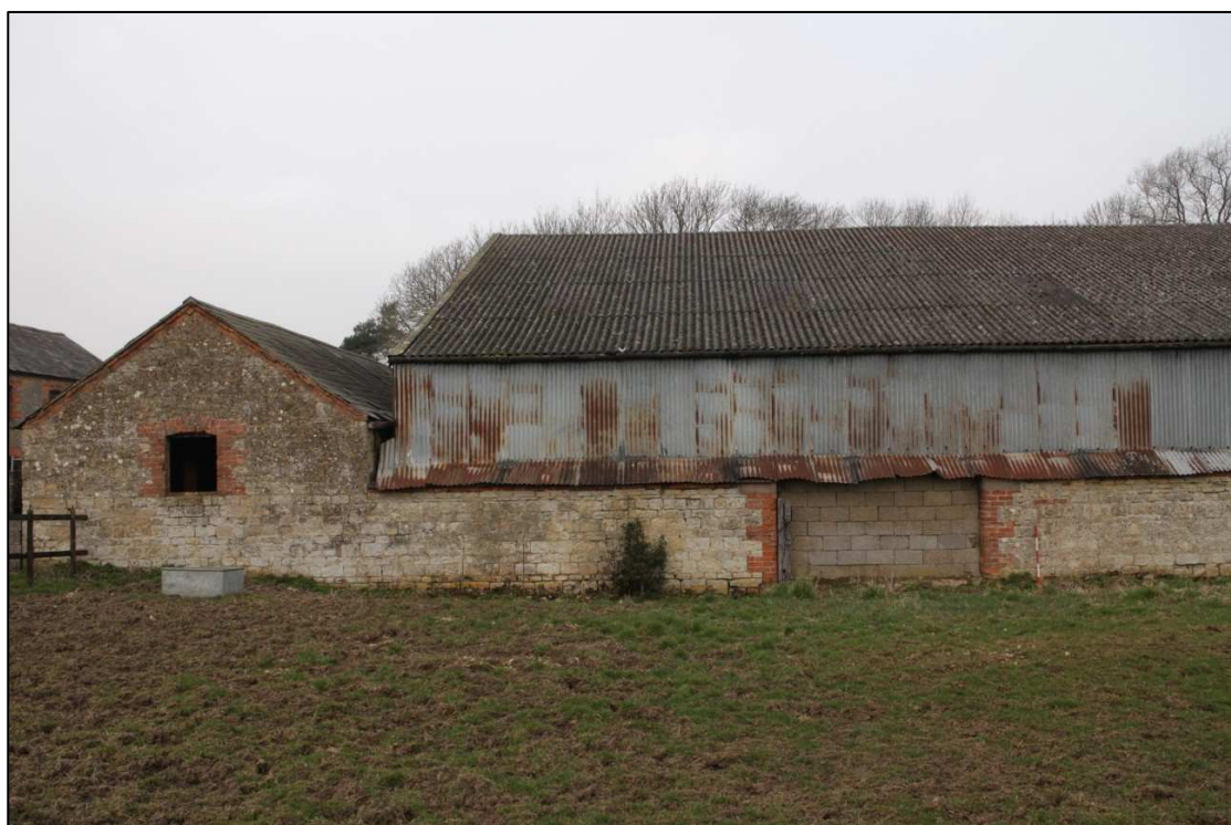
Image 4: General view of plots 3 & 4 from the south (west half) Shows enclosure yard wall with blocked opening, end of west range and modern building within yard area
