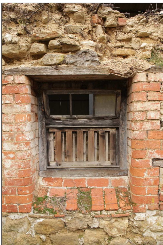
Image 16: North range: C6: Interior window detail: north wall Shows bullnose bricks on the sides of the opening and tile dressing to sloping section below
