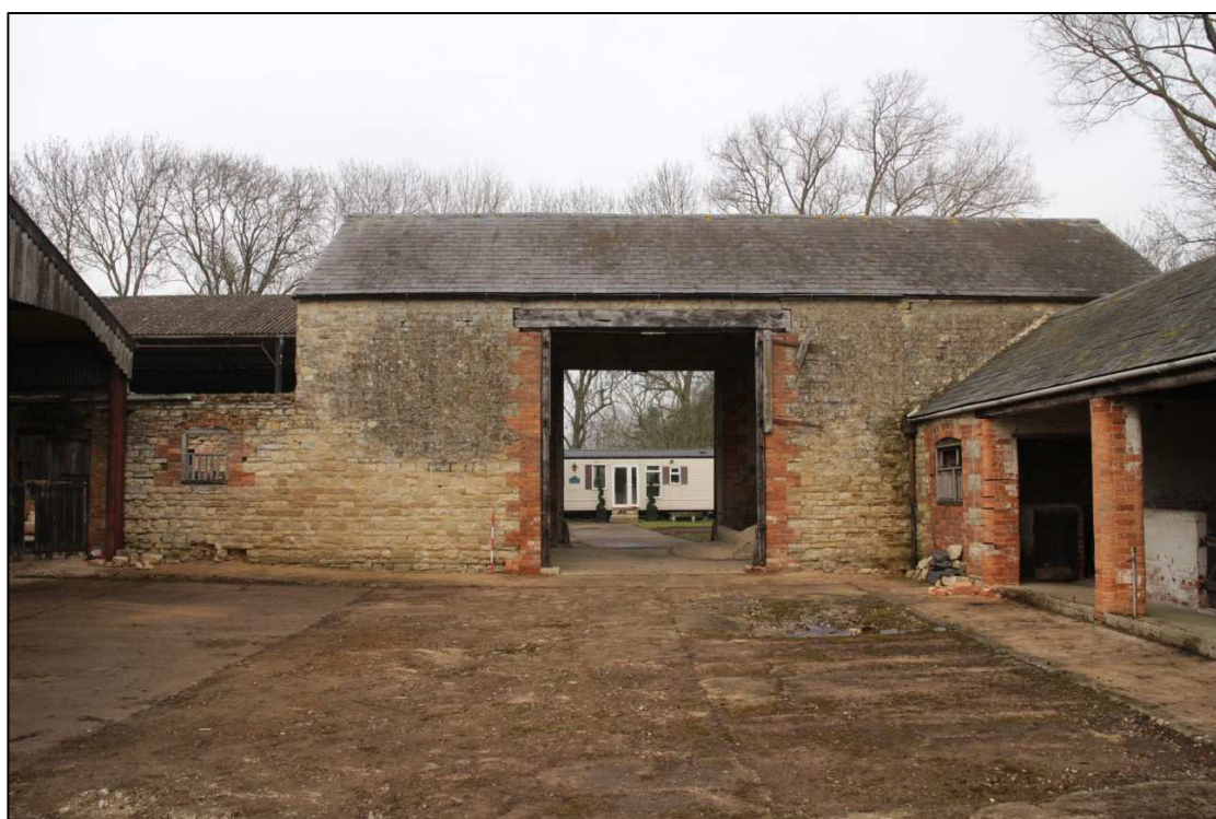
Image 18: North range: C7 Barn: Exterior view of south elevation
