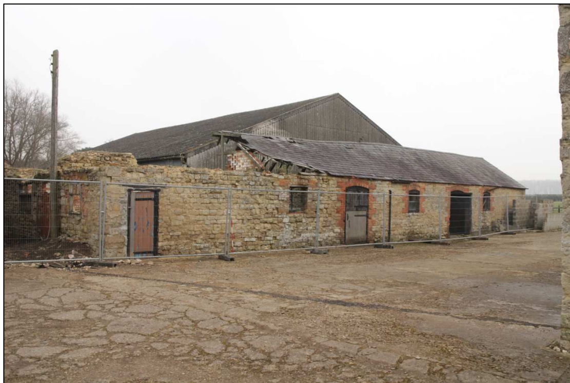
Image 5: West range, exterior elevation
