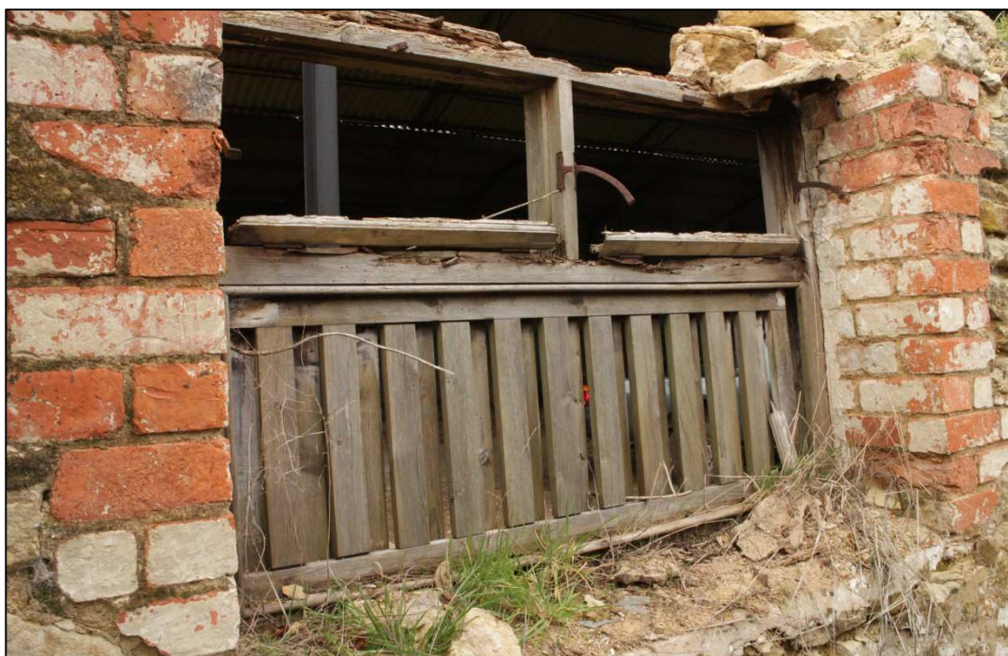
Image 12: North range: C5: Window detail
