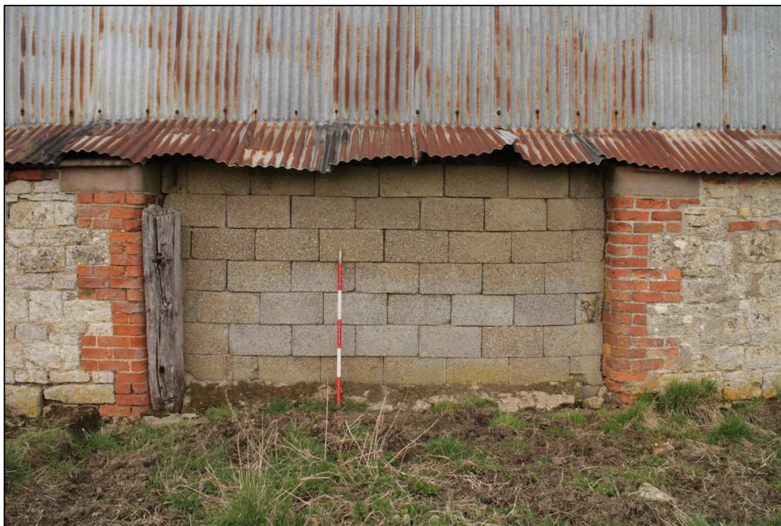
Image 31: Yard wall: Detail of western opening
