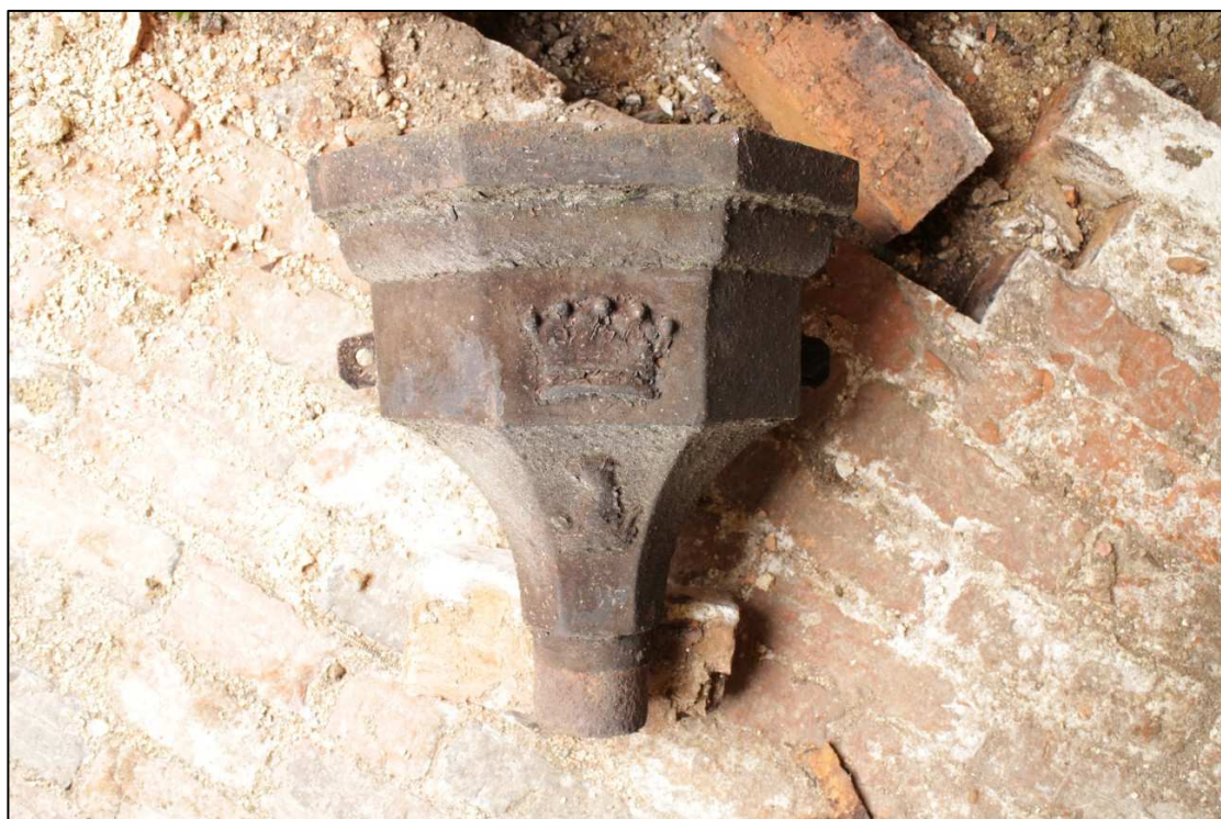
Image 32: Detail of rainwater head
