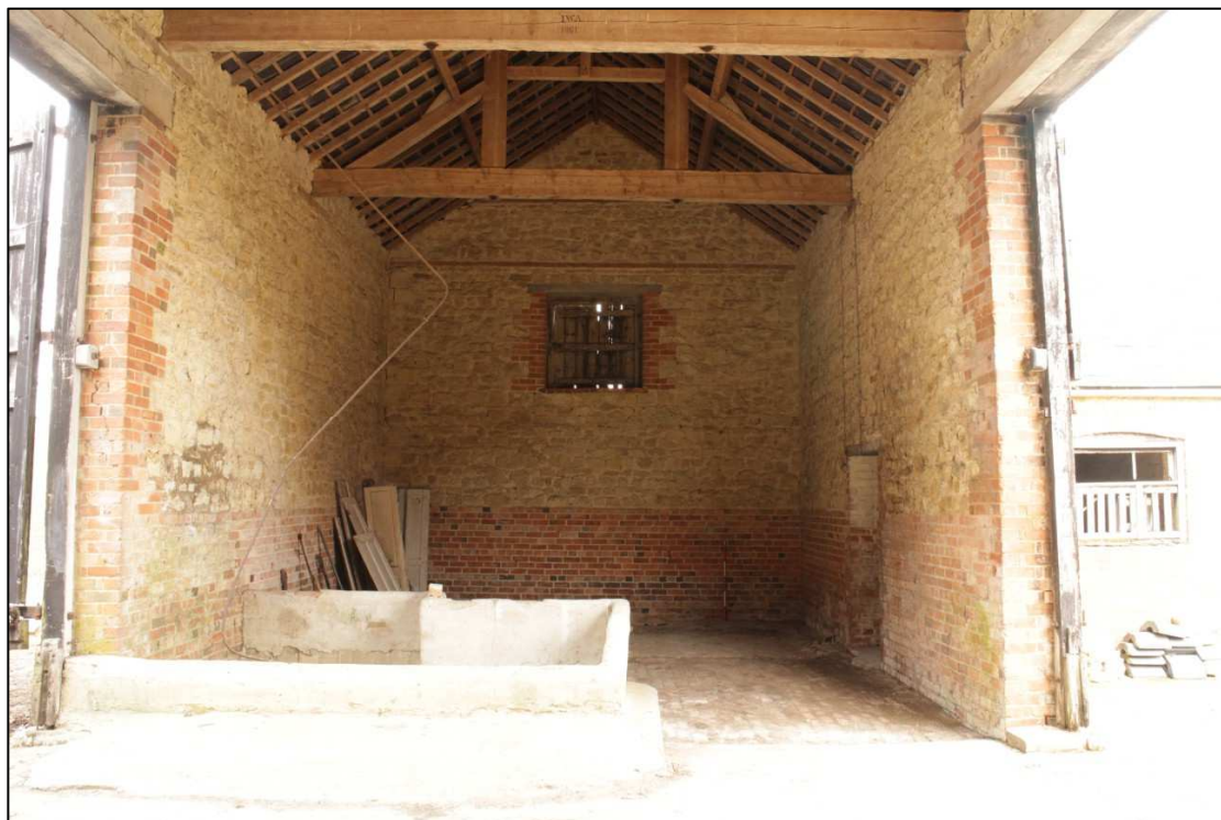
Image 21: North range: C7 Barn: Interior looking east
