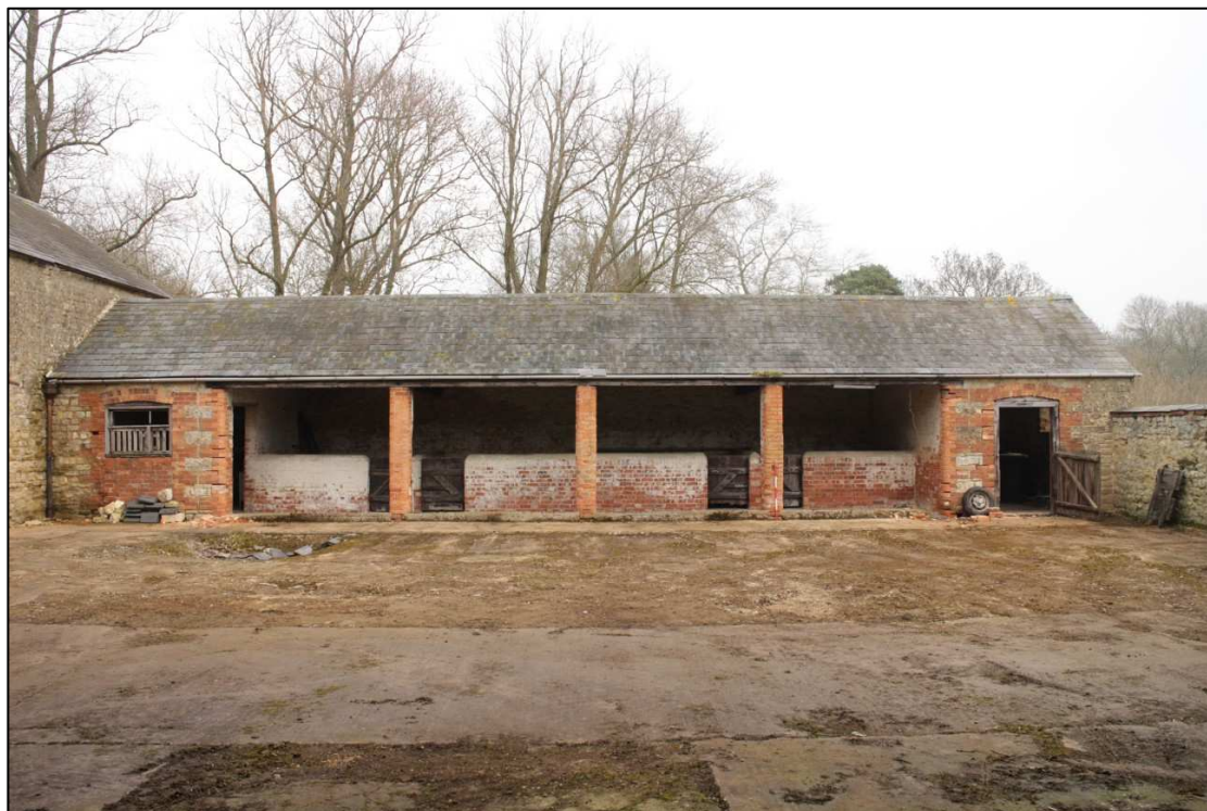
Image 27: East range: West side
