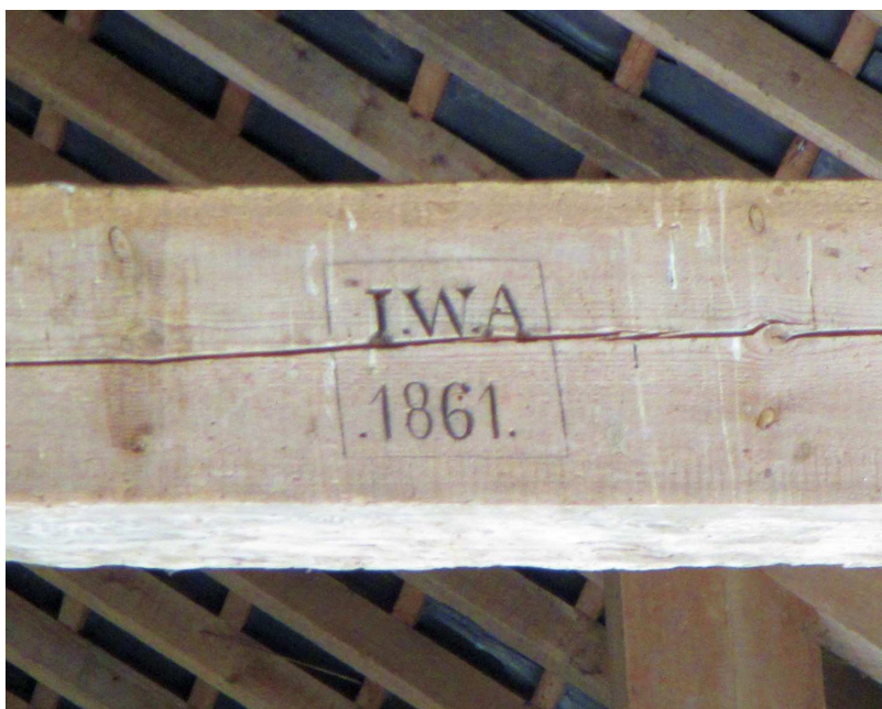
Image 23: North range: C7 Barn: Detail of date and initials
