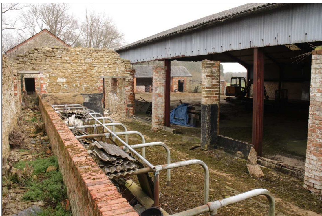
Image 11: North range: C5: Interior, looking south-east Shows brick pillars of original open front and 20th century stalls
