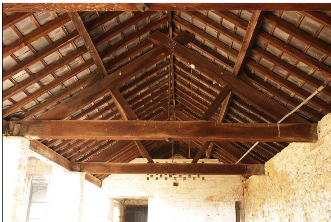
Image 28: East range: Roof structure
