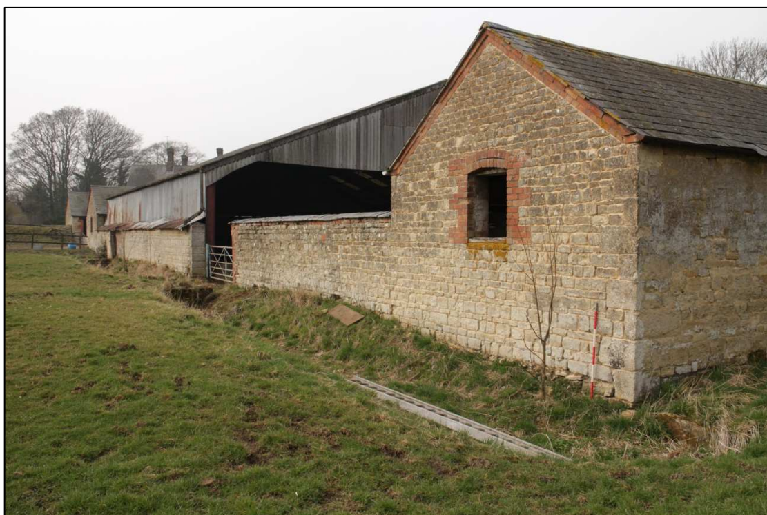
Image 26: East range: Exterior view of south gable end
