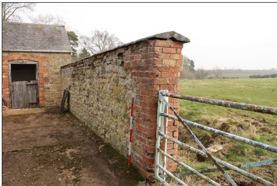
Image 30: Yard wall: east end
