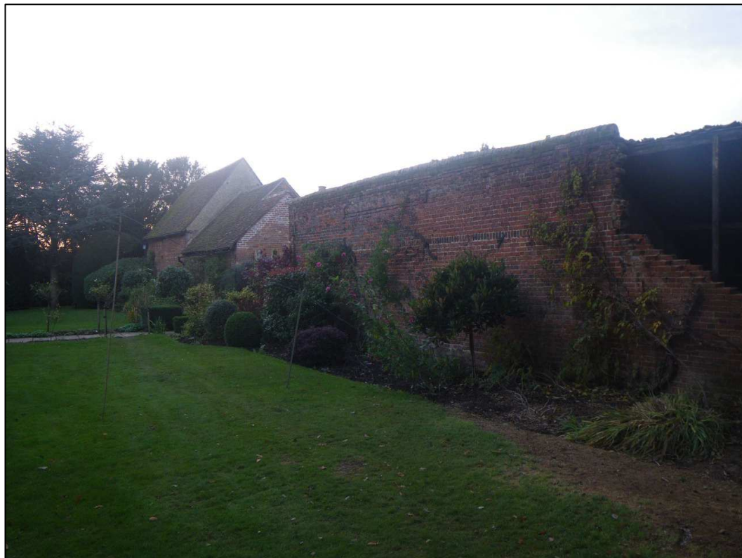
Image 2: Rear wall of building prior to development (View looking west from garden. Photographed in 2013.)
