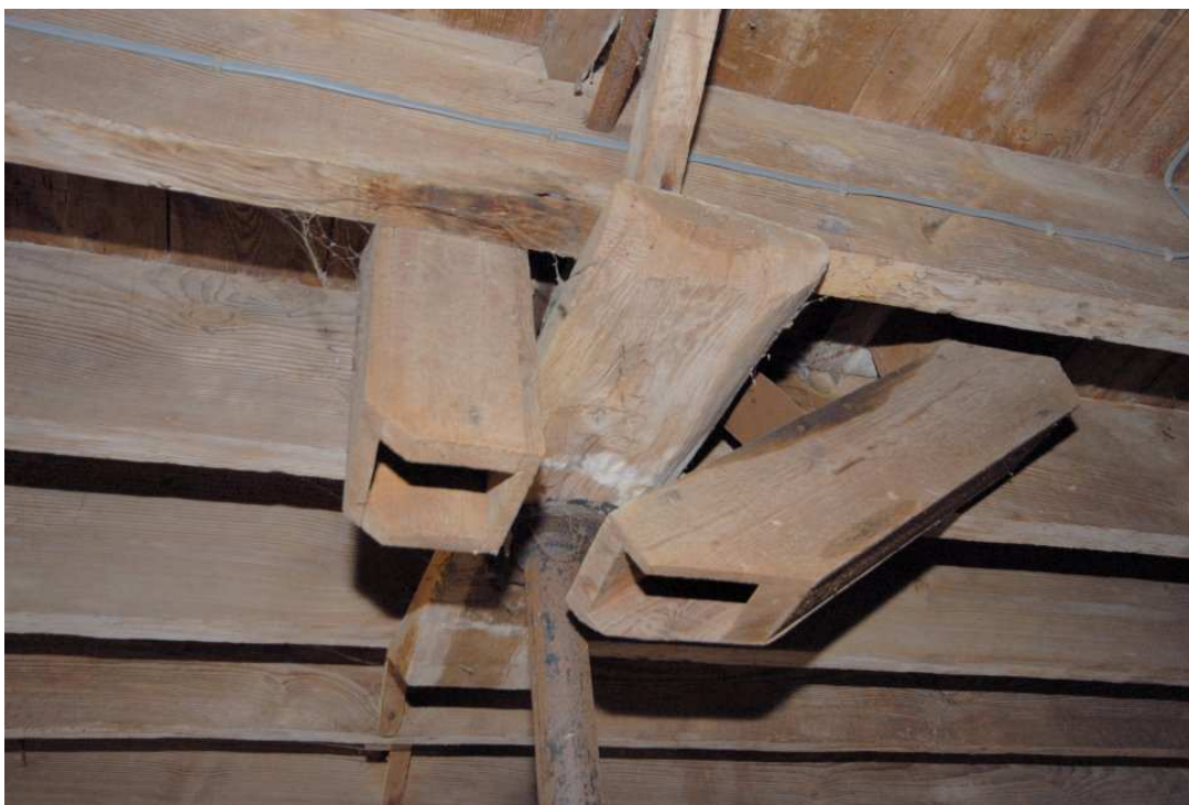
Image 21: Long Barn C1, detail Wooden chutes in centre of ceiling
