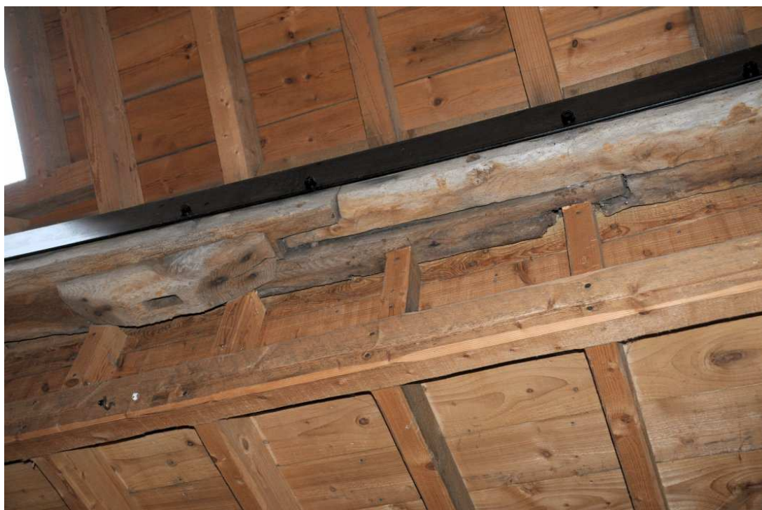
Image 8: Bean Barn, scarf joint in north aisle plate
