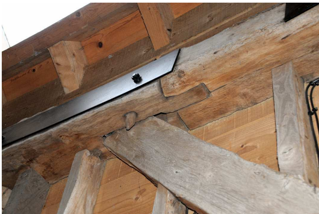
Image 7: Bean Barn, scarf joint in north aisle plate
