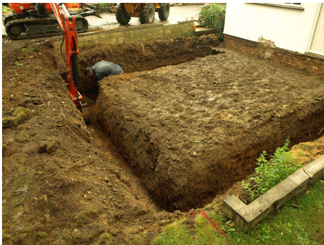
Figure 4: Post-excavation photograph from south-east
