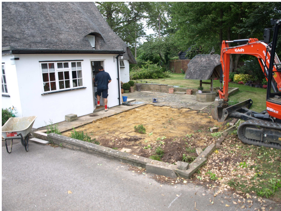
Figure 3: Pre-start photograph from south-west
