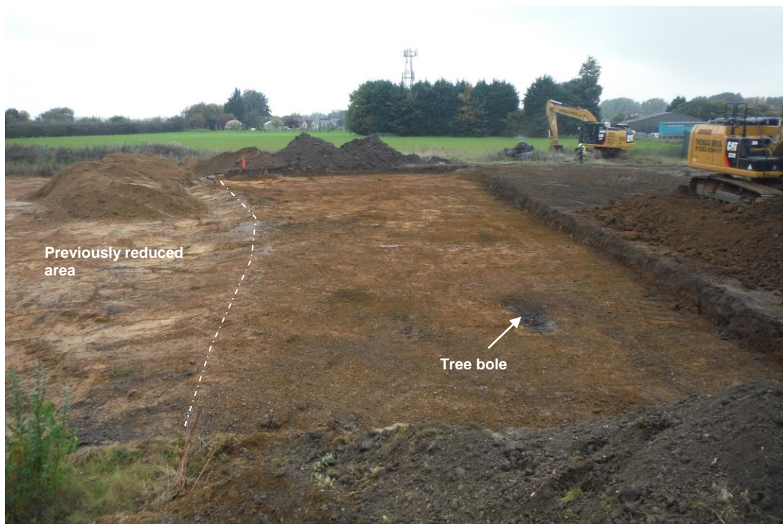
Figure 4: Newly excavated area, looking north (1m scale)
