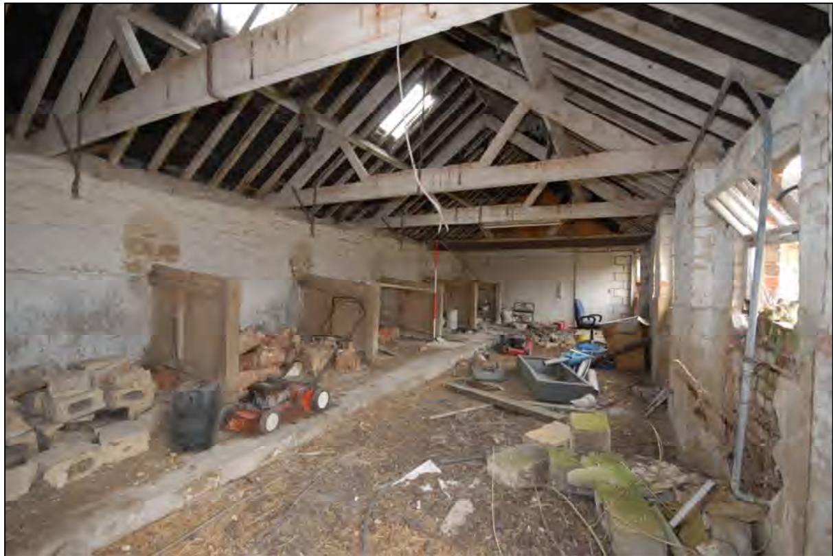
Image 31: Compartment C10, view looking south
