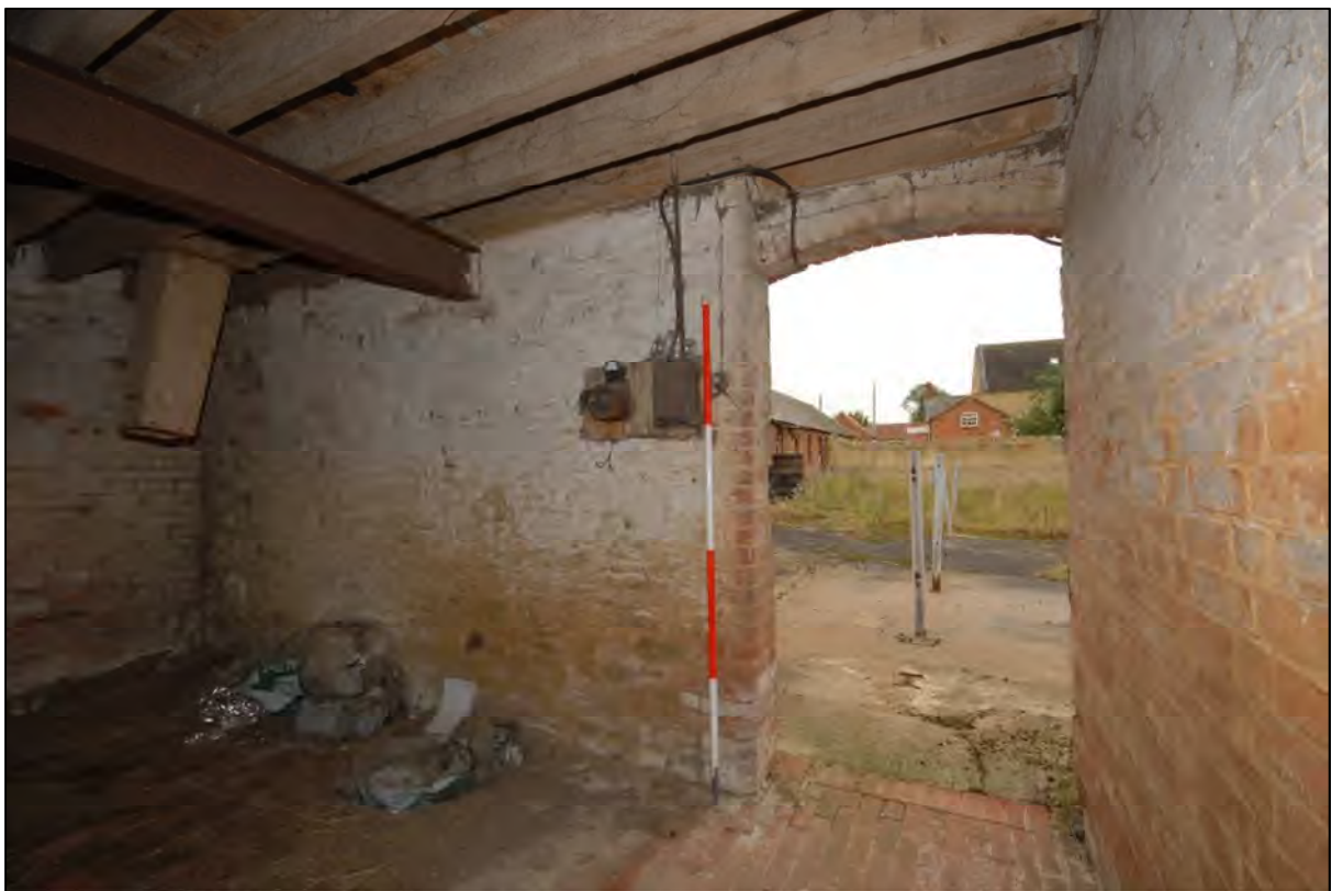
Image 22: Compartment C5, view looking south
