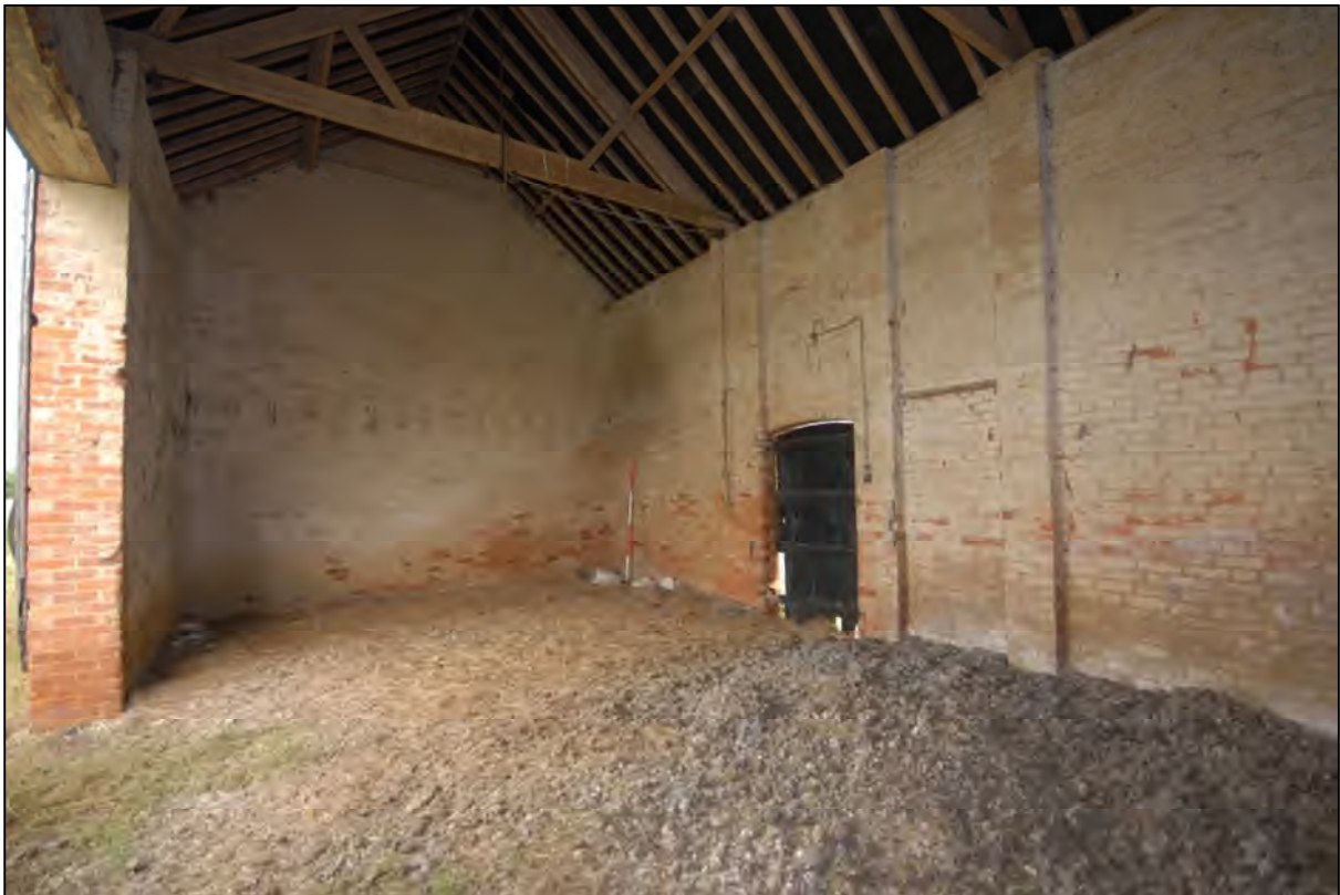
Image 20: Compartment C4, view looking east
