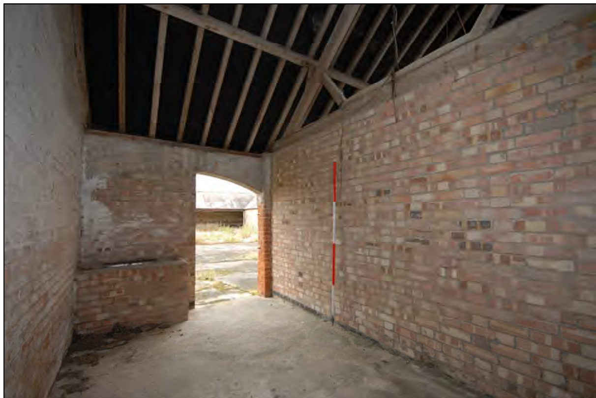
Image 30: Compartment C9, view looking west
