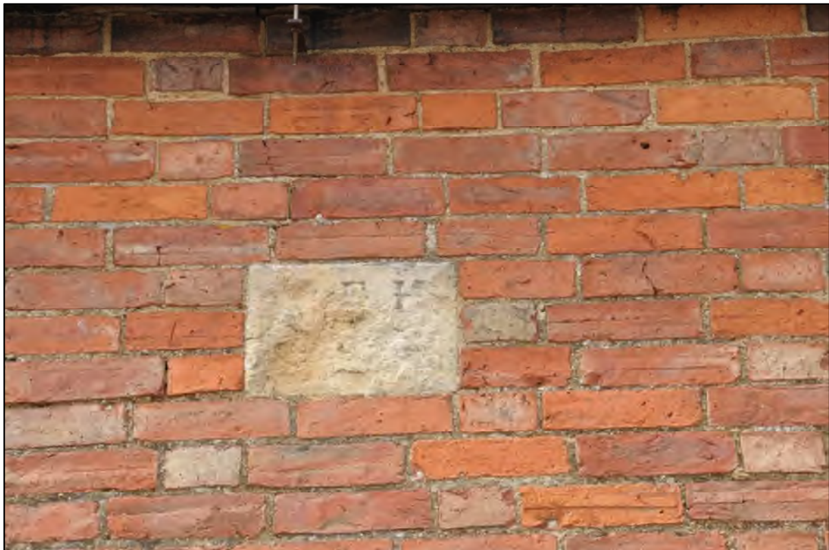
Image 2: Brickwork in south wall of north range
