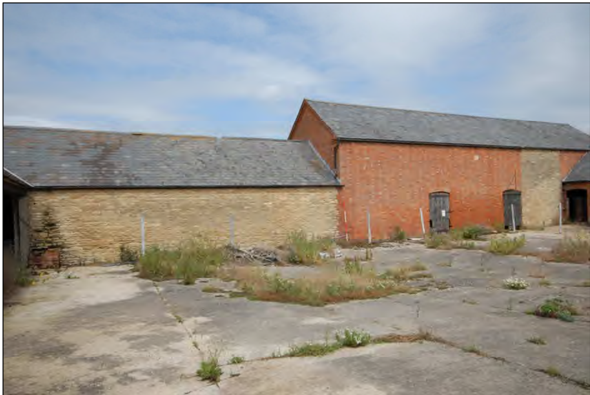
Image 16: Exterior view of north range, looking south-west
