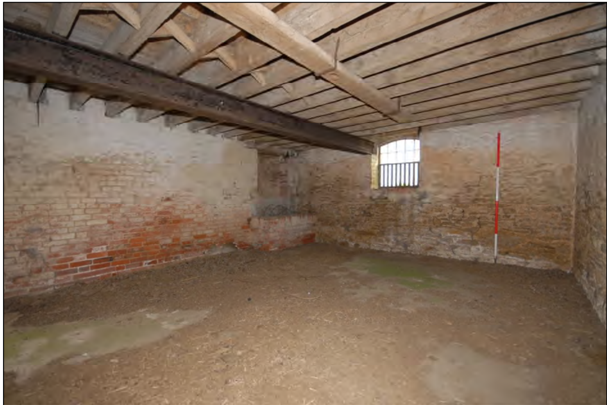
Image 23: Compartment C6, view looking north-west
