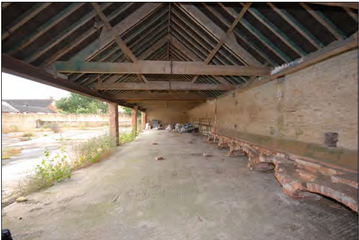
Image 12: Compartment C1, view looking south
