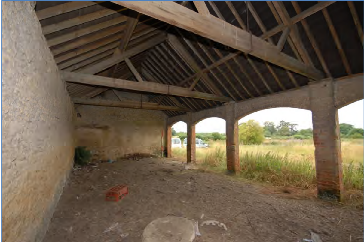
Image 17: Exterior view of north range, looking south-west Showing brick piers and arches supporting open side to the north
