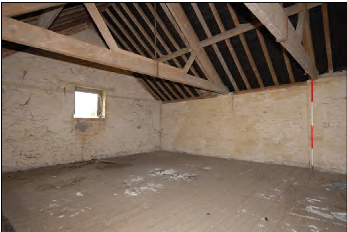
Image 26: Compartment C6, view looking south-east
