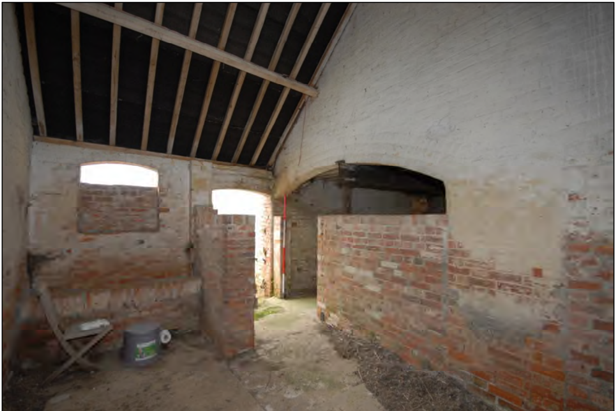
Image 29: Compartment C8, view looking west
