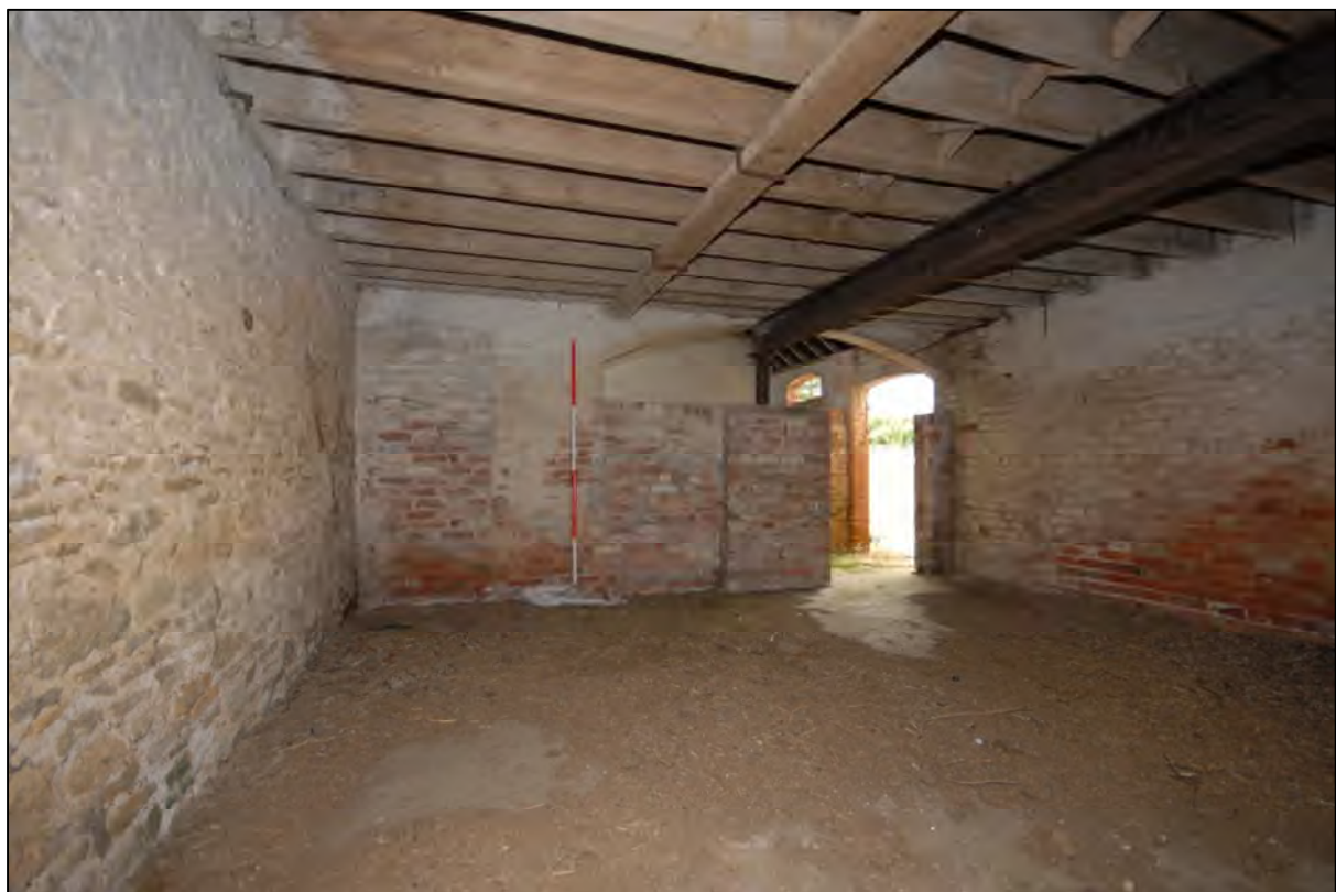
Image 24: Compartment C6, view looking south
