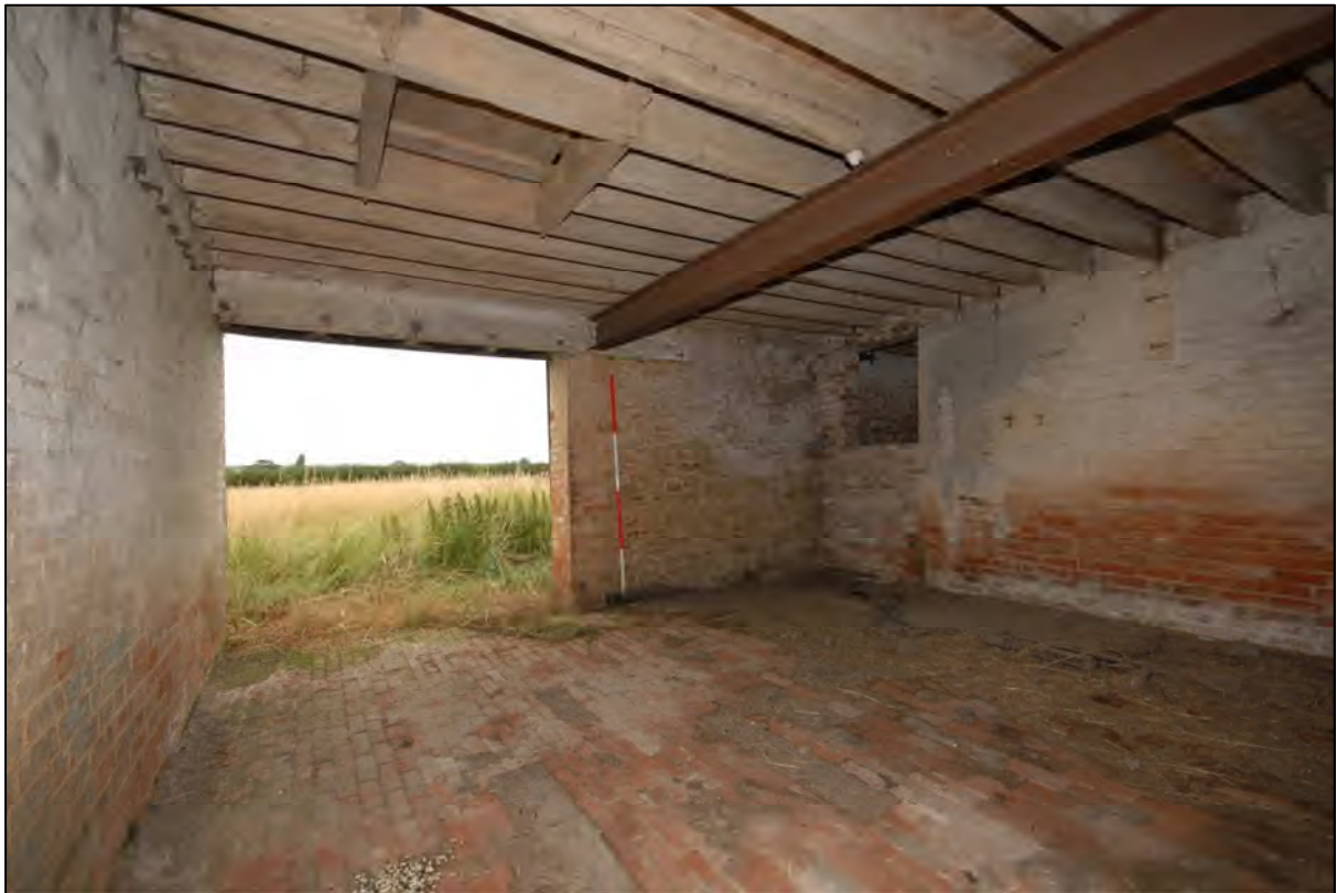
Image 21: Compartment C5, view looking north-east
