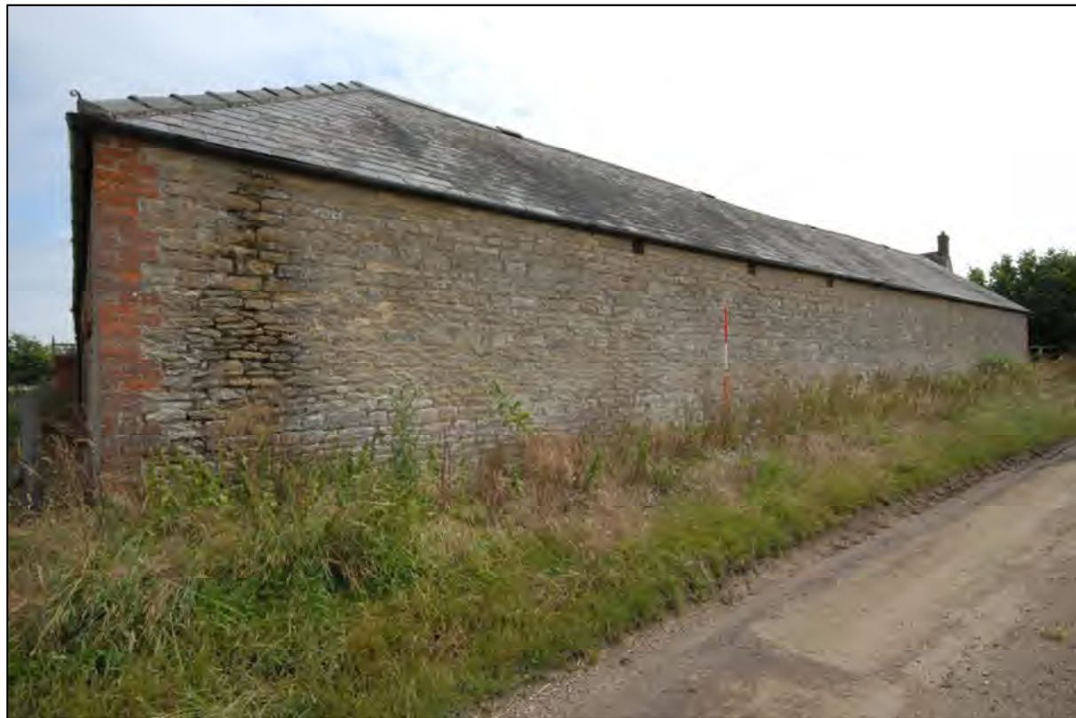
Image 10: Exterior of west range from the north-west Showing hipped roof at north end and blank limestone wall facing roadside
