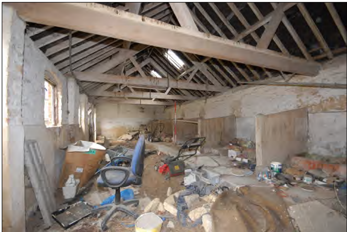
Image 32: Compartment C10, view looking north
