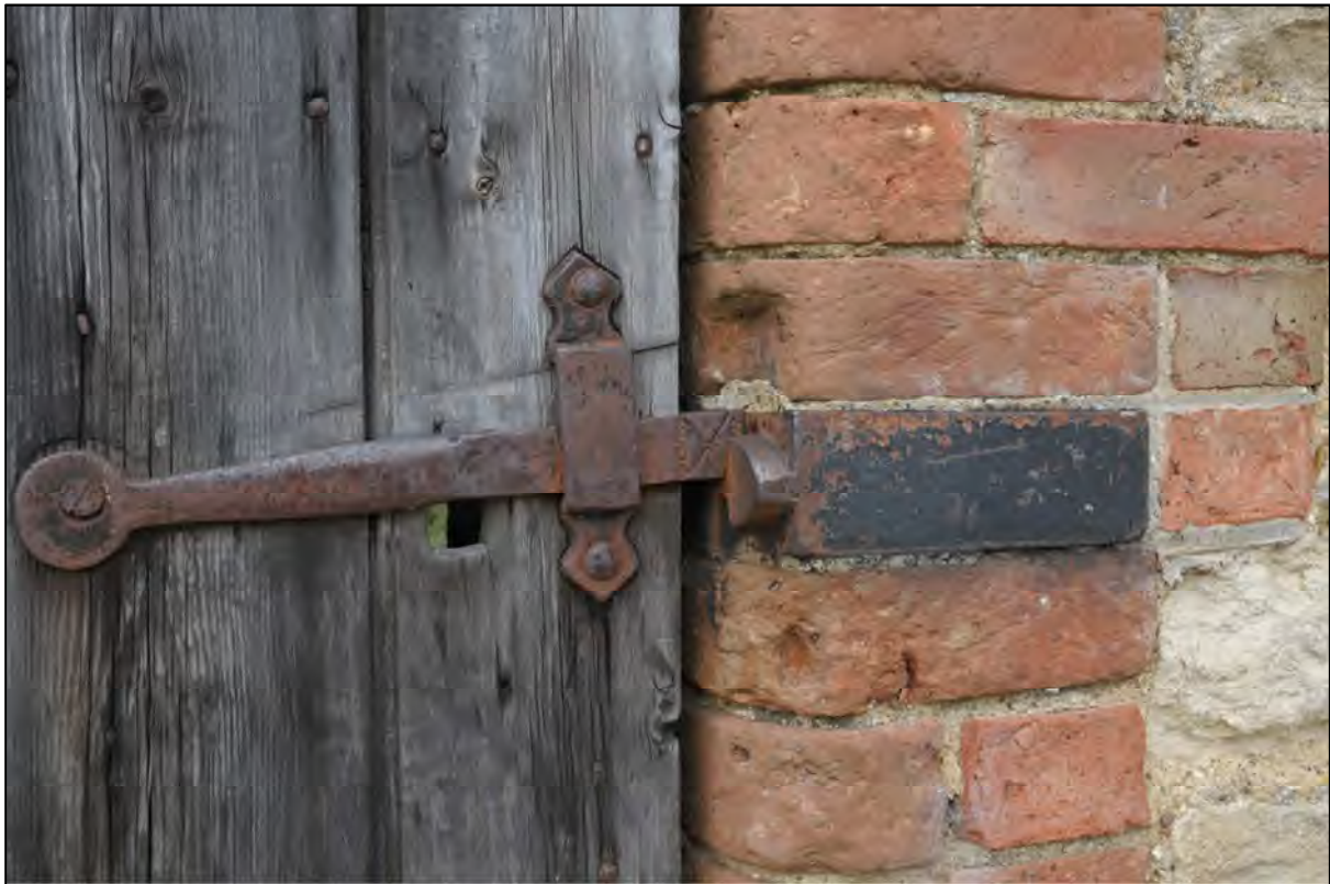
Image 7: Cast iron latch fastener and iron latch
