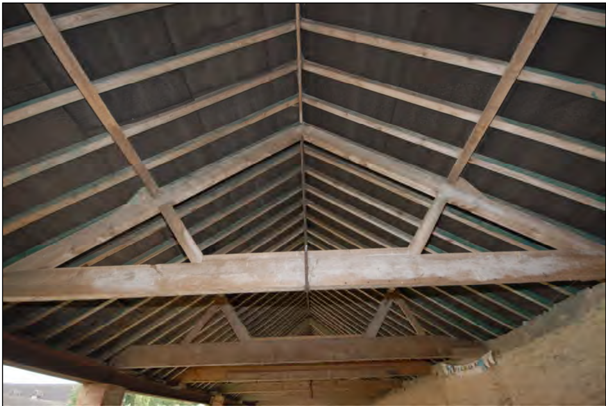
Image 8: Roof over compartment C1
