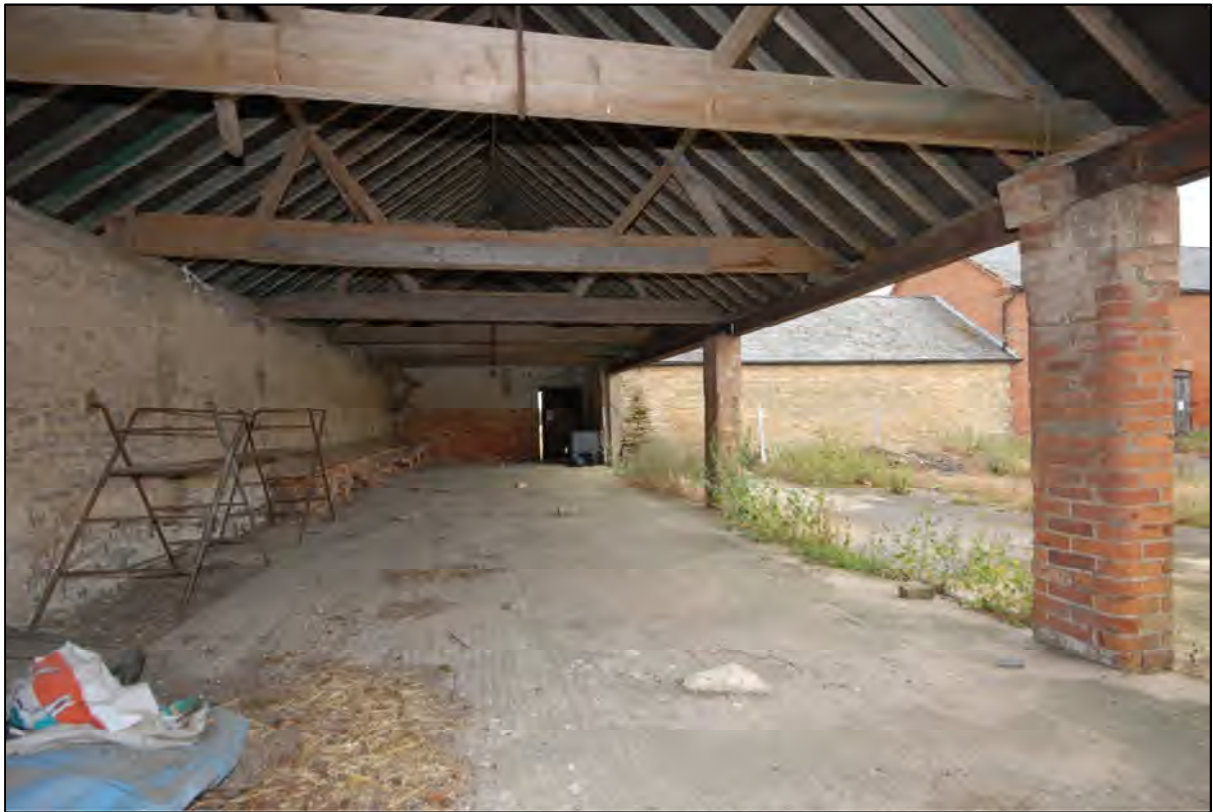
Image 11: Compartment C1, view looking north
