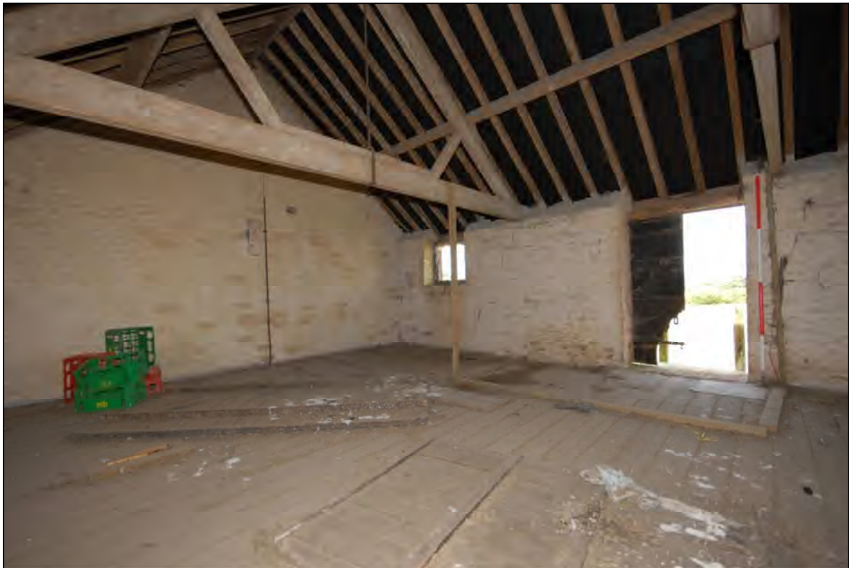
Image 25: Compartment C7, view looking north-west
