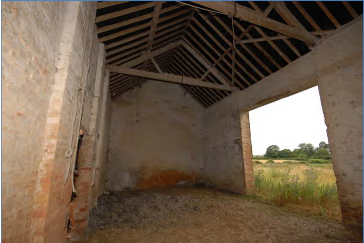
Image 19: Compartment C4, view looking west
