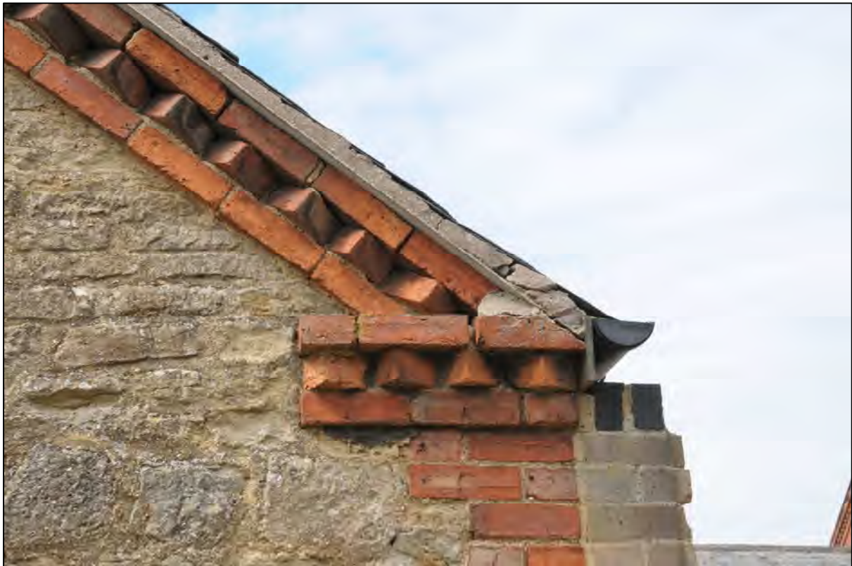
Image 3: Brickwork on south gable end of west range Shows dogtooth detail used on gable ends
