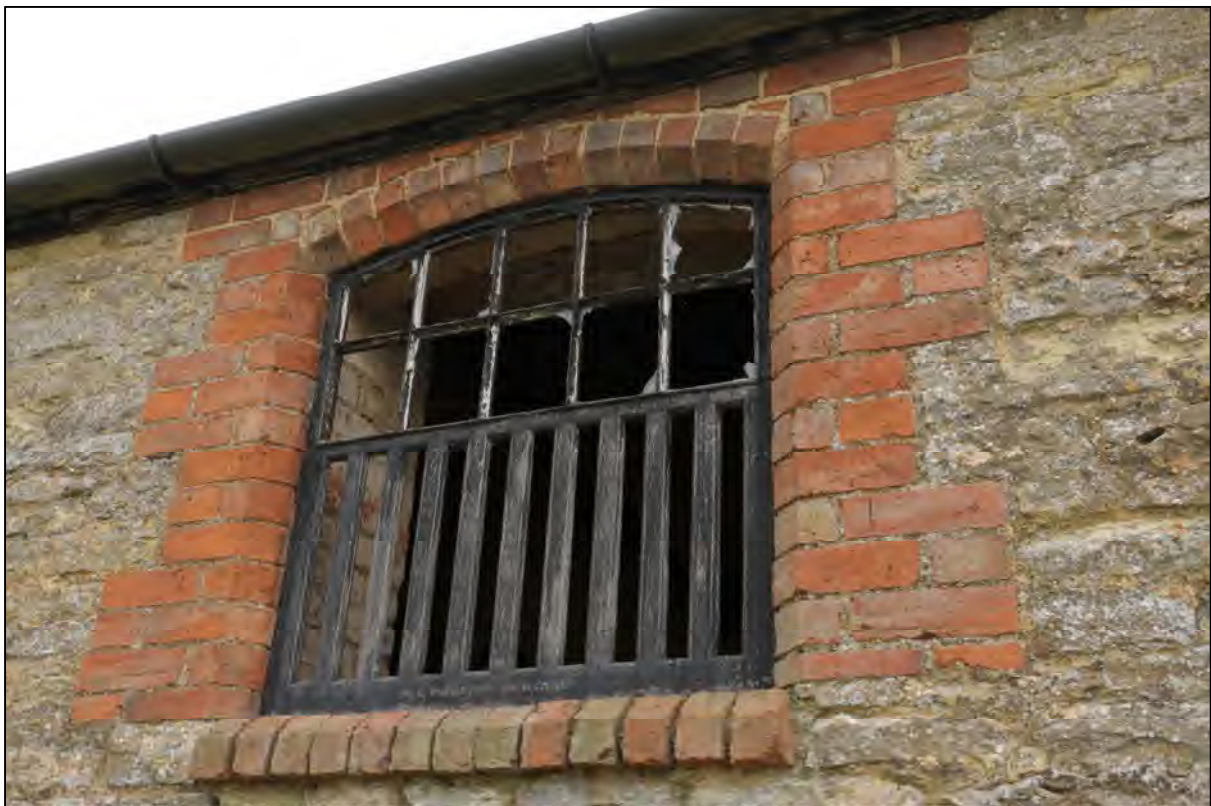
Image 6: Cast iron window in the north range
