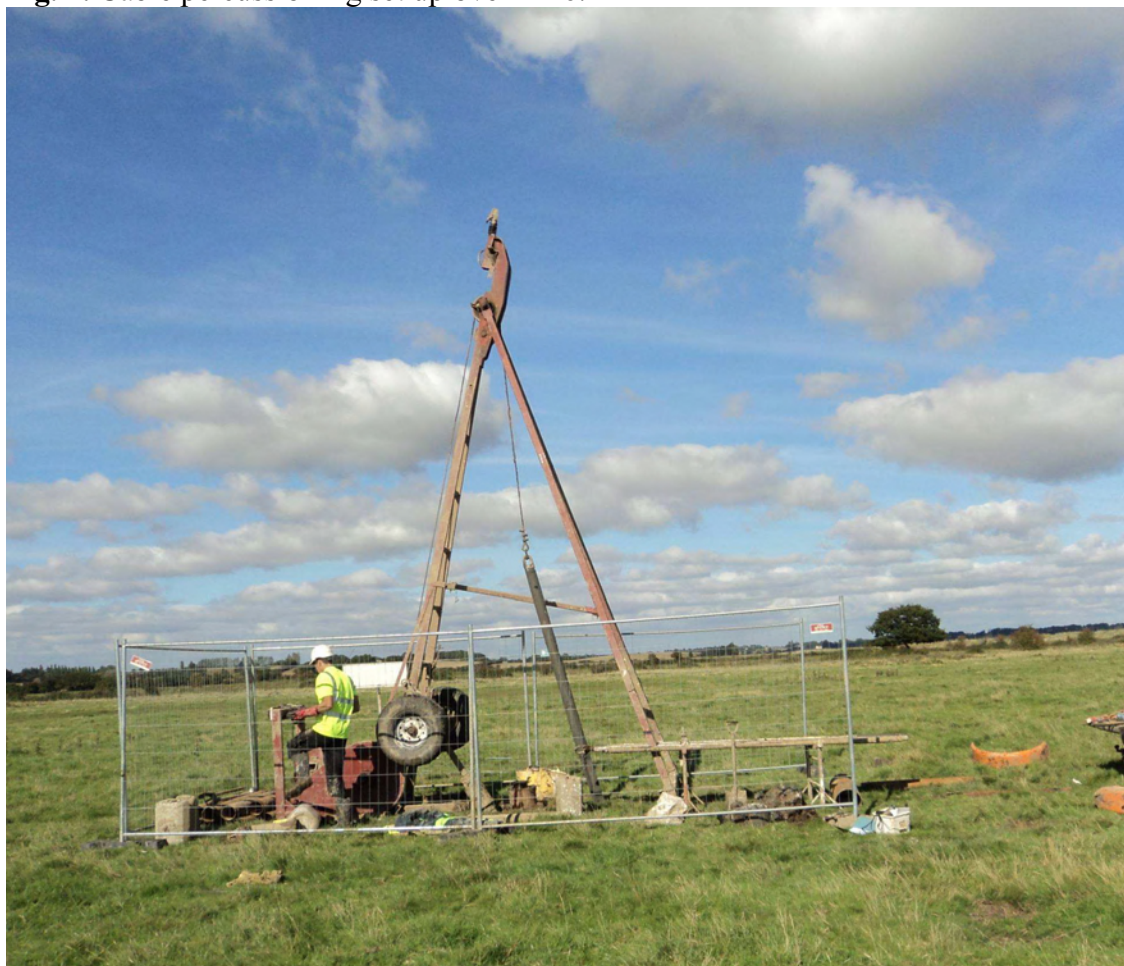
Fig. 2. Cable percussion rig set up over BH6.
