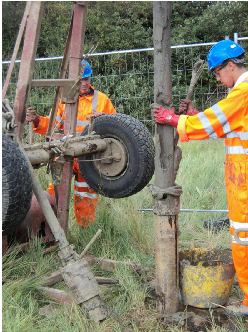
Fig. 3. Deposits being cleaned off the auger
