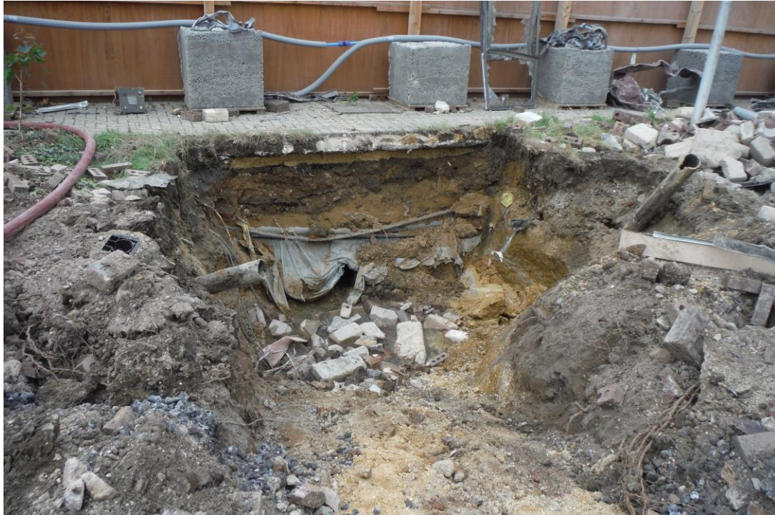
Figure 2: Make-up layers and river gravels exposed after removal of pile cap
