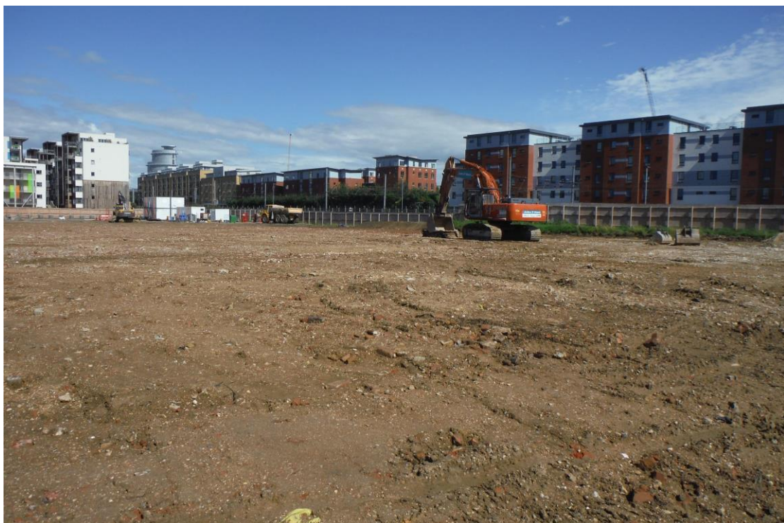
Figure 5: Graded surface after removal of Edinburgh Building, looking north-east
