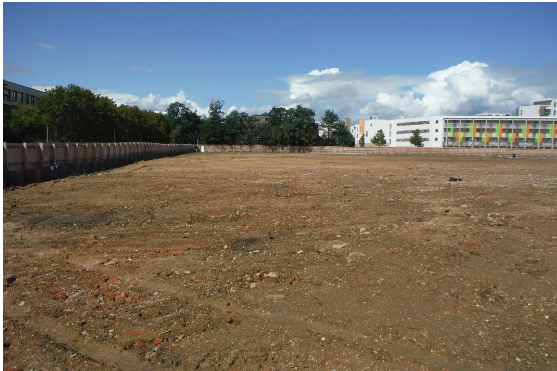
Figure 4: Graded surface after removal of Edinburgh Building, looking north
