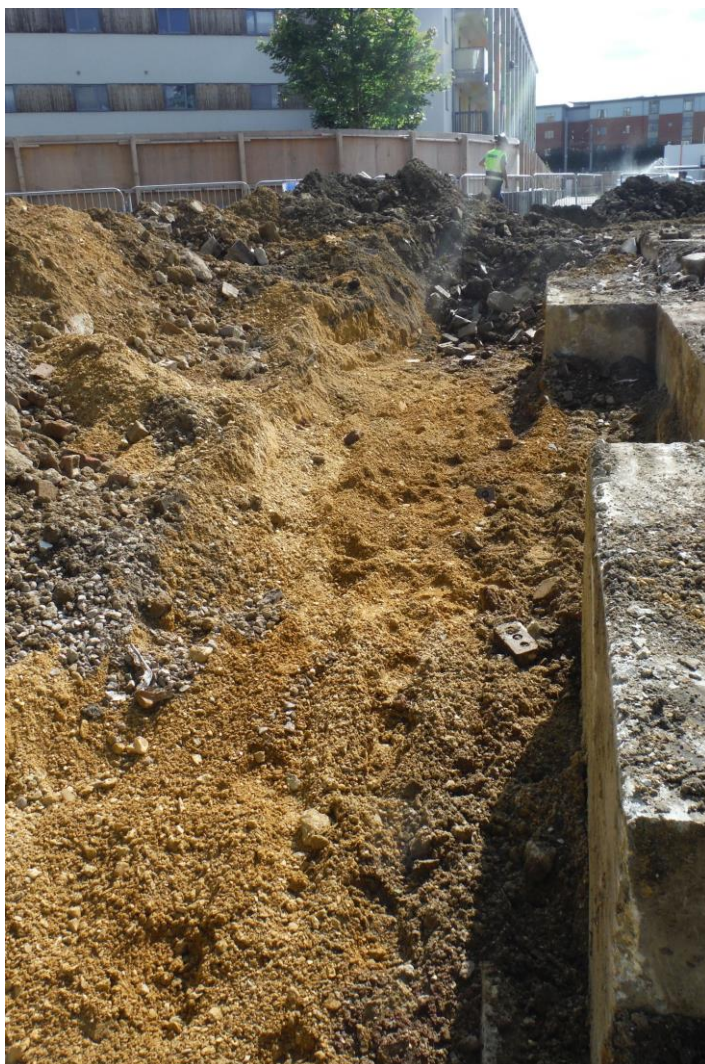
Figure 3: River gravels cut through by ring beam
