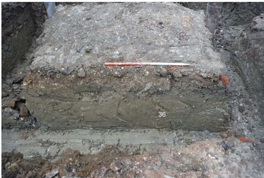
Figure 10: Natural deposits (36) beneath thin layer of overburden in the north-west corner of the building, looking north
