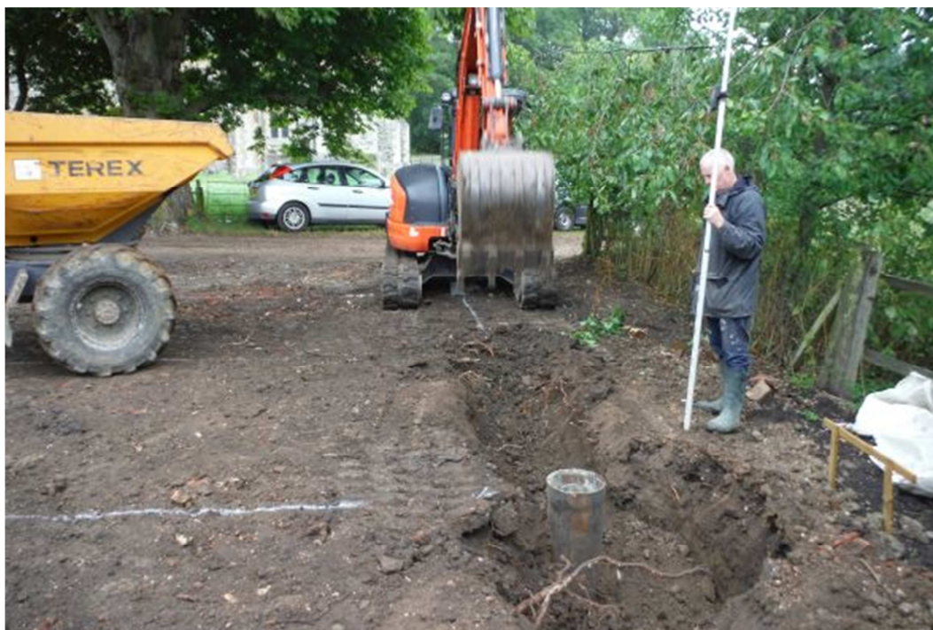
Figure 5: Start of excavation of footings, east side of building
