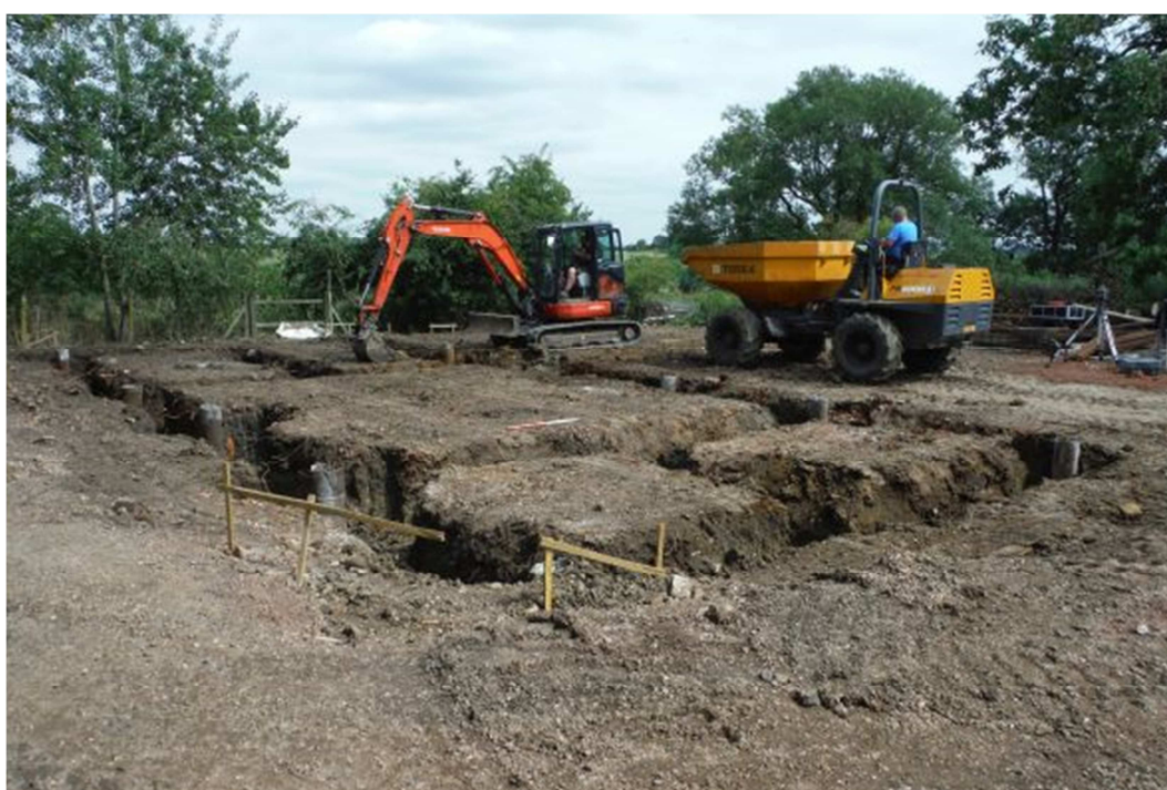
Figure 12: General view of the site after excavation of footings, looking south-east
