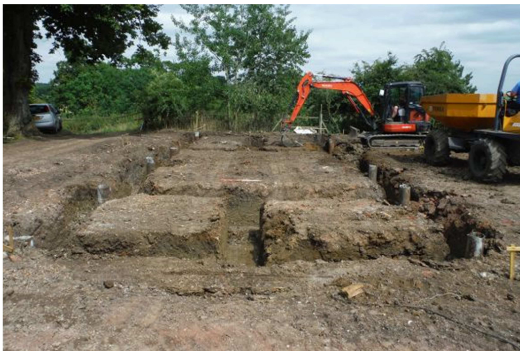
Figure 11: General view of the site after excavation of footings, looking east
