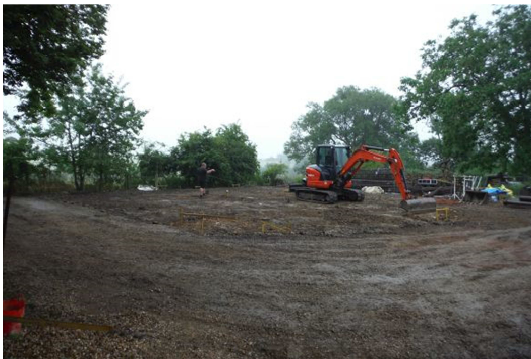
Figure 3: General view of the site after clearance, looking south-east
