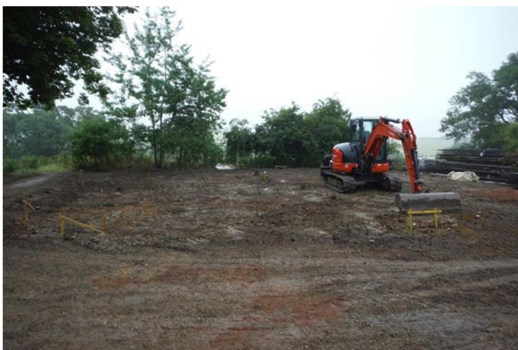
Figure 4: General view of the site after clearance, looking east
