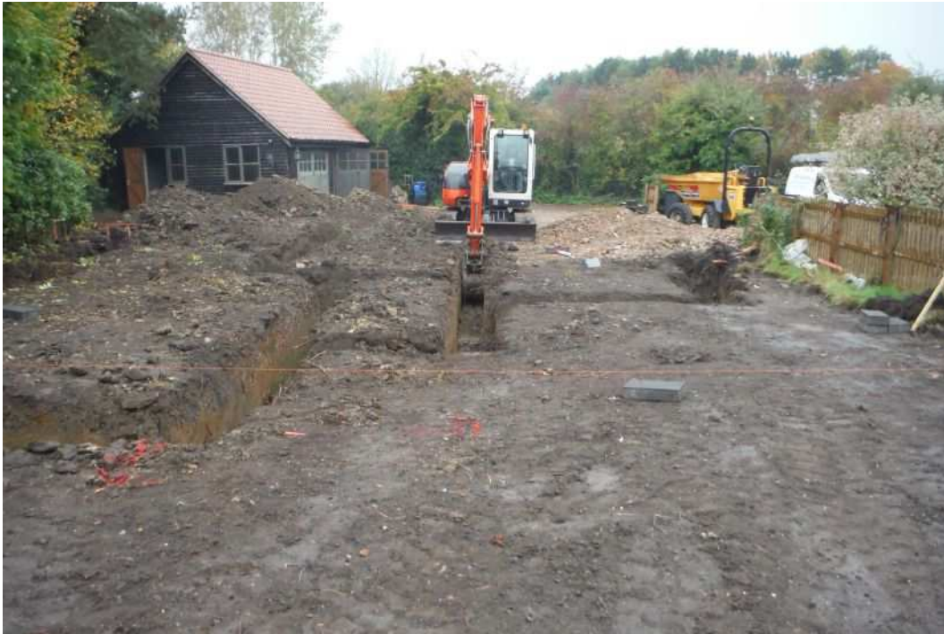
Figure 2: Excavating the footings trenches, looking north
