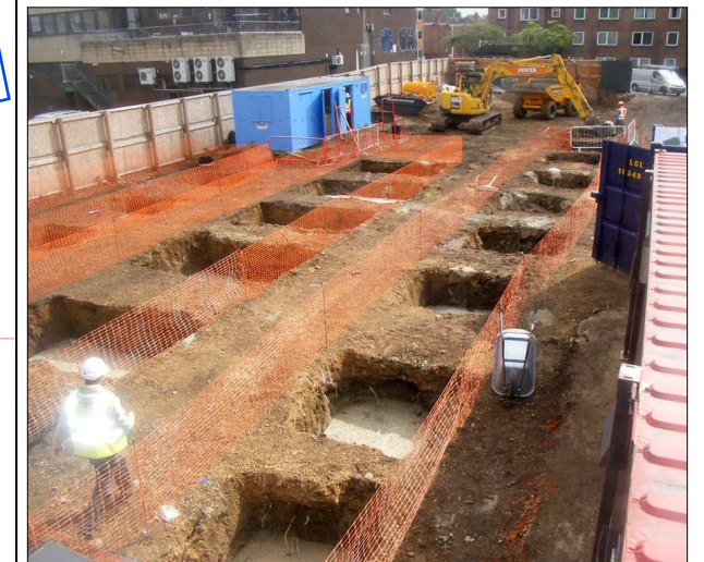
Photograph 2: Overview of foundation pits, looking north-east
