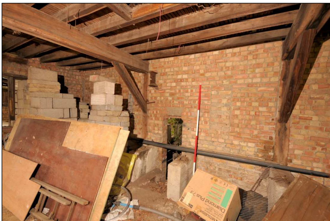
Image 12: Interior of cart shed, view looking south-east
