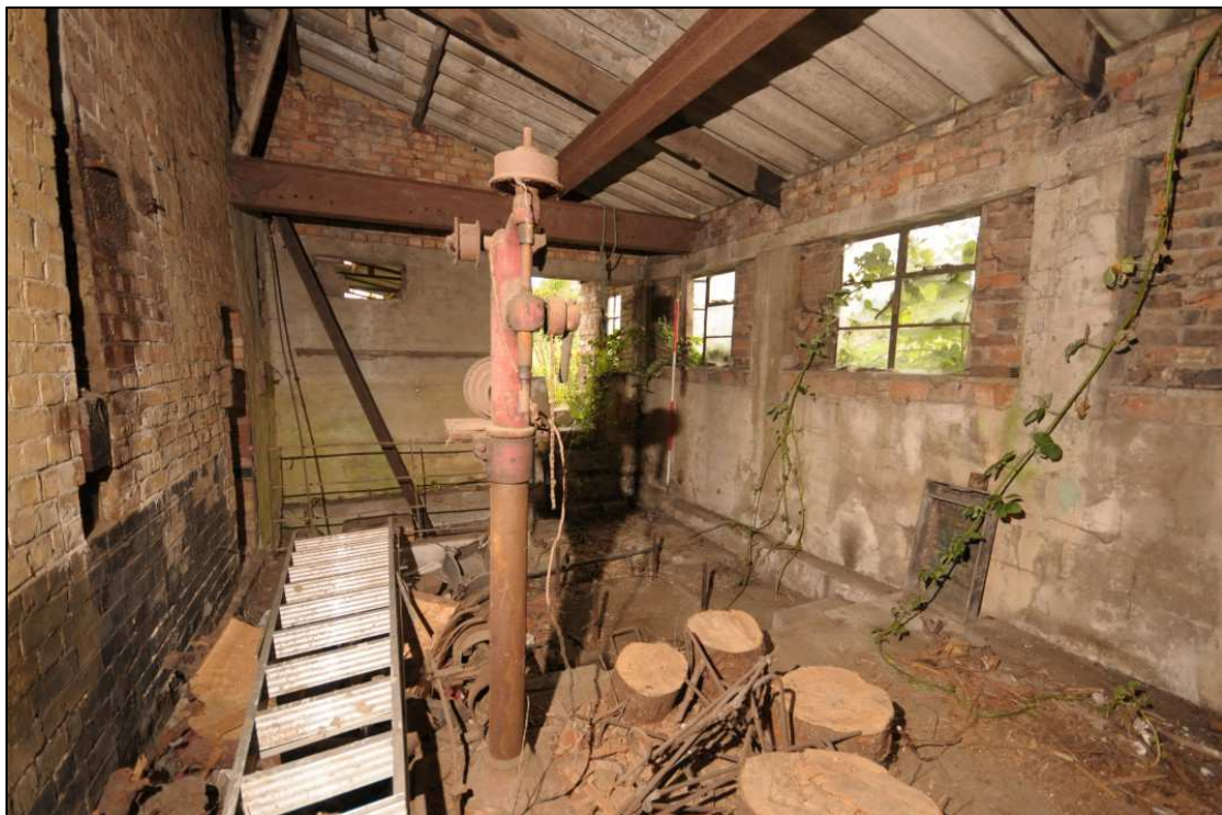
Image 20: Interior of south extension, view looking south-east
