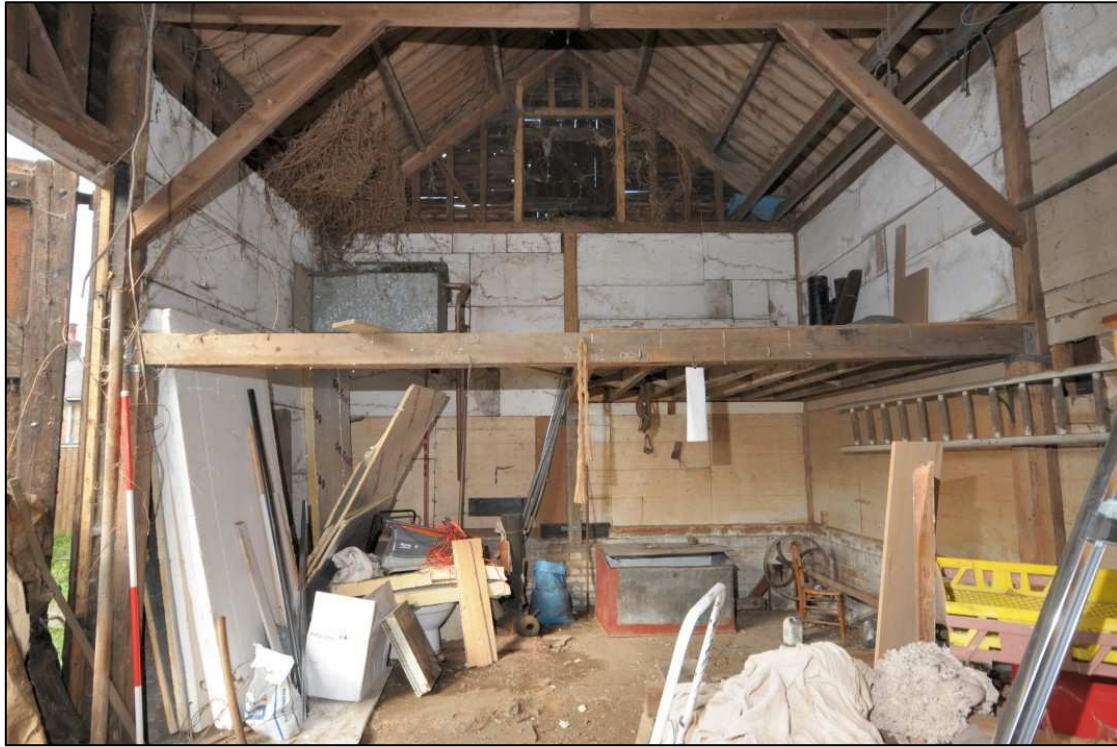
Image 25: Interior of barn, view looking west
