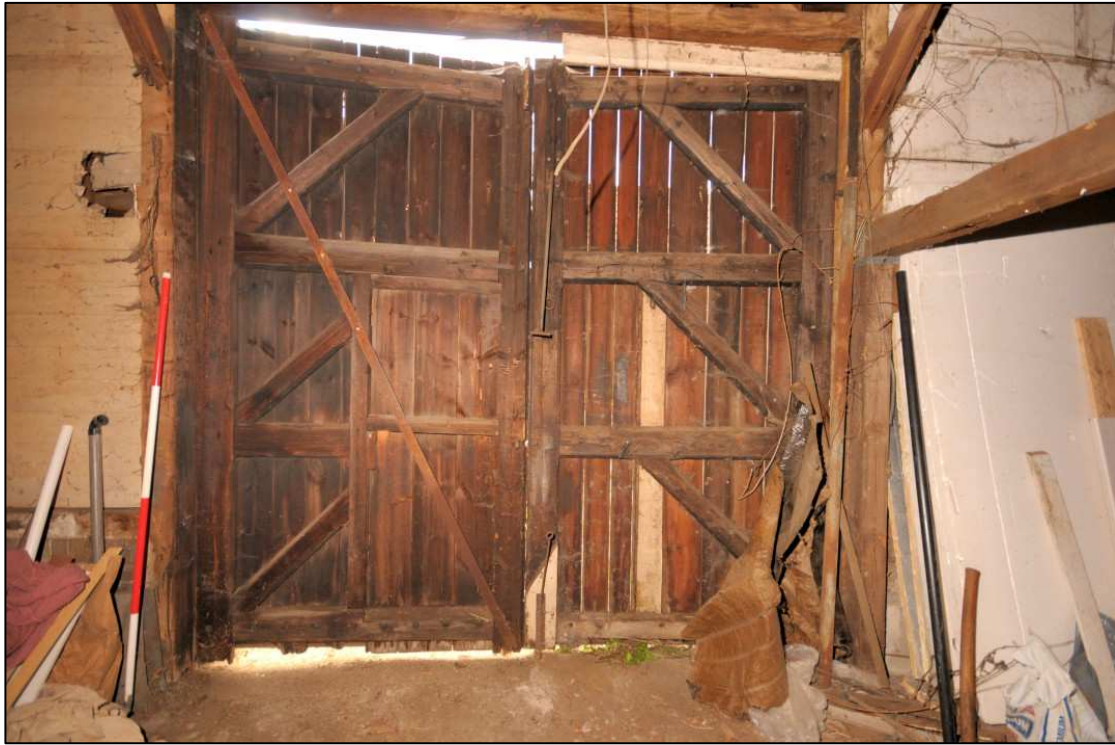
Image 31: Interior of barn, showing construction of double doors
