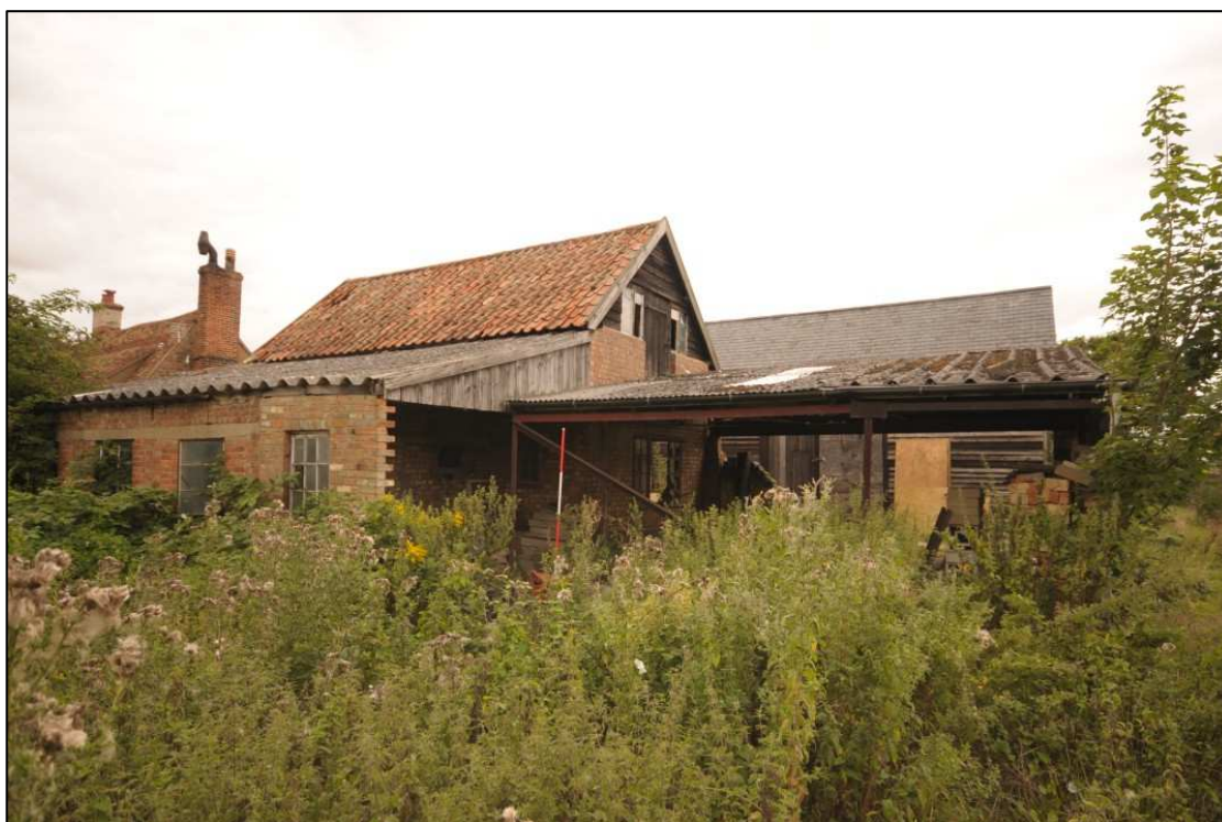
Image 5: Cart shed and extensions viewed looking north-west Shows open east extension to right and brick south extension to left
