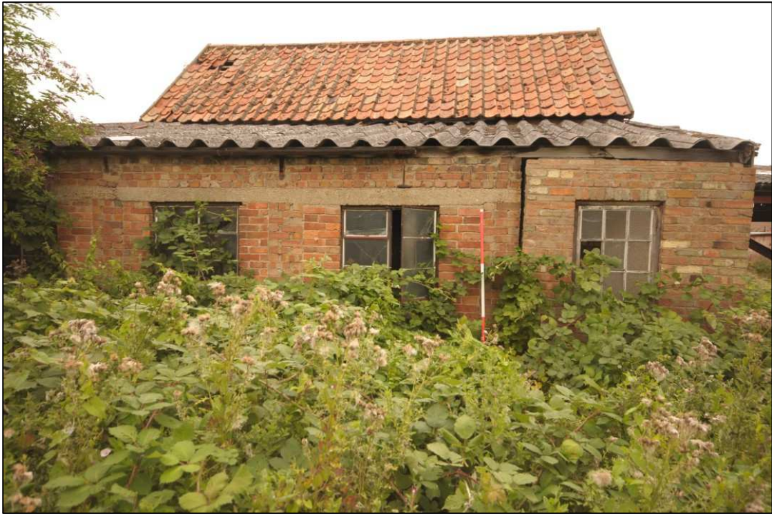
Image 7: South extension to cart shed, viewed looking north
