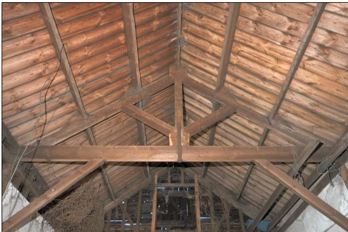
Image 30: Interior of barn, showing roof truss
