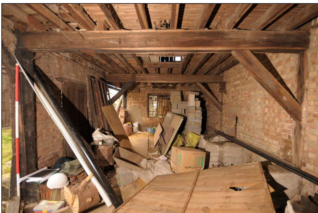
Image 10: Interior of cart shed, view looking east
