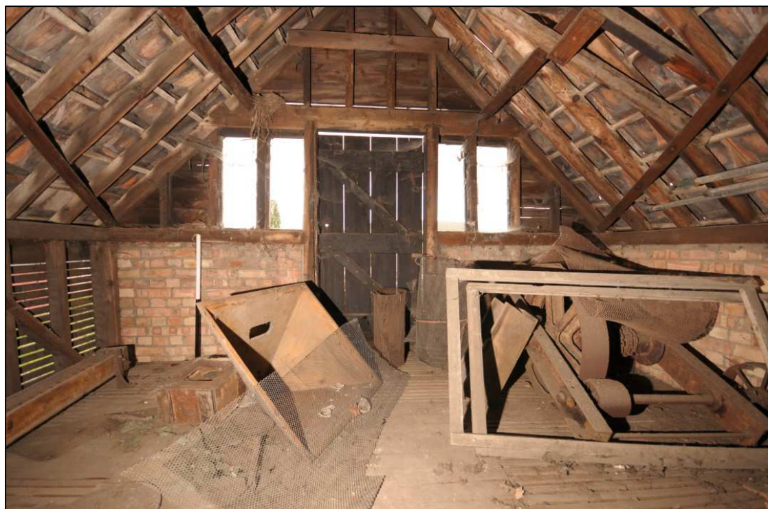
Image 14: Interior of cart shed loft, view looking east
