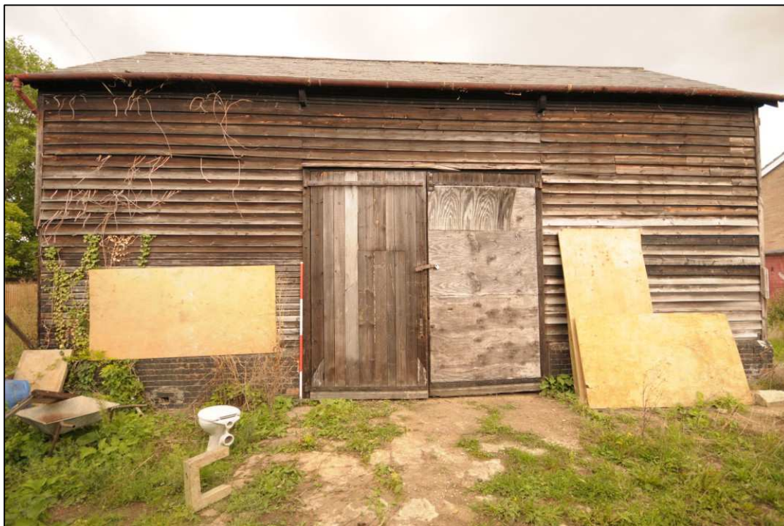
Image 21: South elevation of barn
