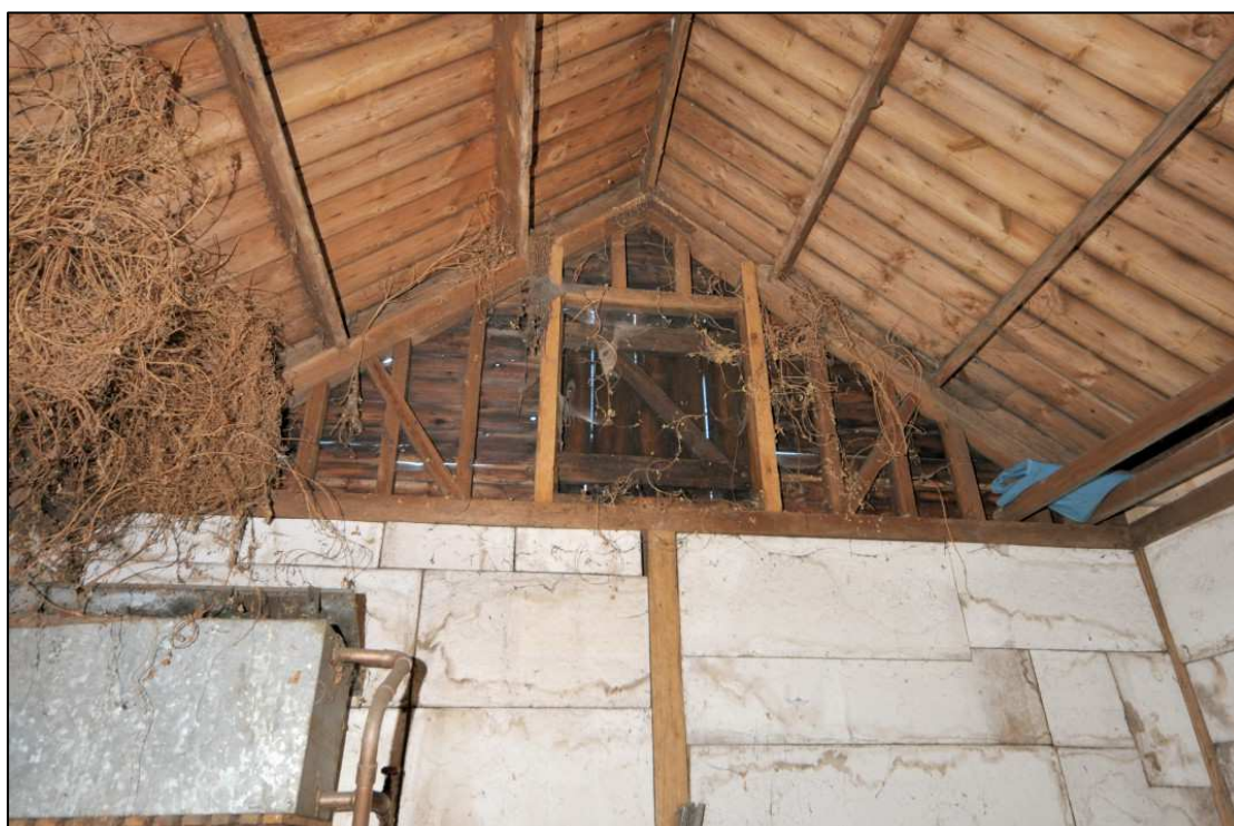
Image 28: Interior of barn showing west gable end
