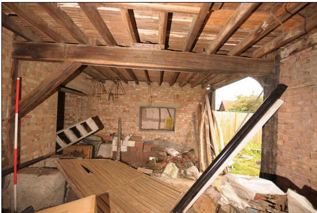
Image 9: Interior of cart shed, view looking west
