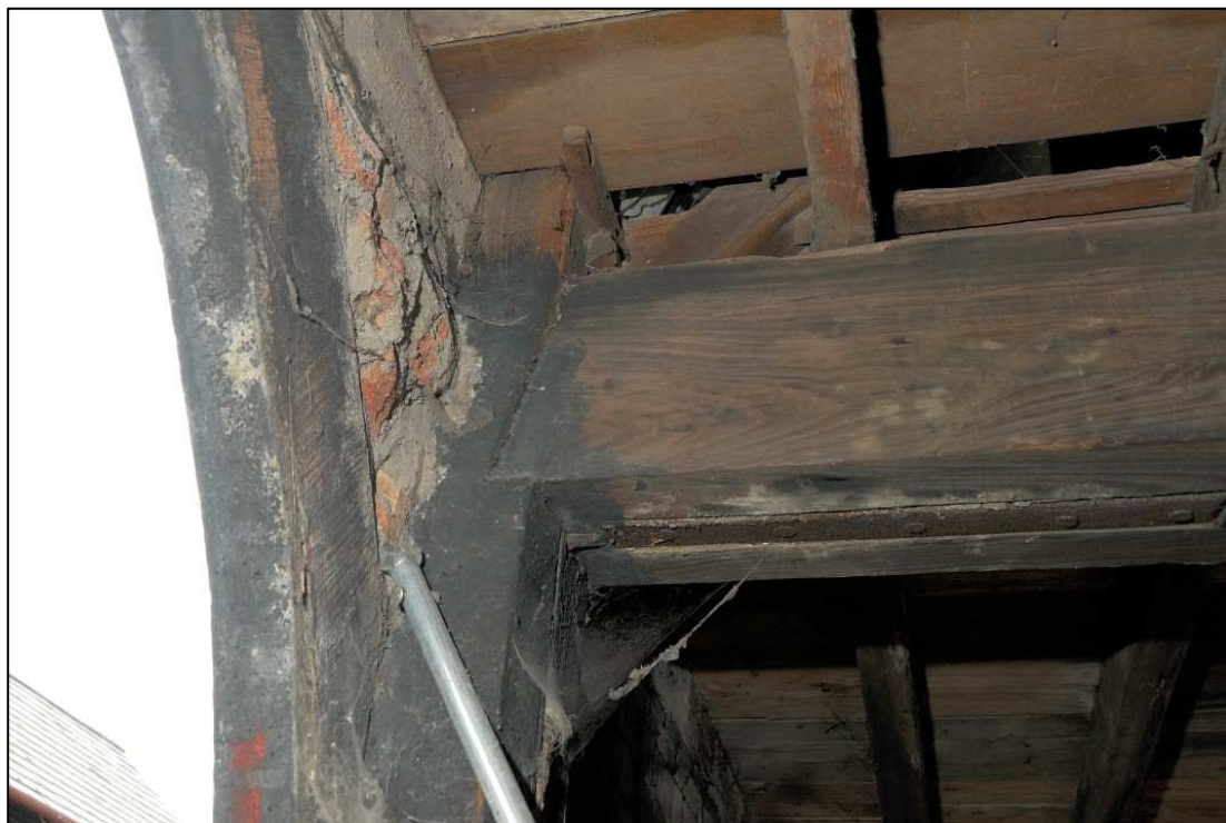
Image 11: Interior of cart shed, showing construction details
