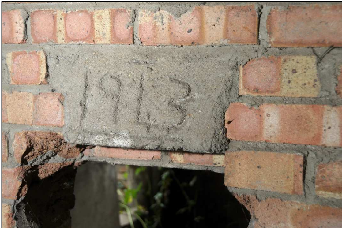
Image 13: Interior of cart shed, showing date
