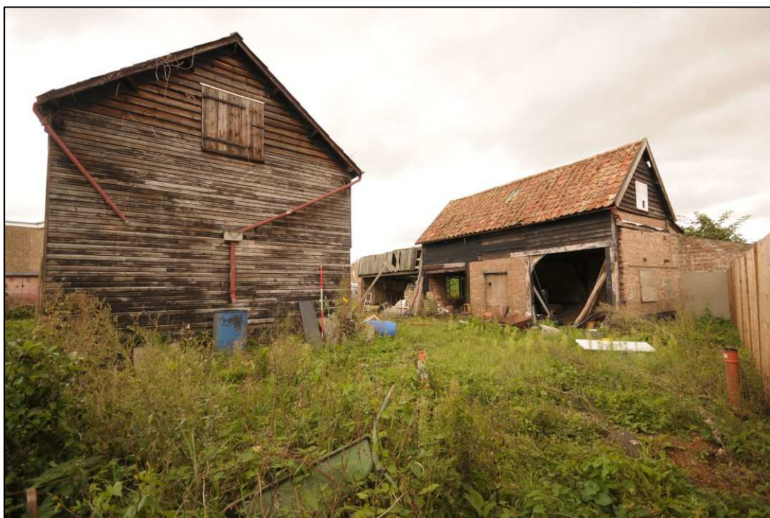
Image 2: Barn and cart shed viewed looking south-east
