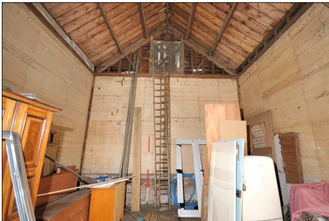
Image 27: Interior of barn, view looking east
