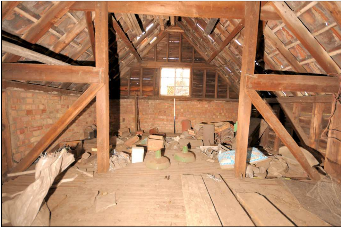
Image 15: Interior of cart shed loft, view looking west
