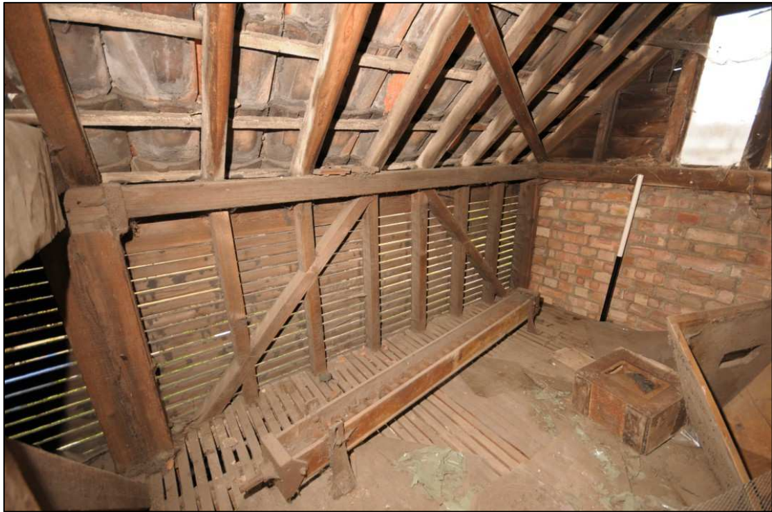
Image 17: Interior of cart shed loft, north-east corner
