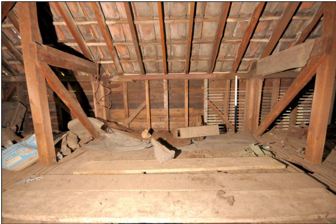
Image 16: Interior of cart shed loft, view looking north
