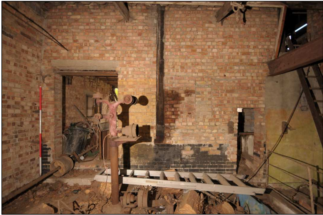
Image 19: Interior of south extension, view looking north
