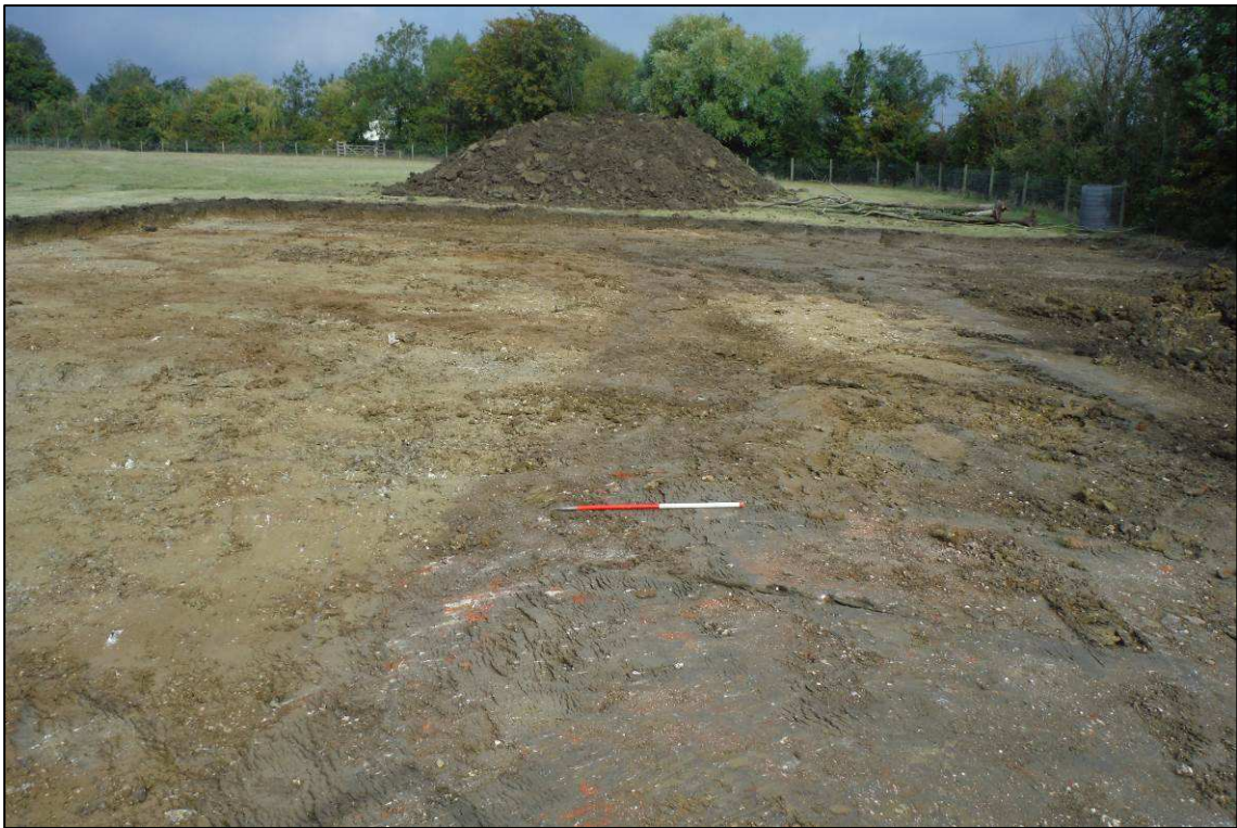
Plate 3: Modern features and overburden in area of manège, looking north
