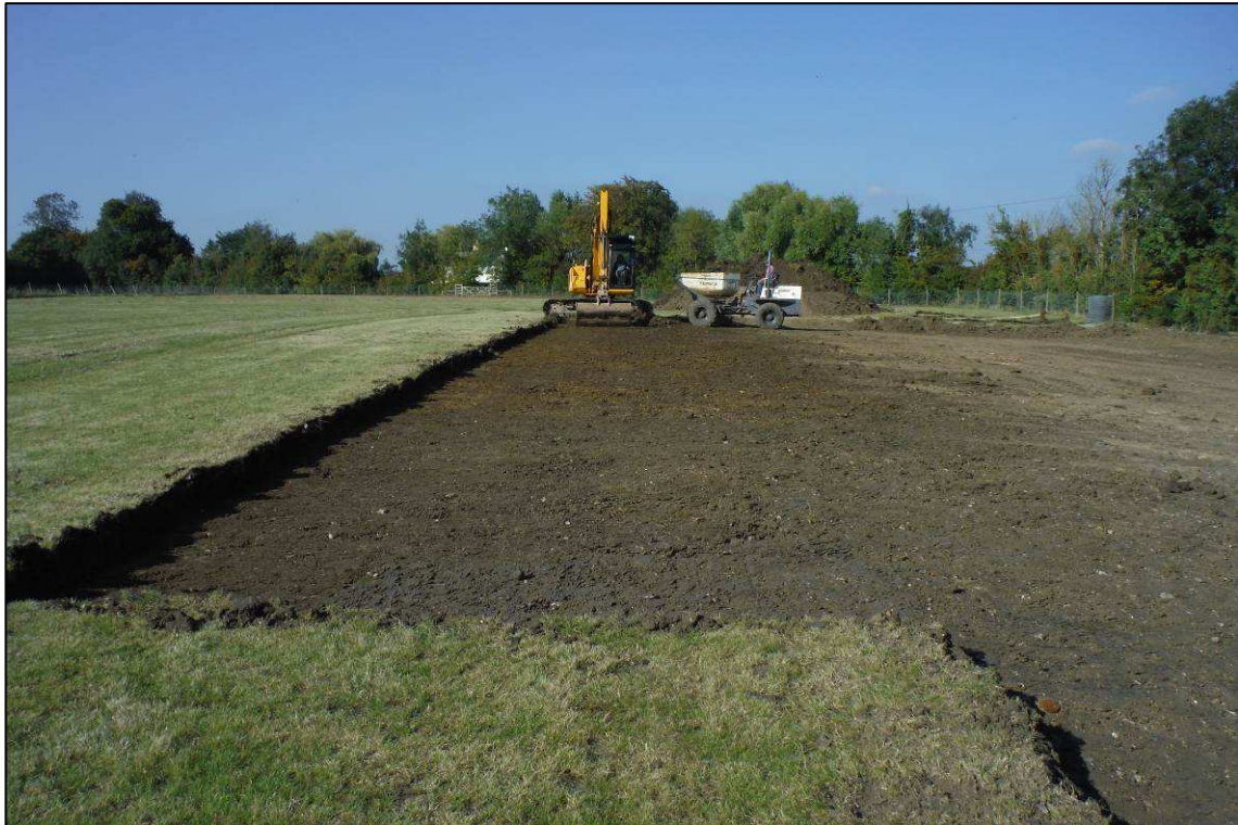
Plate 1: General view of topsoil strip of manège, looking north
