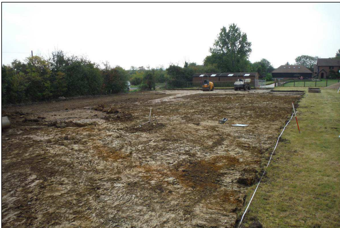
Plate 2: General view of stripped area for manège, looking south-east
