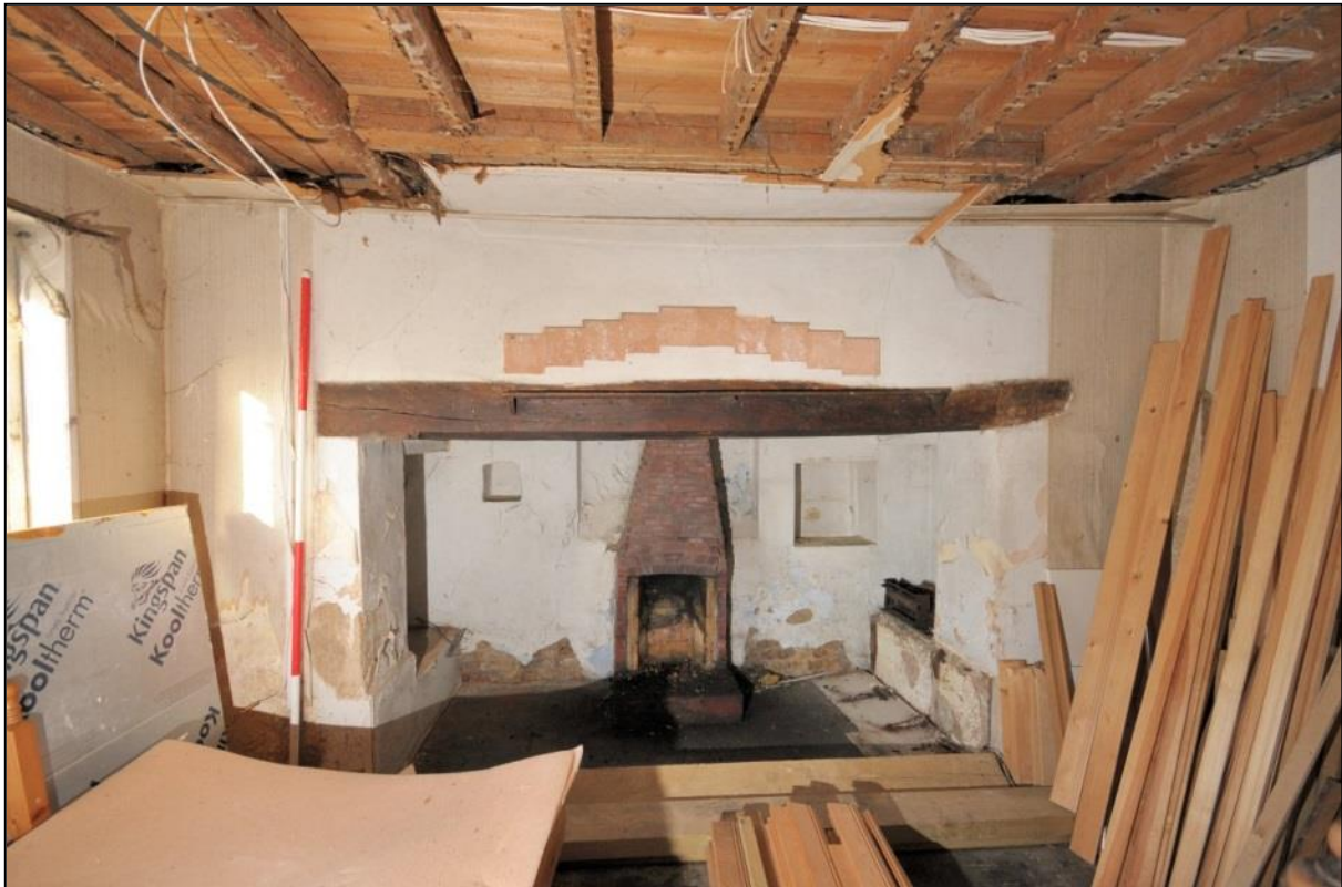
Image 9: Room G1, looking north-east
