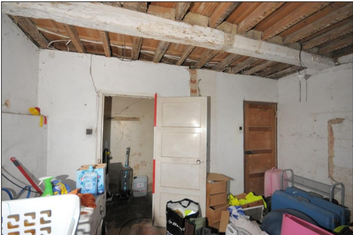
Image 36: Room G3, looking south-west (Scale 2m)
