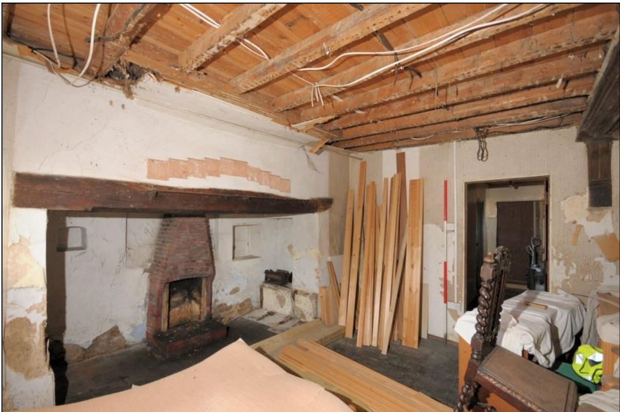
Image 8: Room G1, looking east
