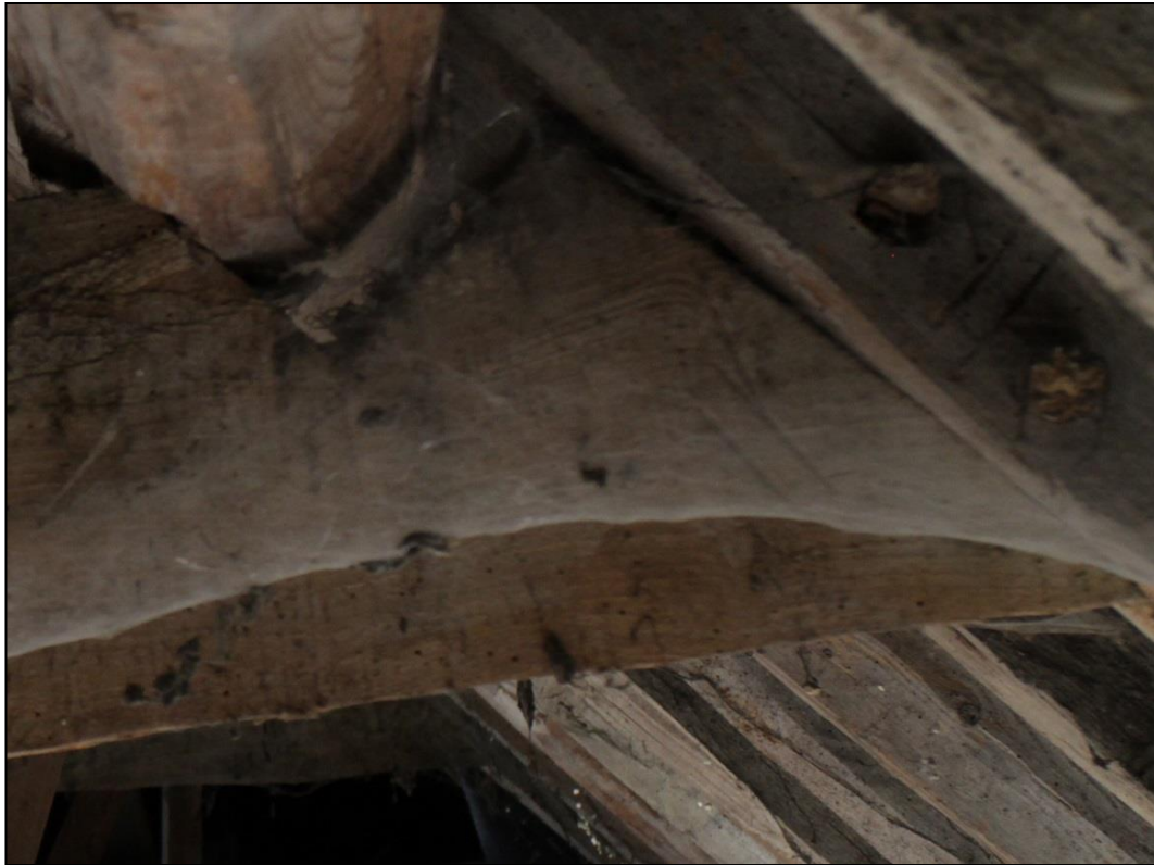
Image 33: Roof, detail of assembly marks
