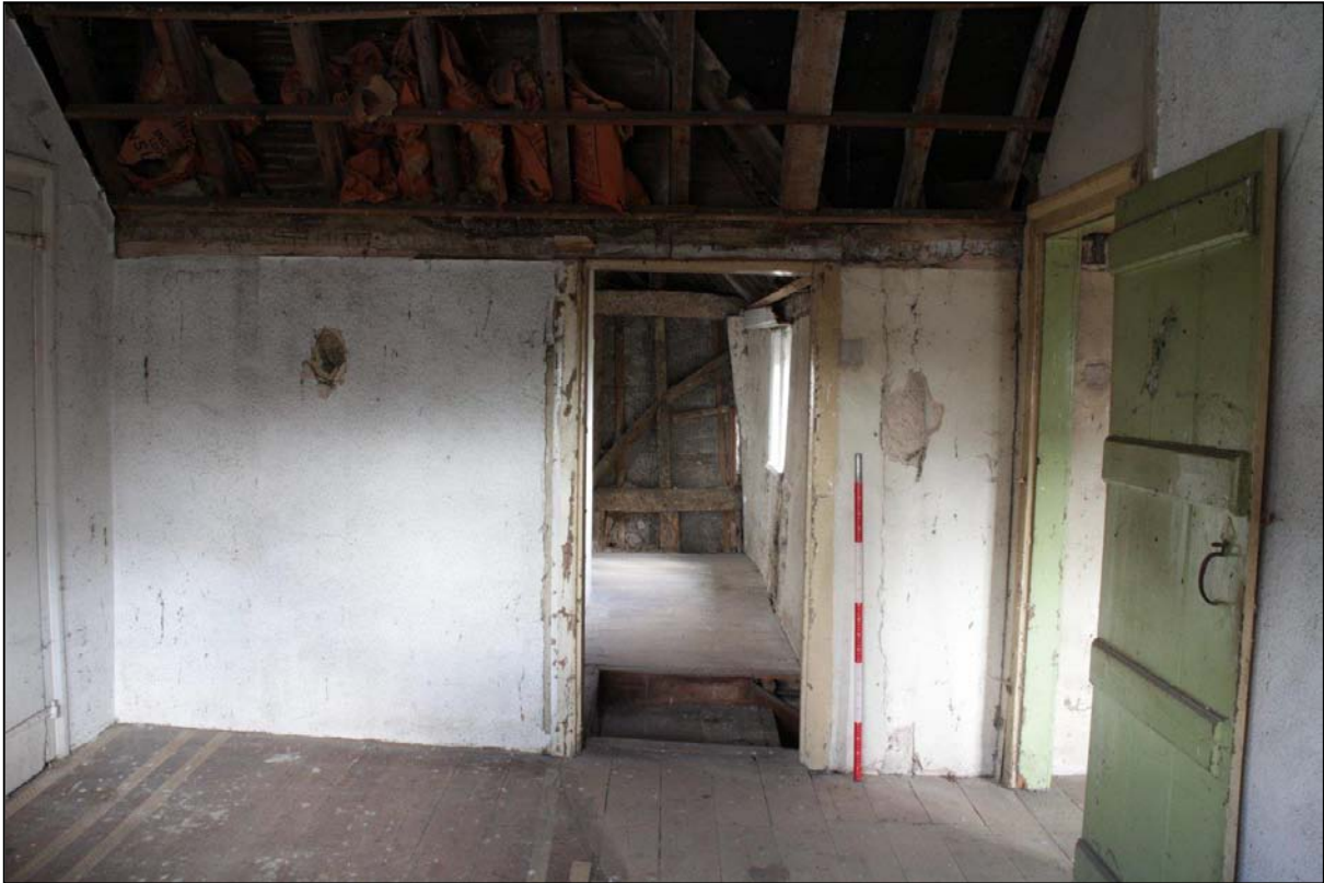
Image 17: Room F1, looking south-east
