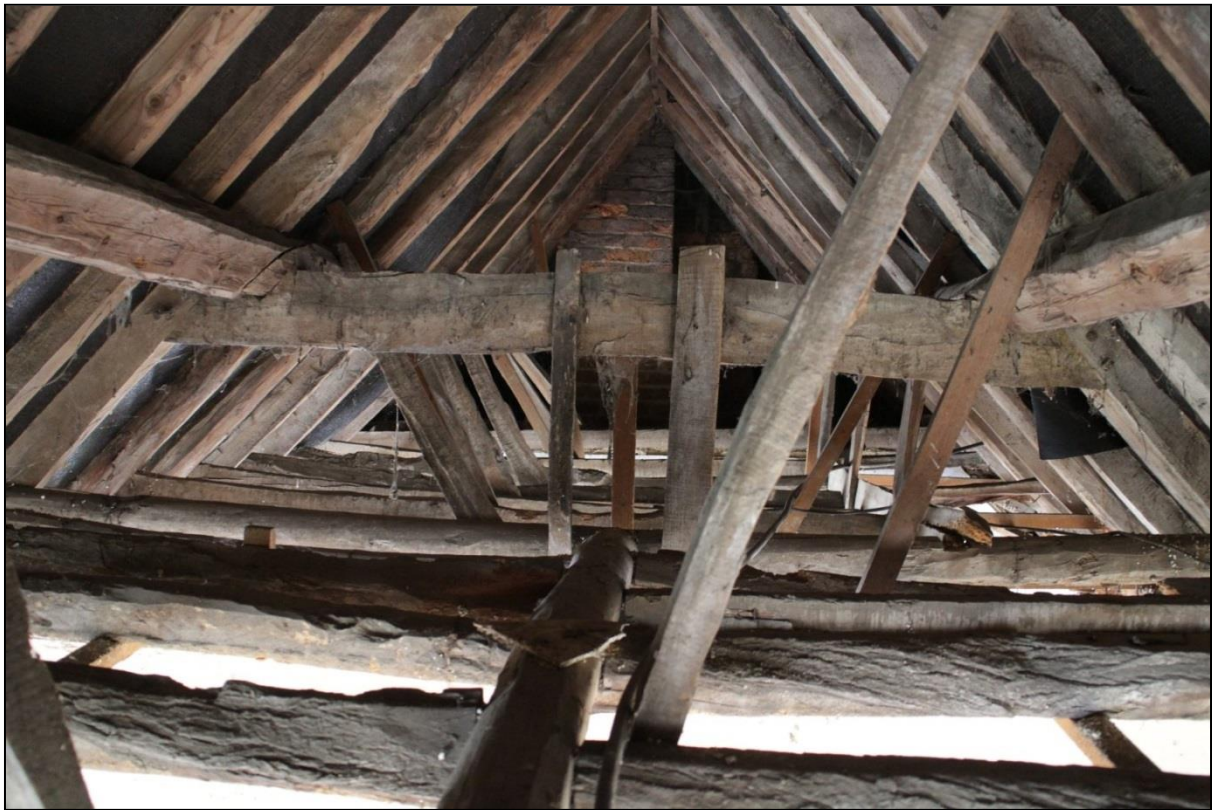
Image 31: Roof over main range, looking north-east
