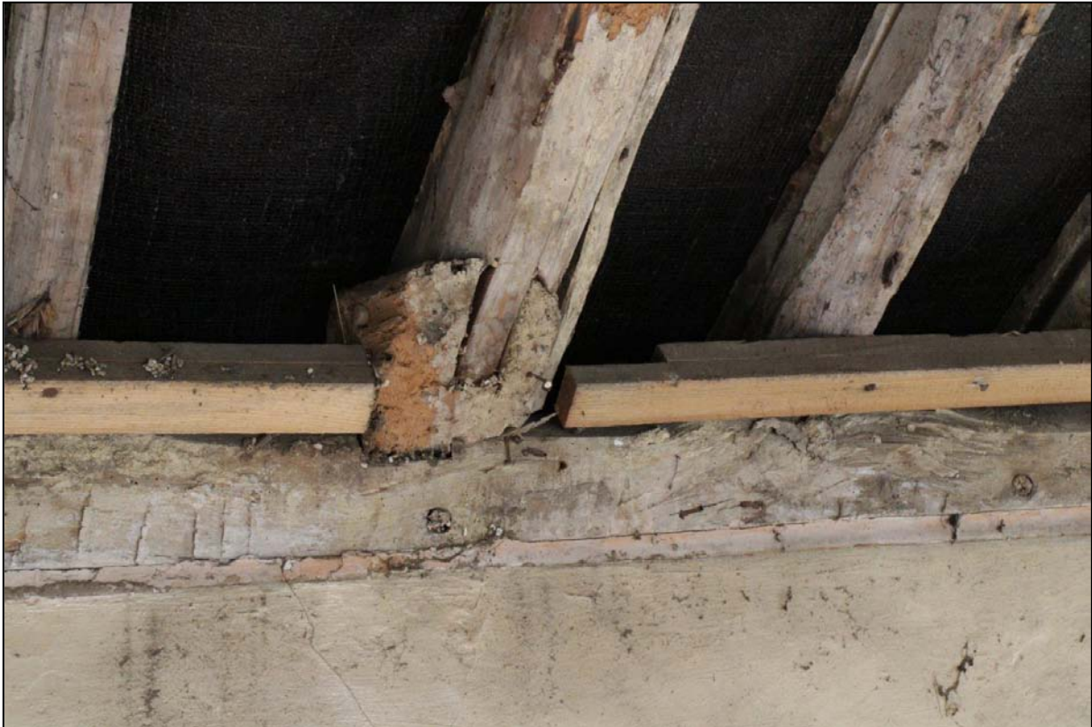
Image 29: Room F2, detail of tie beam and wall plate
