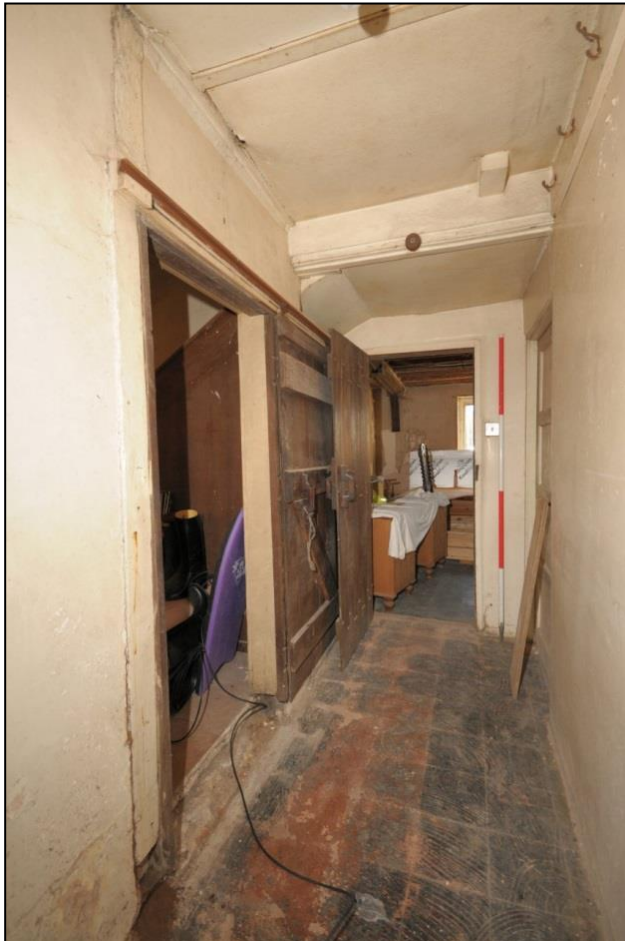
Image 38: Ground floor corridor
