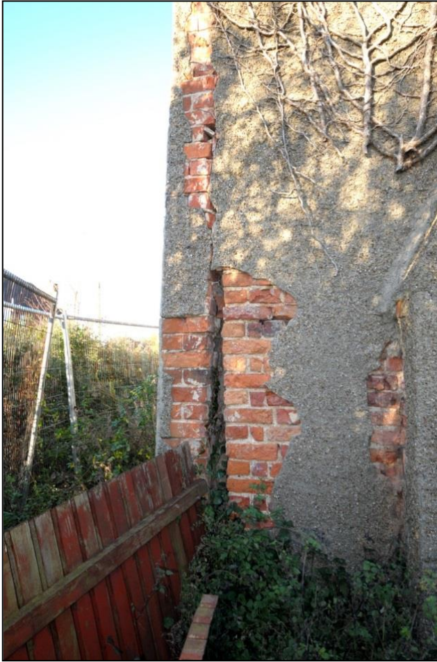
Image 5: Detail of south-west corner of building
