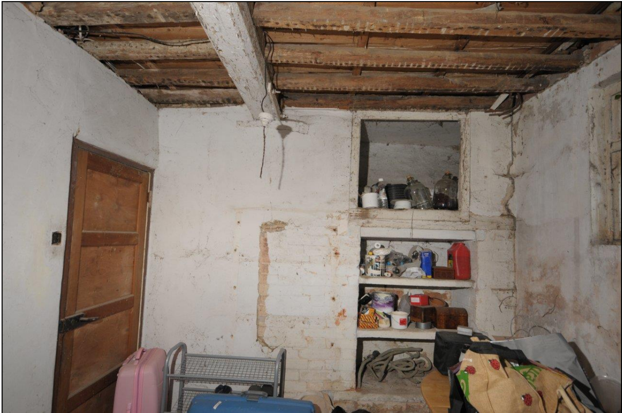
Image 37: Room F3, looking north-west
