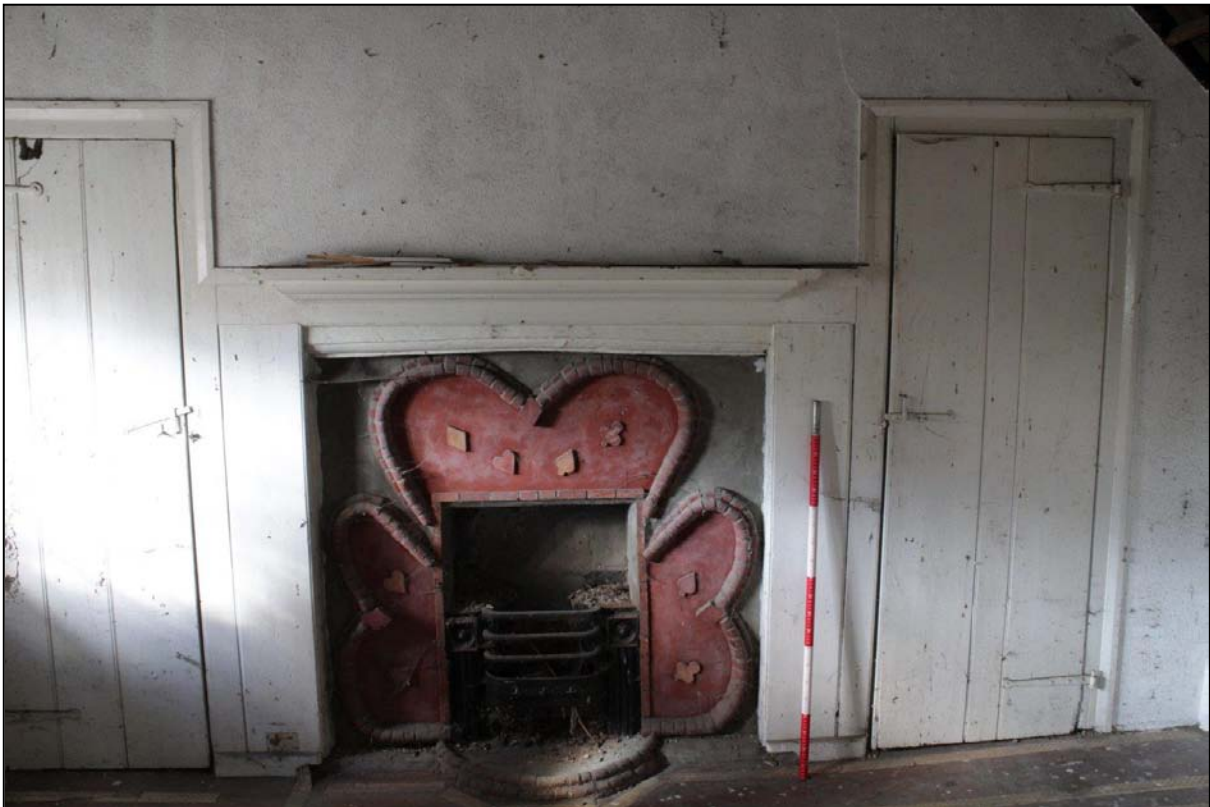
Image 18: Room F1, fireplace and doors in north-east wall
