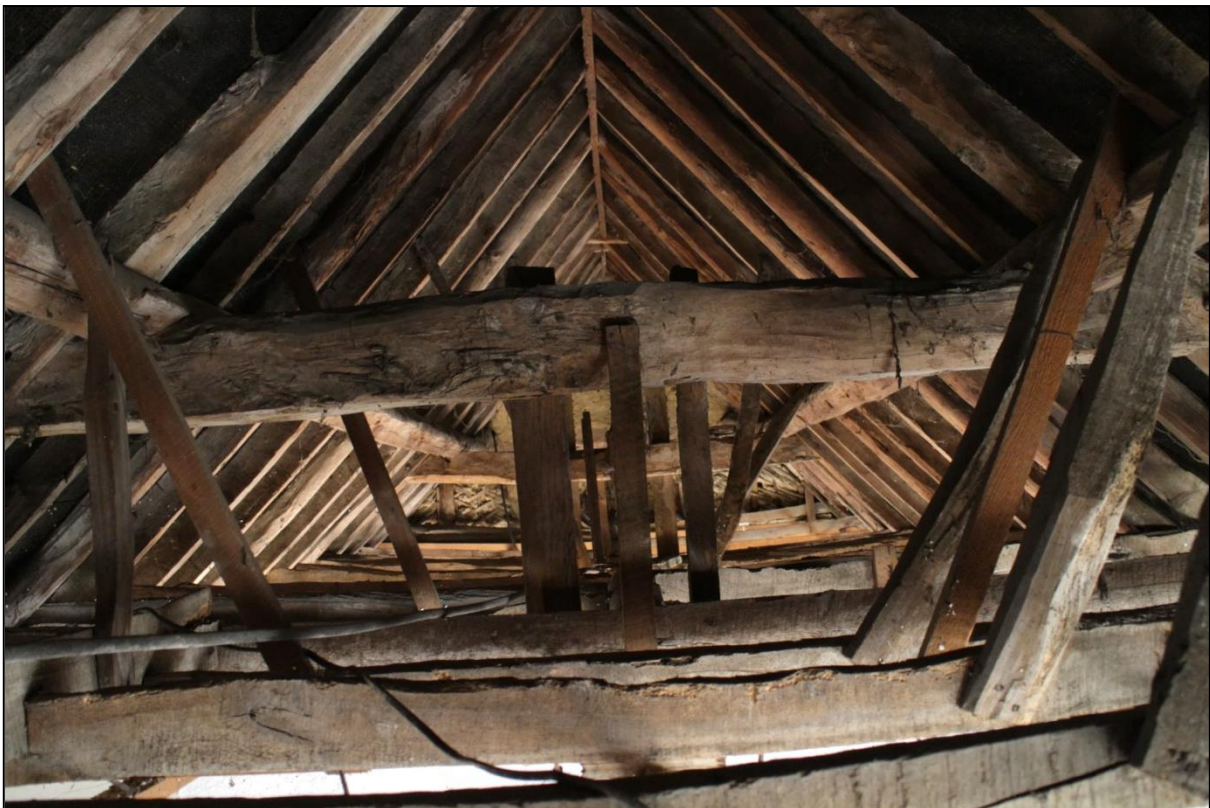
Image 30: Roof over main range, looking south-west
