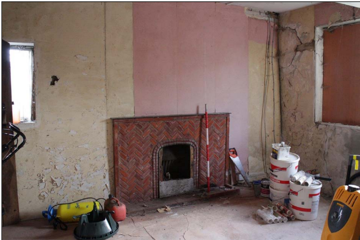
Image 15: Room G2, looking south-west Shows 20th century brick fireplace (Scale 1m)
