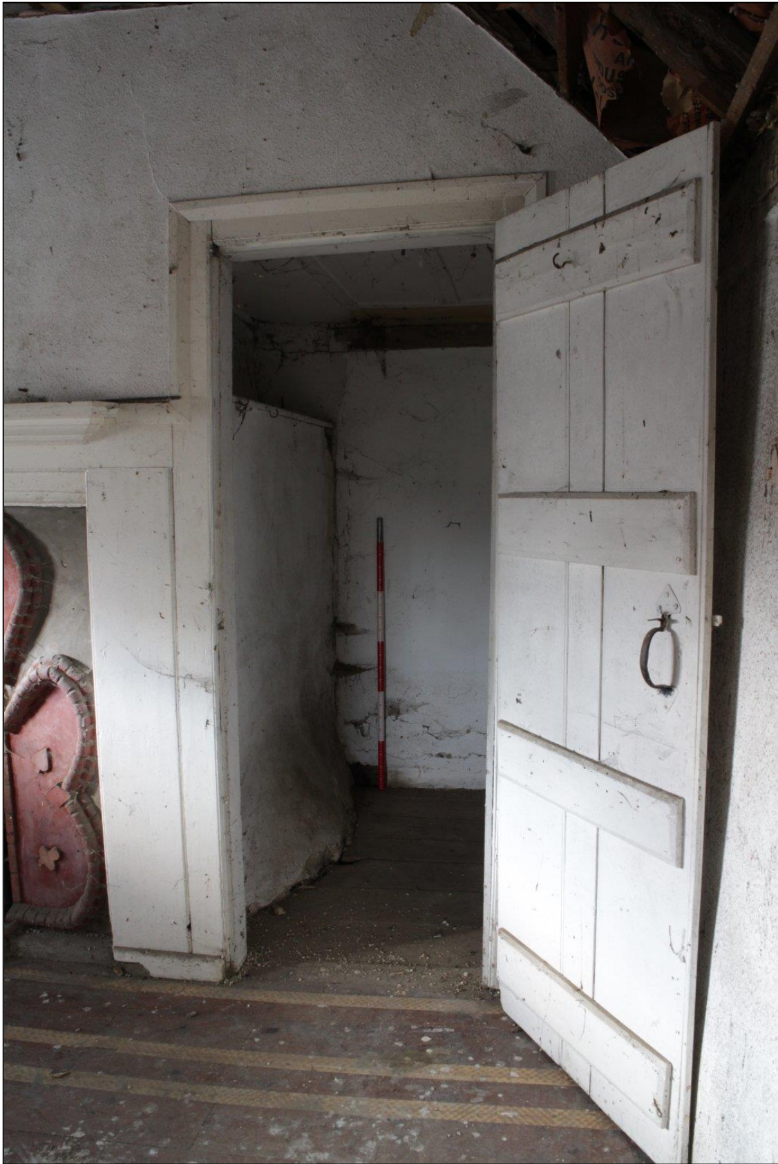
Image 20: Room F1, detail of closet next to the fireplace Shows side of chimney with expanded lower section (Scale 1m)
