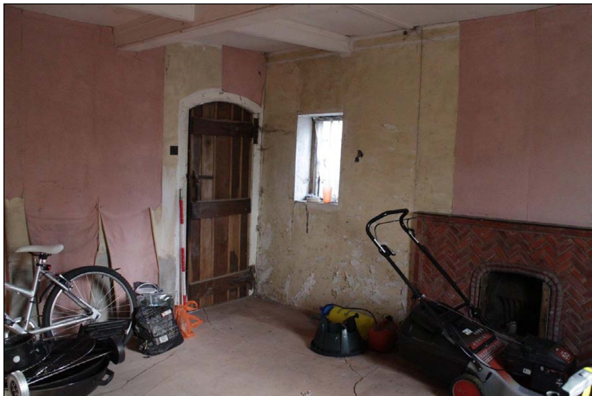
Image 14: Room G2, looking south
