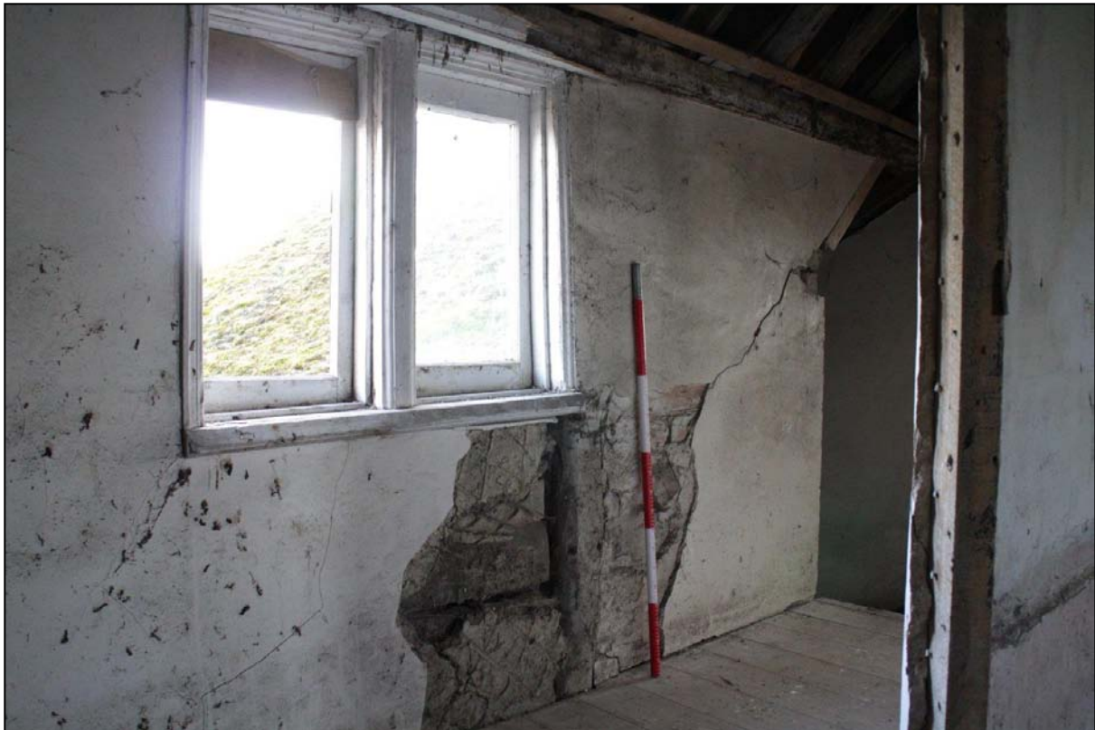
Image 44: Room F, looking west
