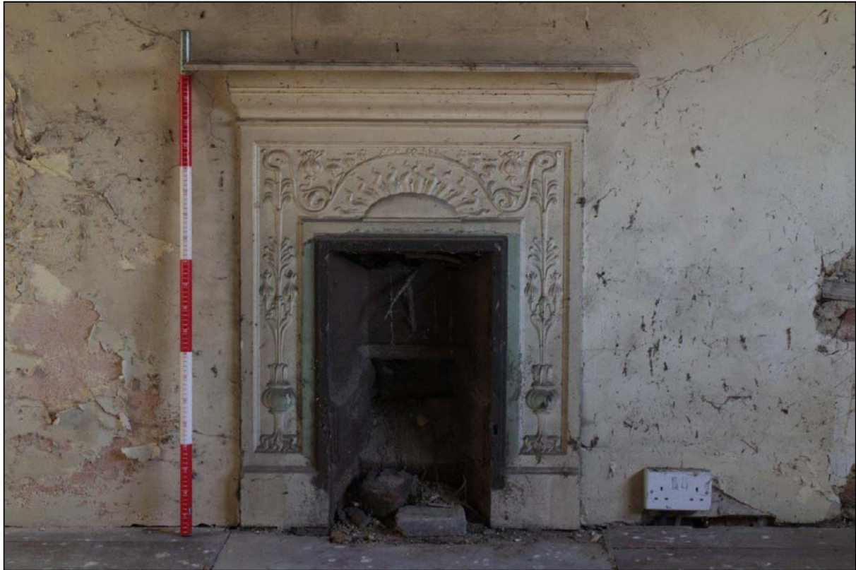
Image 25: Room F2, detail of fireplace
