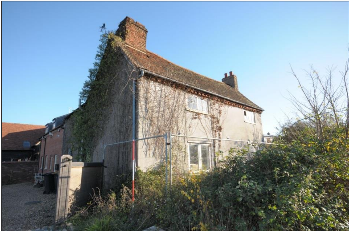
Image 3: View of building looking south
