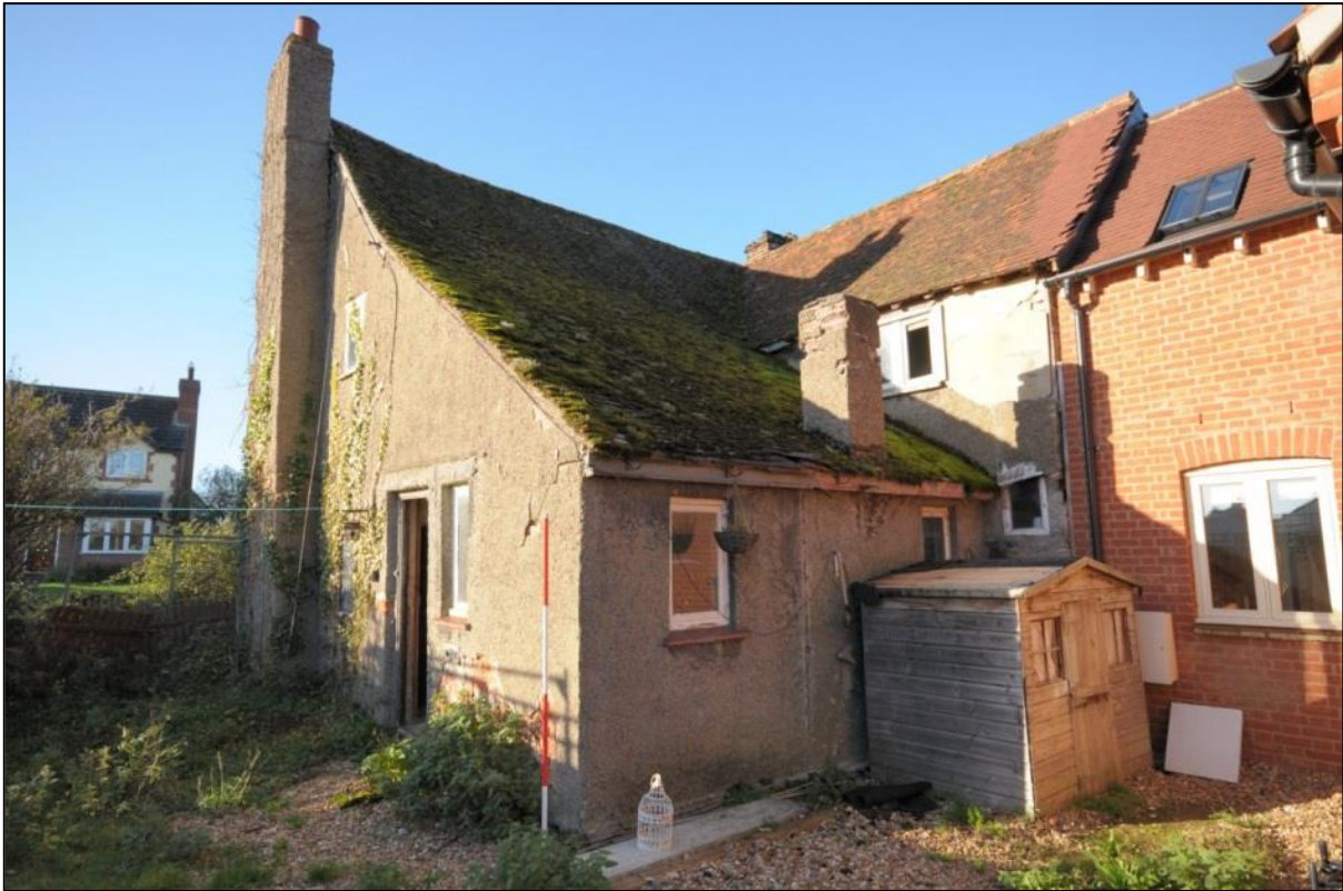
Image 7: View of rear of building, looking north
