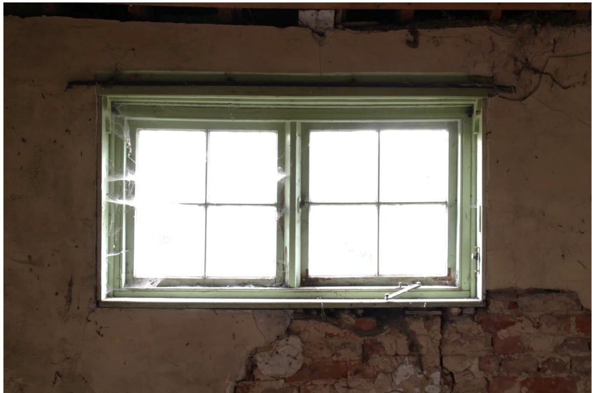
Image 26: Room F2, detail of window in north-west wall
