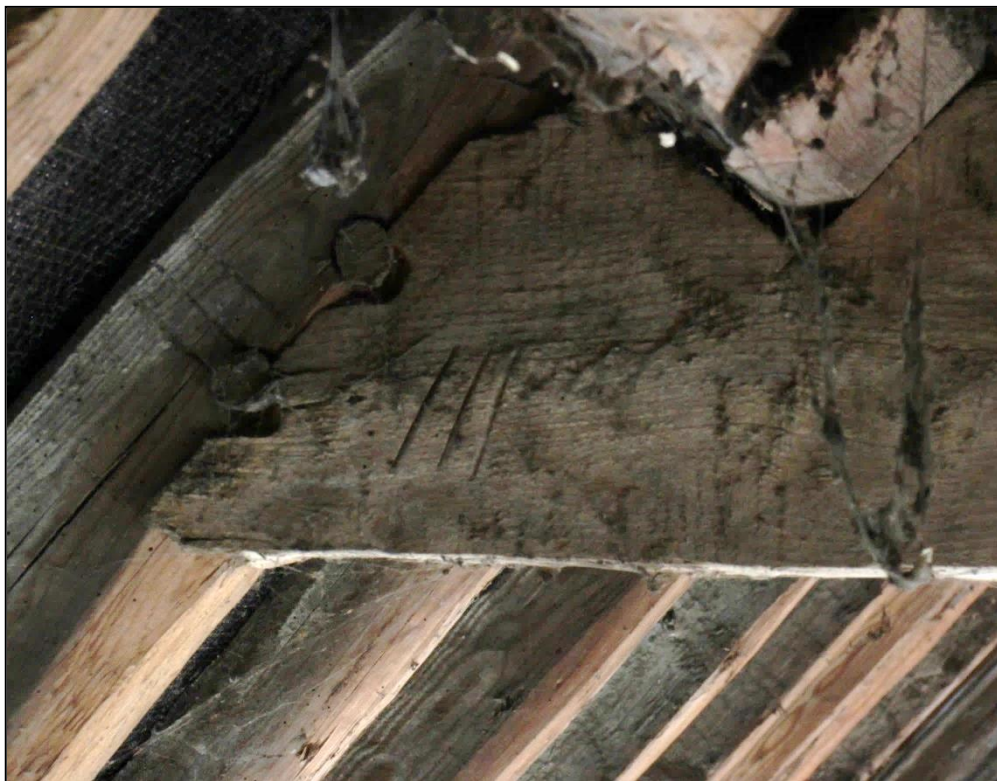
Image 32: Roof, detail of assembly marks
