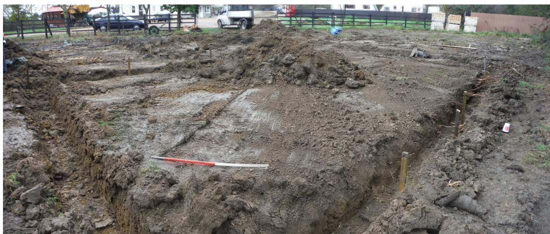
Plate 1: Photo montage of the foundation trenches, looking north-east
