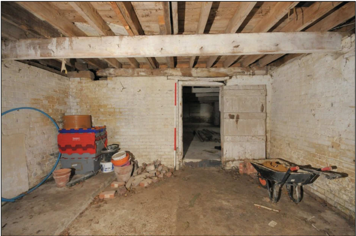
Image 13: Barn 1 interior, southern compartment, looking north-east Shows plank and batten door to main compartment (Scale 2m)
