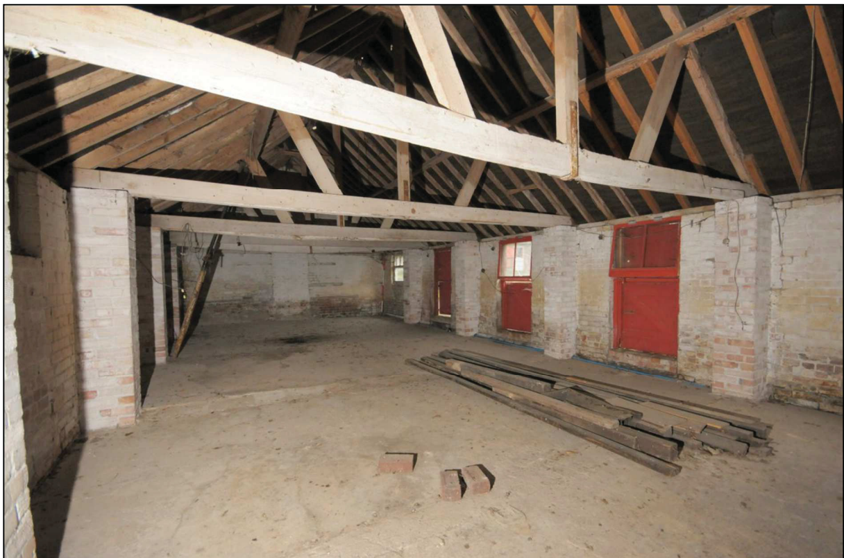
Image 8: Barn 1 interior, main compartment, looking north-east Shows inserted brick piers below the ends of the tie beams
