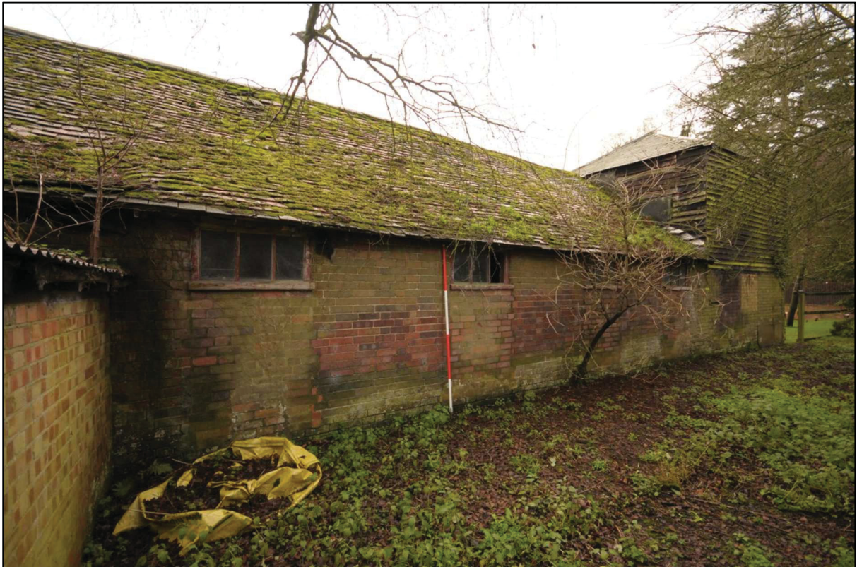
Image 7: Barn 1, north-west (rear) elevation, looking south Shows blocked door openings with inserted windows in rear wall
