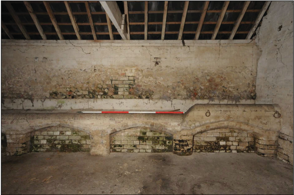
Image 35: Barn 3 interior, north-west compartment, southern end of trough Shows brick trough with raised section with tether rings (Scale 2m)
