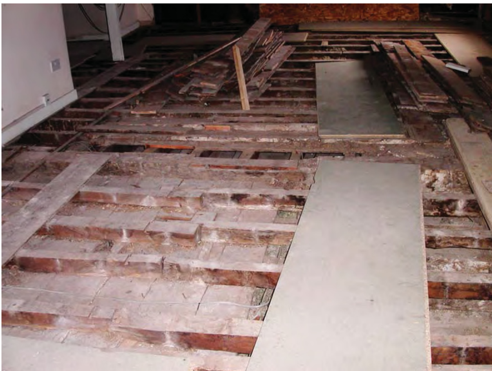
Plate 26: Attic floor, showing earlier floorboards preserved beneath later floor level
