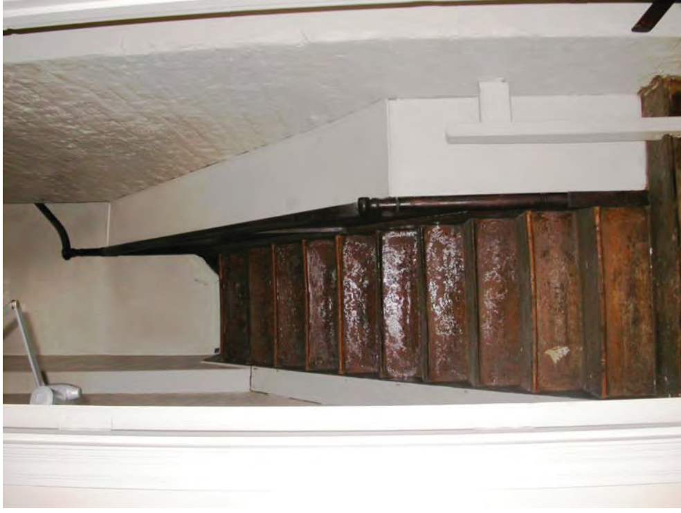
Plate 11: First floor, secondary stairs, looking up from the first floor landing
