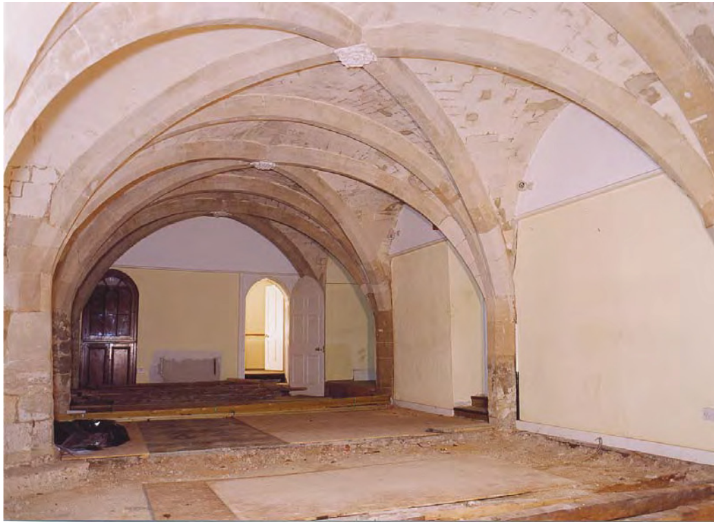
Plate 5: Ground floor, Room G1 looking towards the western end
