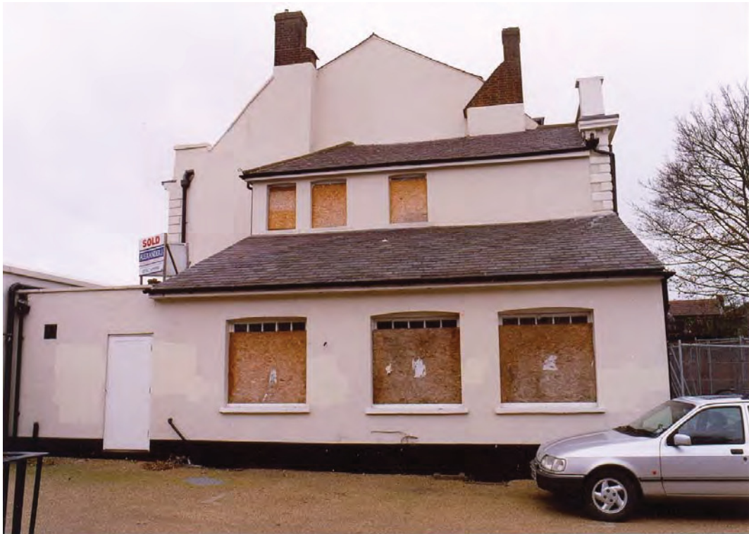
Plate 3: Exterior, east facing elevation
