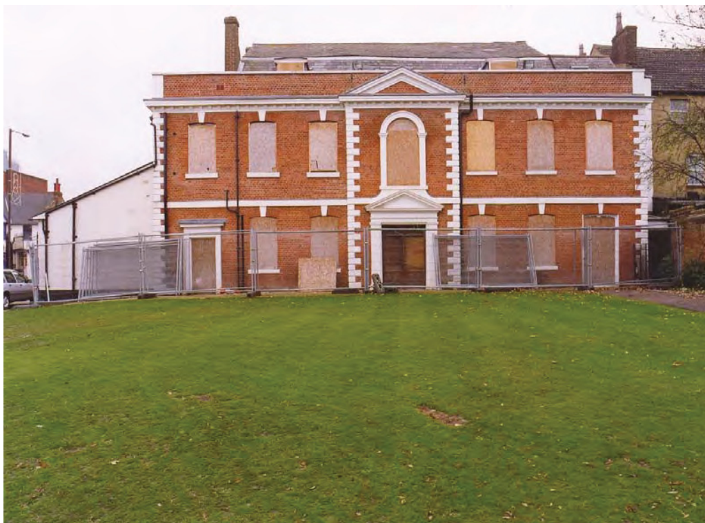
Plate 2: Exterior, north facing elevation
