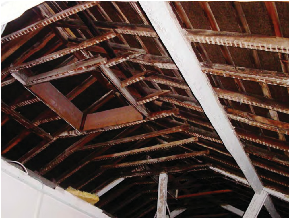
Plate 25: Attic floor, roof structure, showing framing of former ventilator
