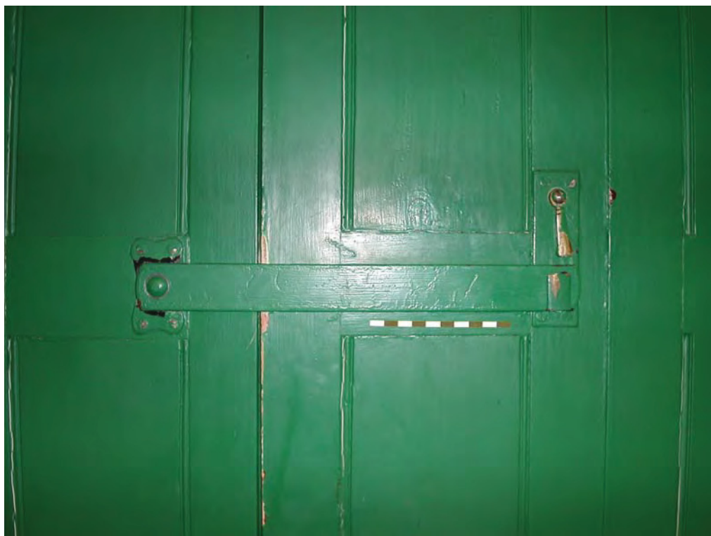
Plate 20: Shutter closure (scale 10cm)
