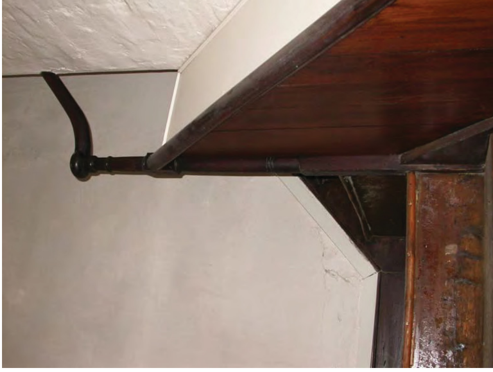
Plate 12: First floor, secondary stairs
