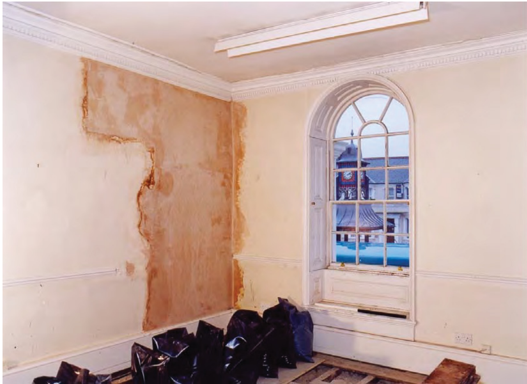
Plate 21: First floor, Room F6, southeast corner
