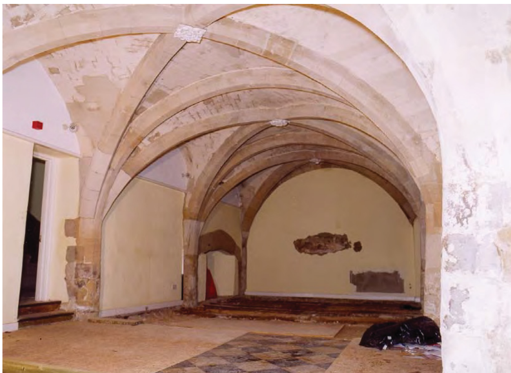
Plate 4: Ground floor, Room G1 looking towards the eastern end
