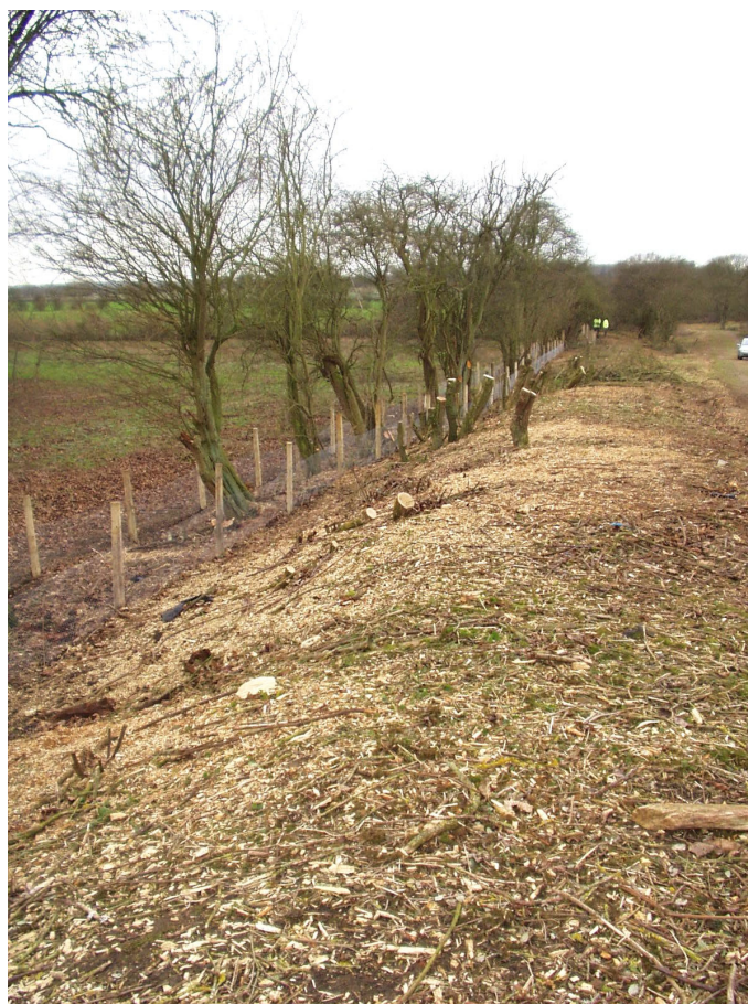
Photograph 1: Western side of embankment near modern ramp (looking north-west).
