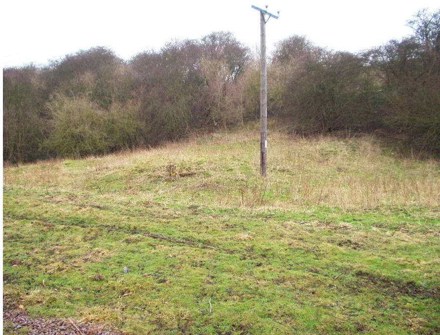
Photograph 2: Main debris tail (D) sloping down western side of embankment.
