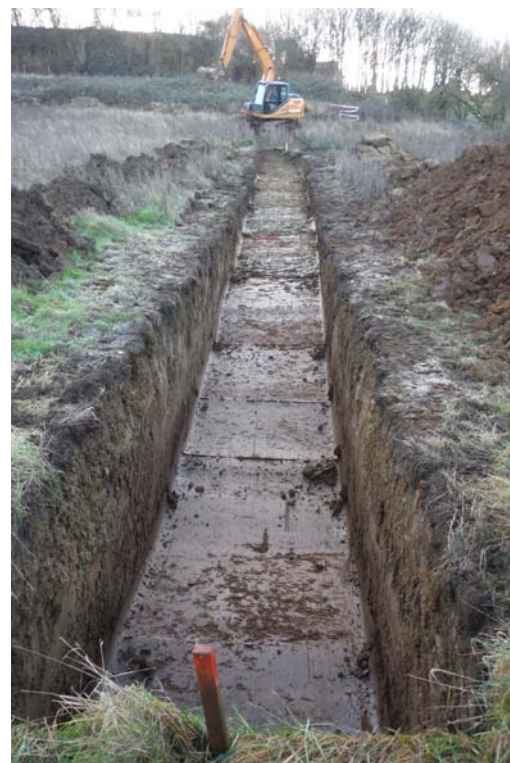
Image 2: Trench 2 – looking SSE.
