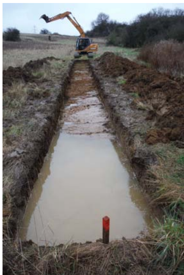
Image 1: Trench 8 – looking NE; flooded ditches [807] and [809] in foreground
