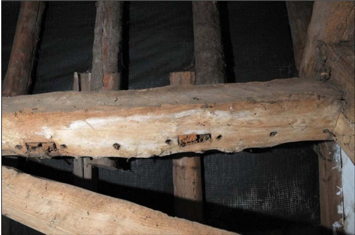
Image 7: Barn interior, underside of wall plate in east side of Bay 2
