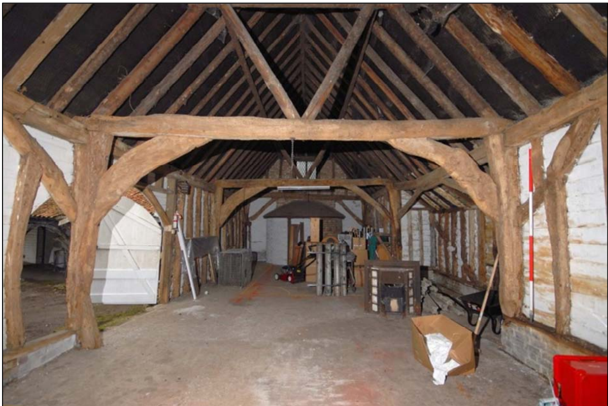
Image 6: Barn interior, looking north from Bay 3
