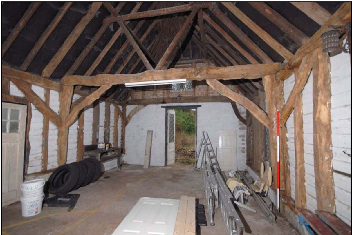
Image 4: Barn interior, looking south from Bay 3
