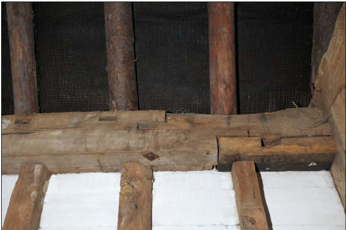
Image 12: Barn interior, repaired wall plate in west wall
