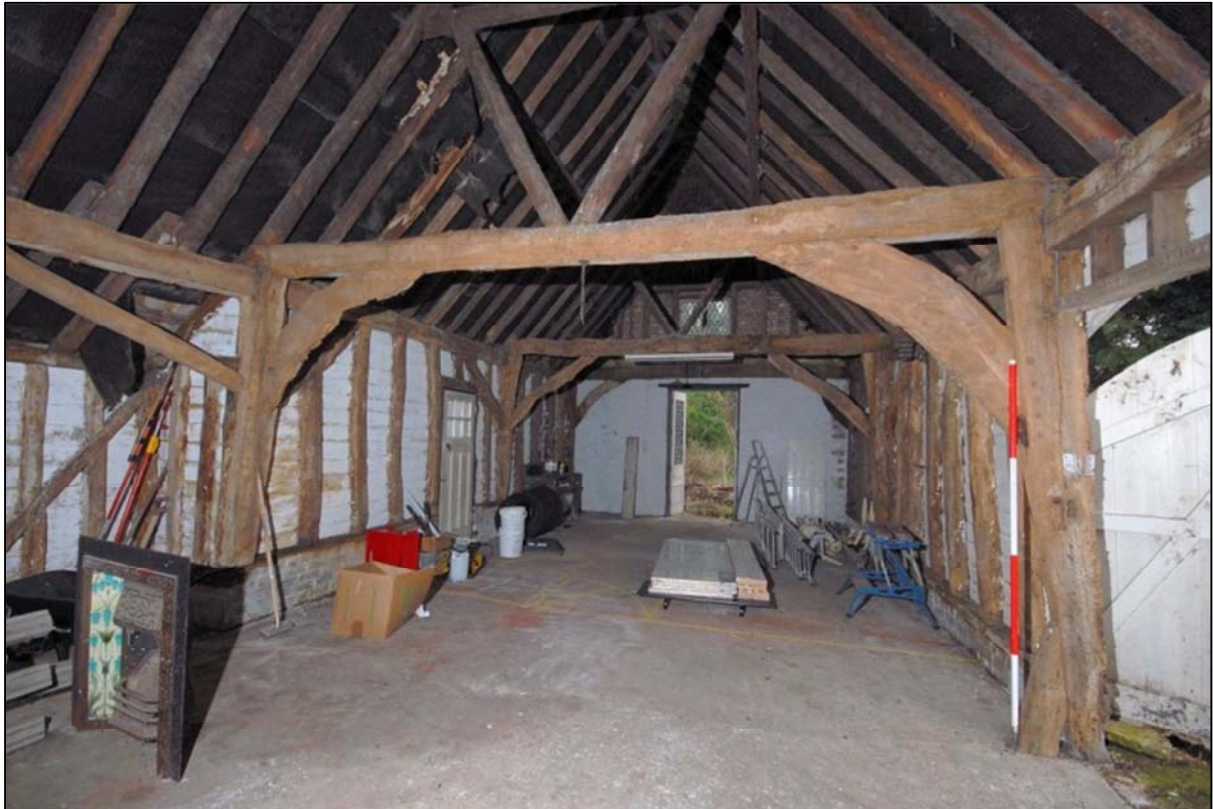
Image 3: Barn interior, looking south from Bay 2
