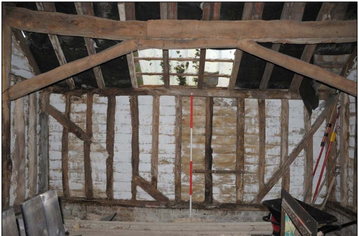
Image 10: Barn interior, extension on east side of Bay 2
