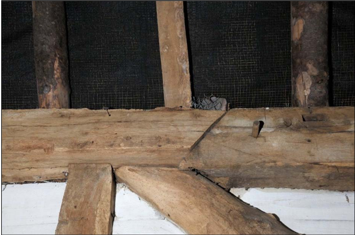
Image 11: Barn interior, repaired wall plate in west wall
