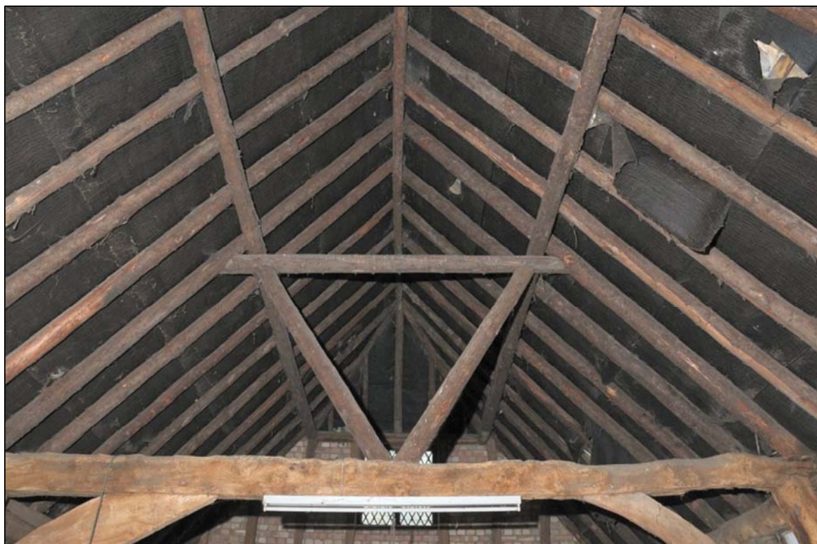
Image 14: Barn interior, roof structure
