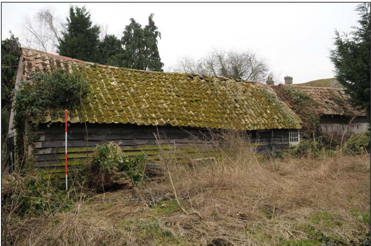
Image 16: Stables, north elevation, looking south-west
