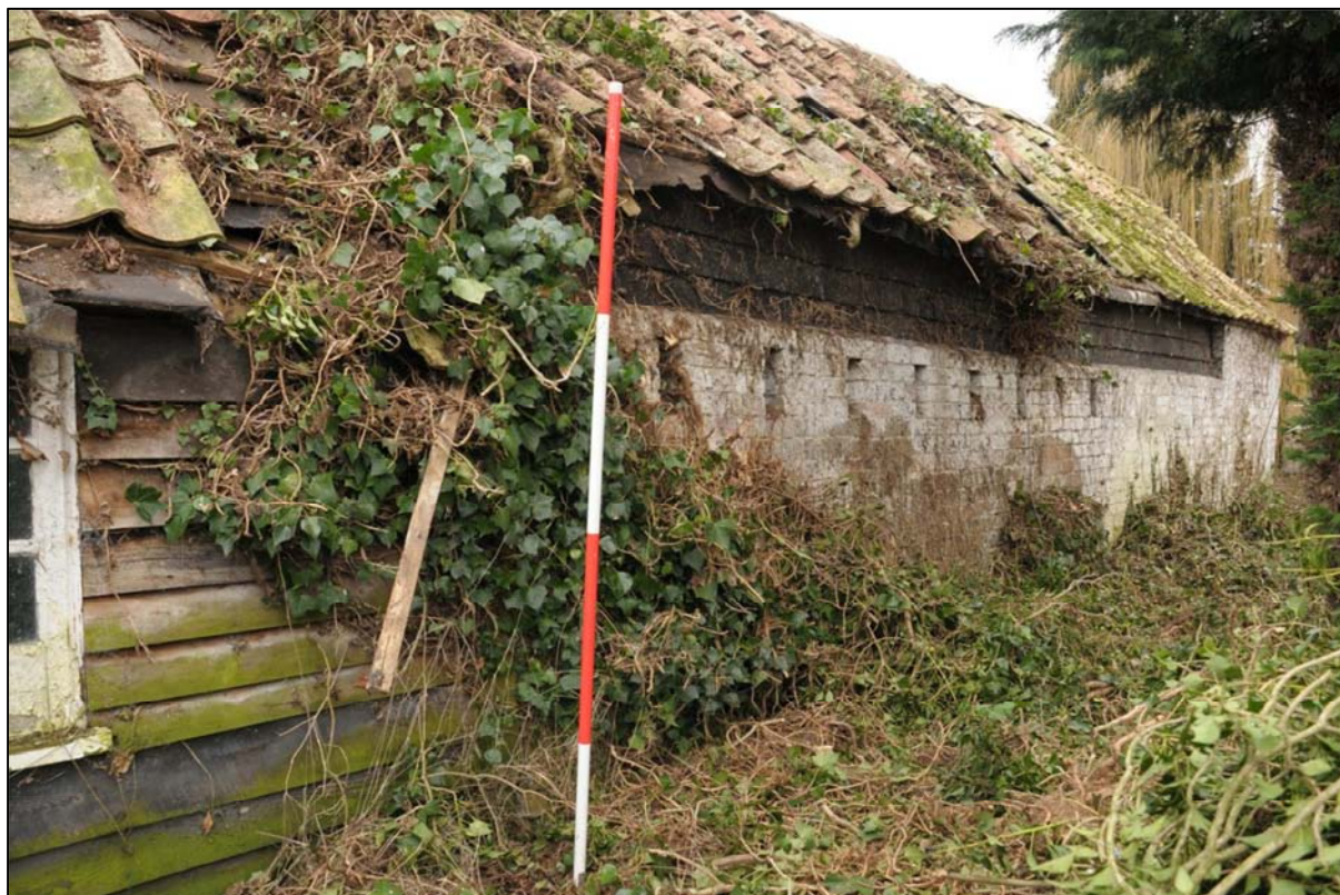
Image 17: Stables, north elevation, looking south-west
