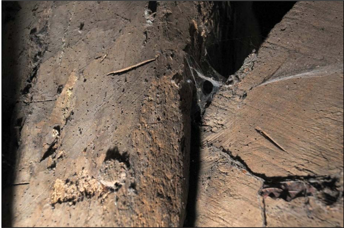
Image 9: Barn interior, assembly marks
