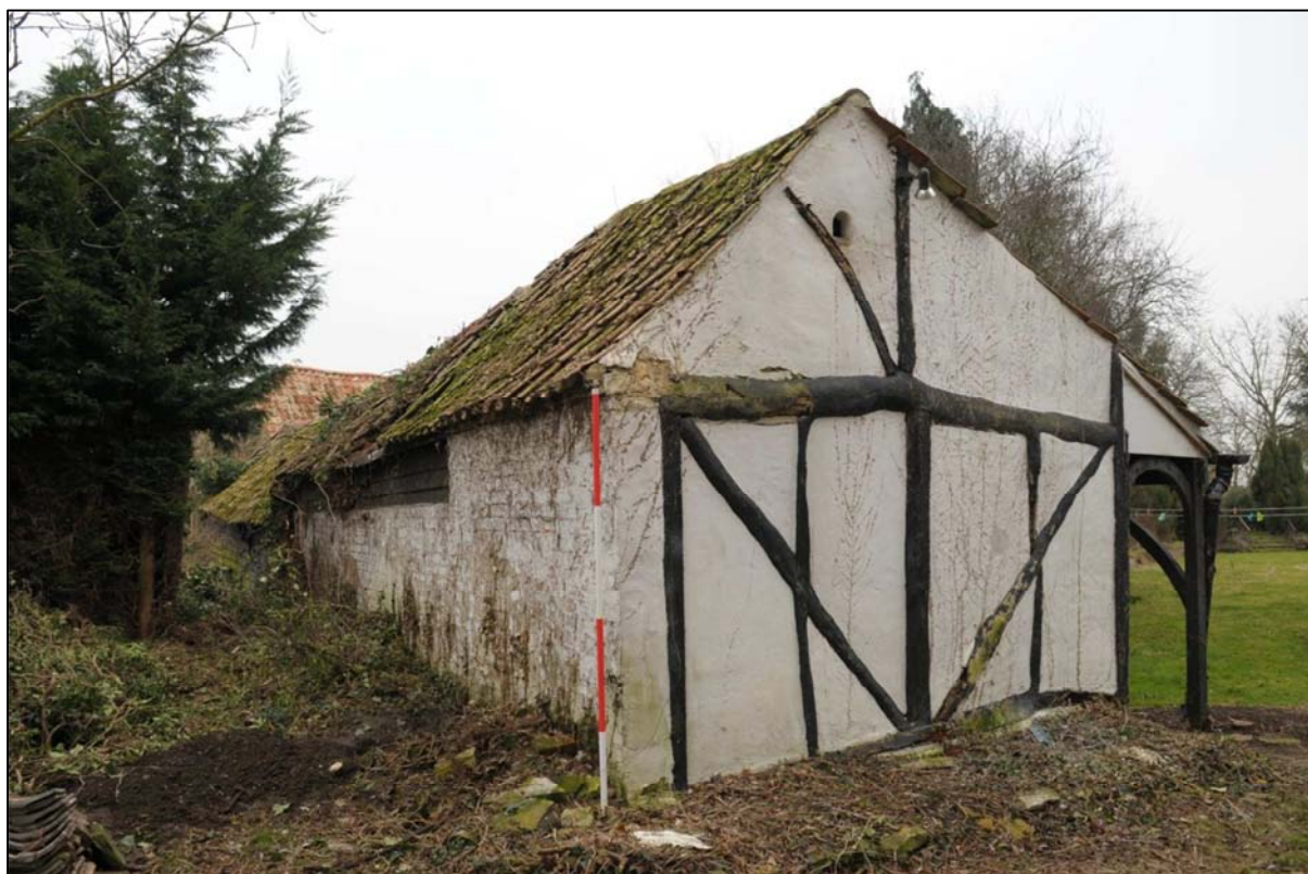
Image 18: Stables, west end wall, looking south-east
