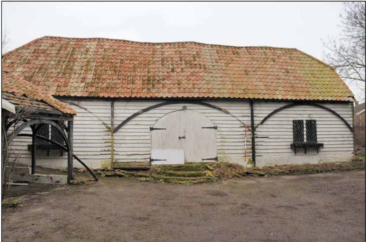
Image 1: Barn, west elevation
