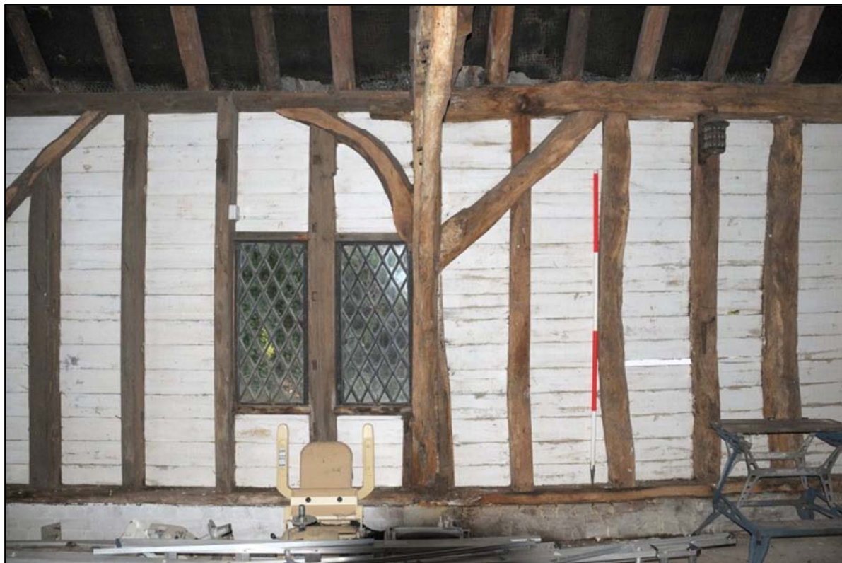
Image 13: Barn interior, west wall at Frame 4
