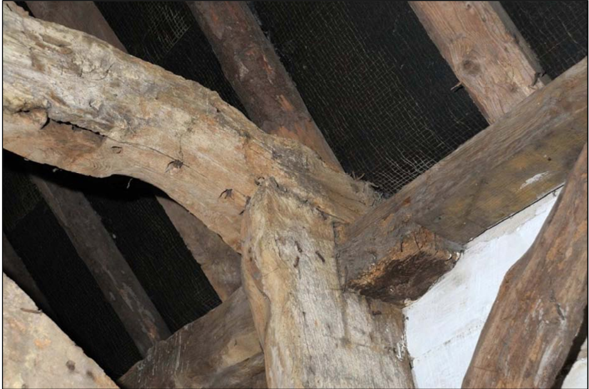
Image 8: Barn interior, south side of Frame 4, east wall
