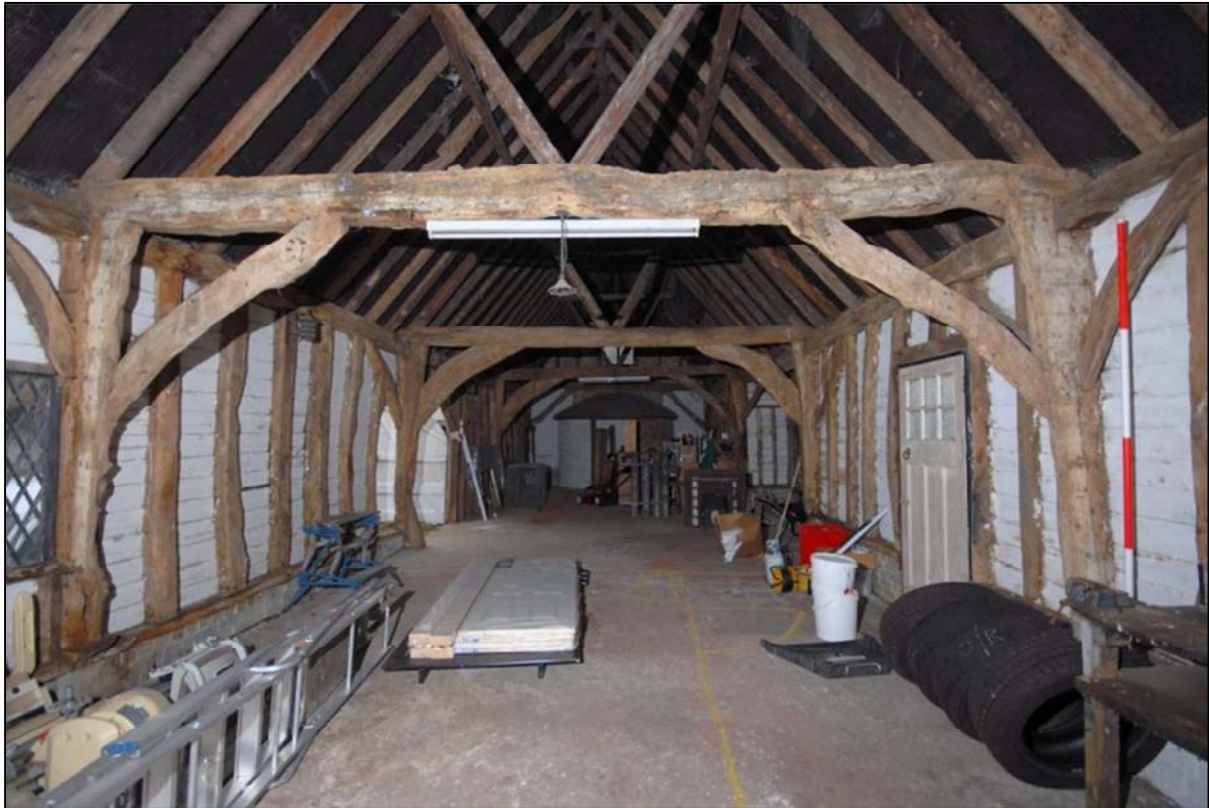
Image 5: Barn interior, looking north from Bay 4
