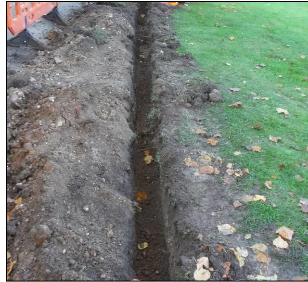
Example trench through churchyard south-west of Z004, looking south-west (1m scale)
