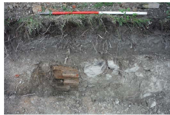
Tr 3. Foundation [308] & (314). Scale 1m. Looking NW.
