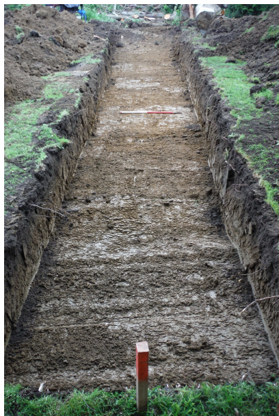
Image 1: View of Trench 3 – pre-excavation; looking NE. Scale 1m
