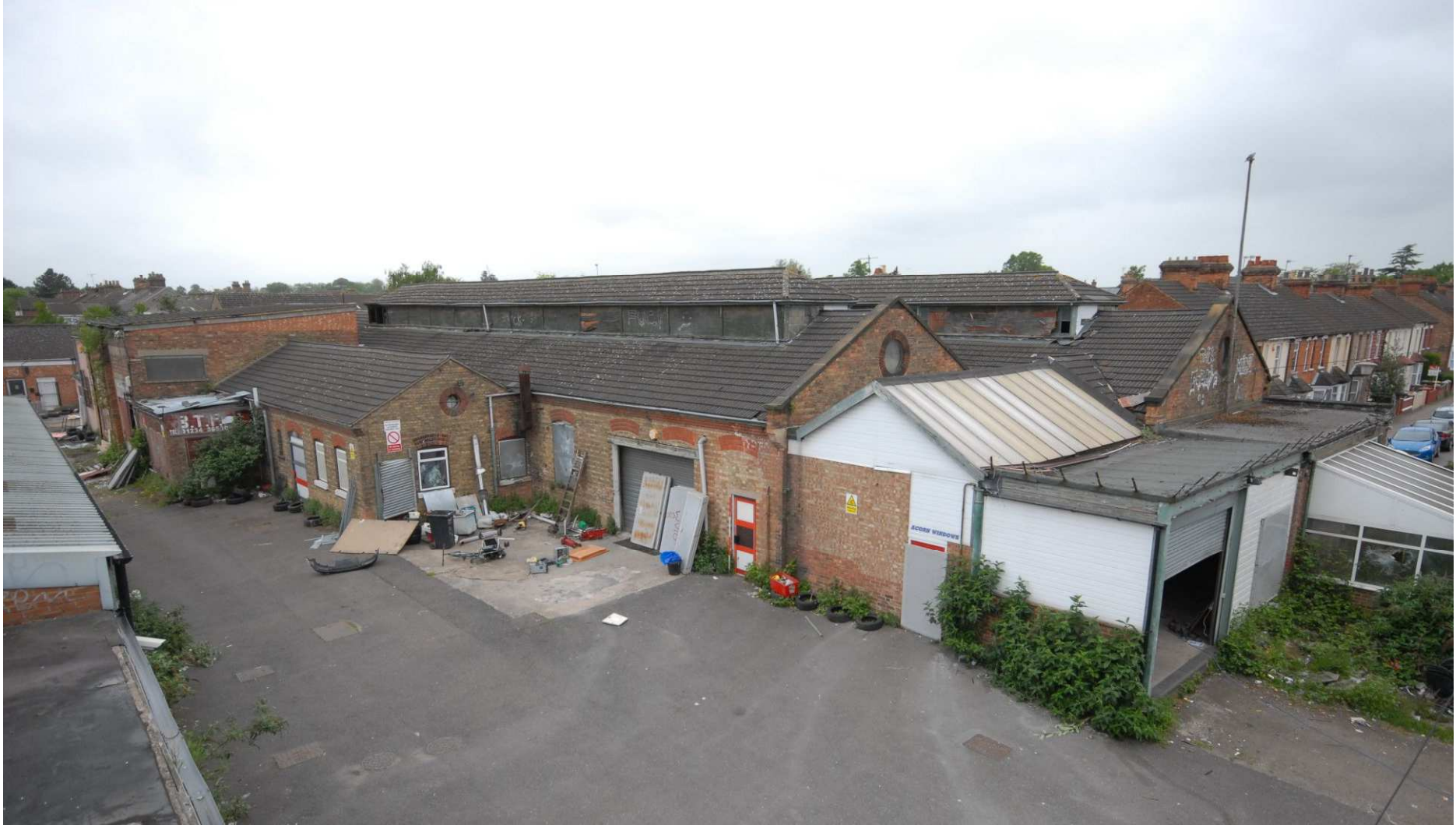
Figure 8: Bedford Sanitary Laundry eastern side, looking SW from footbridge across railway
