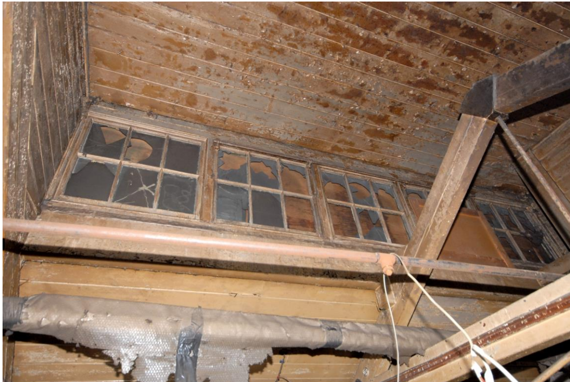
Figure 18: Interior photograph of roof clerestory windows in drying closets room
