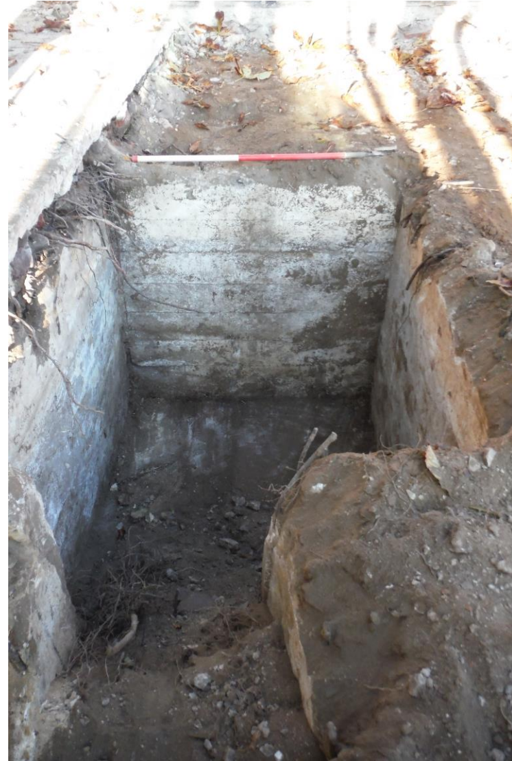
Figure 6: Air-raid shelter, looking south-east
