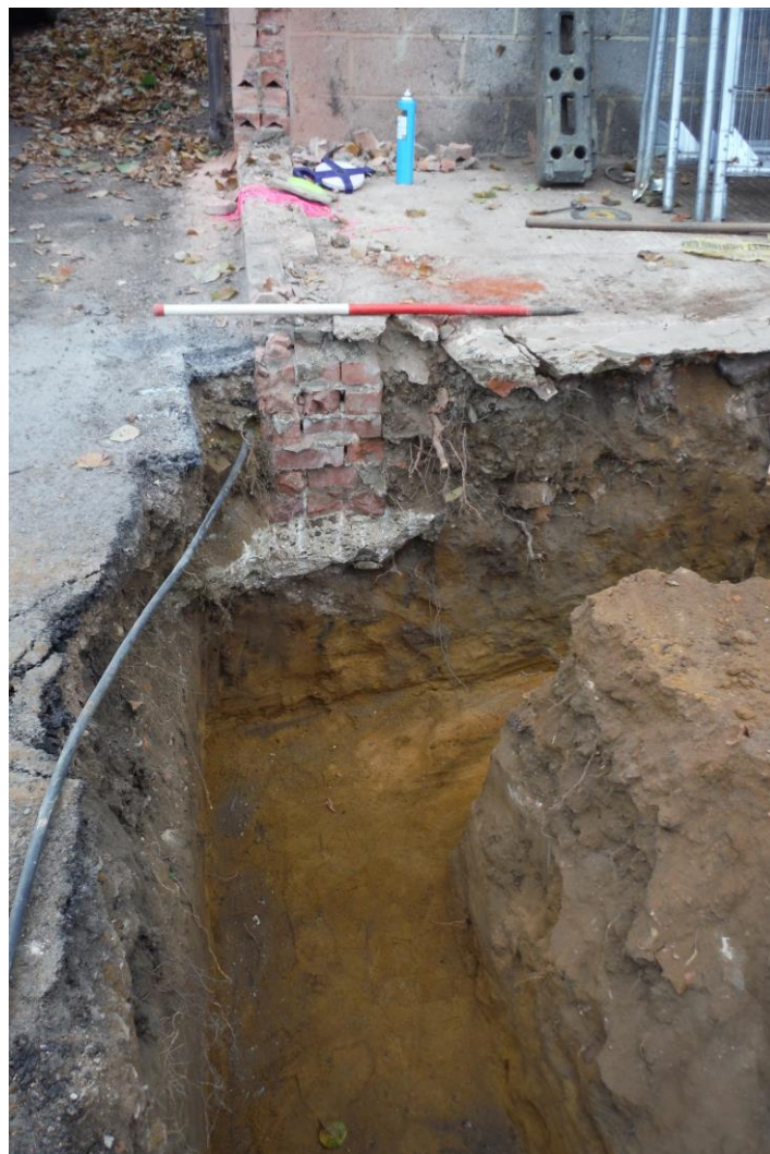
Figure 7: Wall foundation, looking north-east
