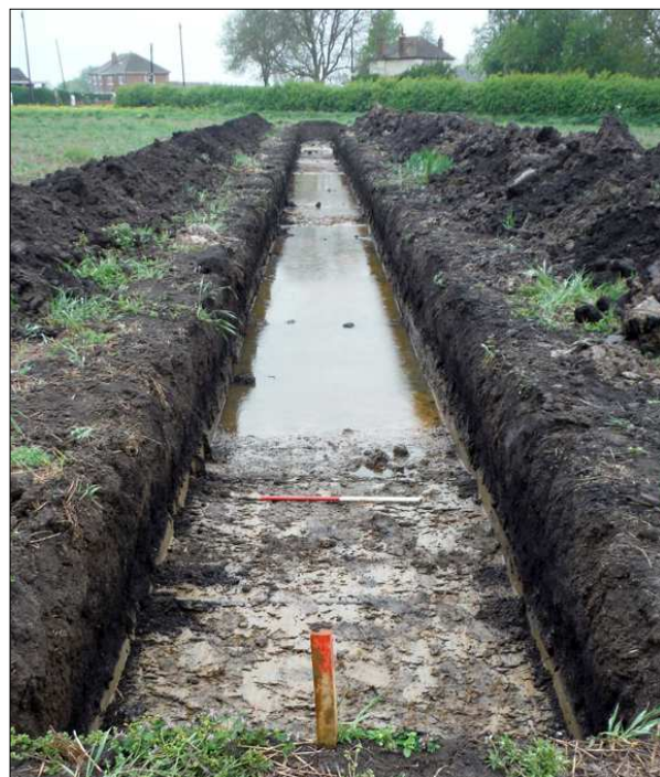
Photograph 5: Trench 4, looking south-west. Scale 1m
