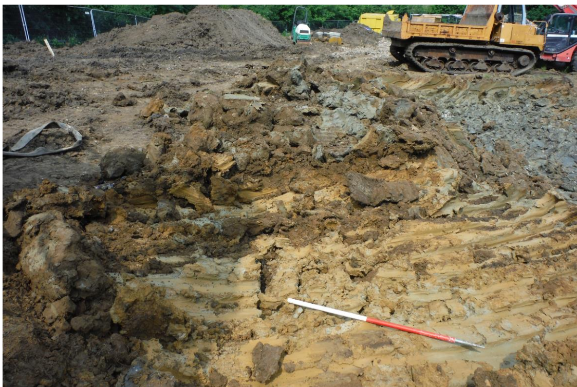
Image 3: Machining reveals a clean area of undisturbed geological strata at a shallow depth. Scale 1m in 50cm divisions.
