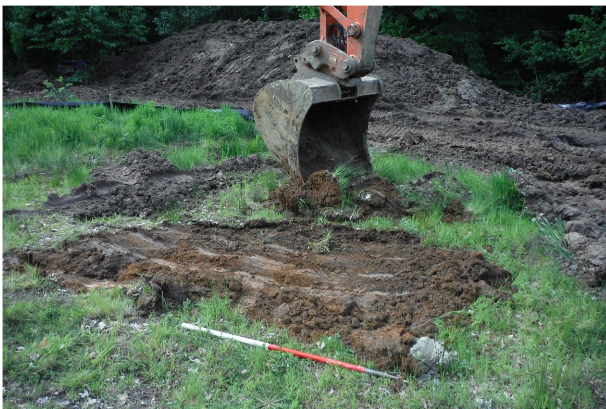
Image 2: Truncated soil profile revealed upslope in area of the building footprint during second visit. The thicker grass seems to define the undisturbed area beyond the building. Scale 1m in 50cm divisions.
